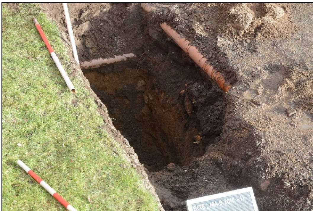
Illus 5: Gully pot trench, looking SE
