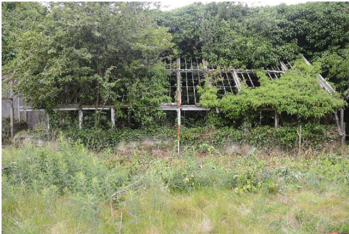
Illus 78 Greenhouse (27) Looking N
