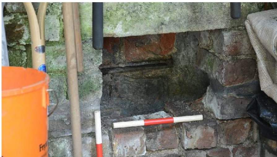
Illus 61 Detail of lower vent in N wall. The grooved metal bar at back may have held a shutter to direct the hot air either sideways or upwards
