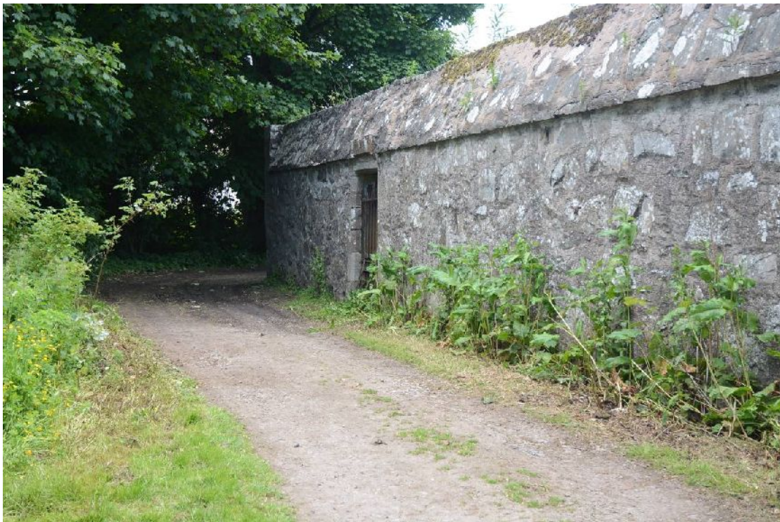
Illus 27 W end of outside of S wall, looking W to SW corner and door 13 (with datestone). Note heavy external batter at top of wall
