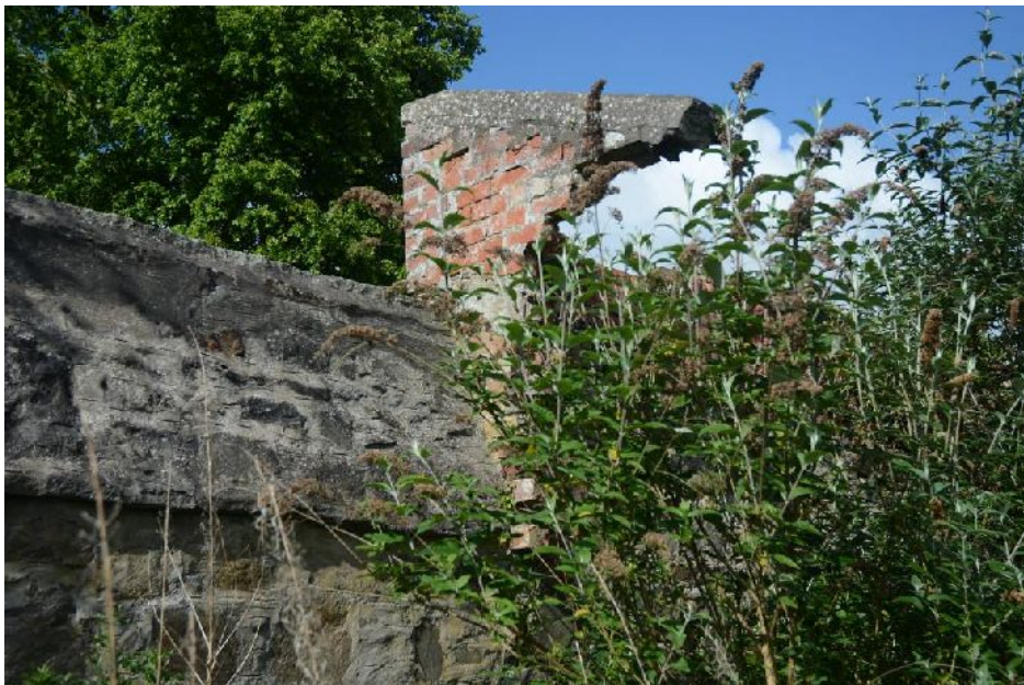
Illus 96 Detail of NW corner of building 24 with garden wall raised to give additional height.
