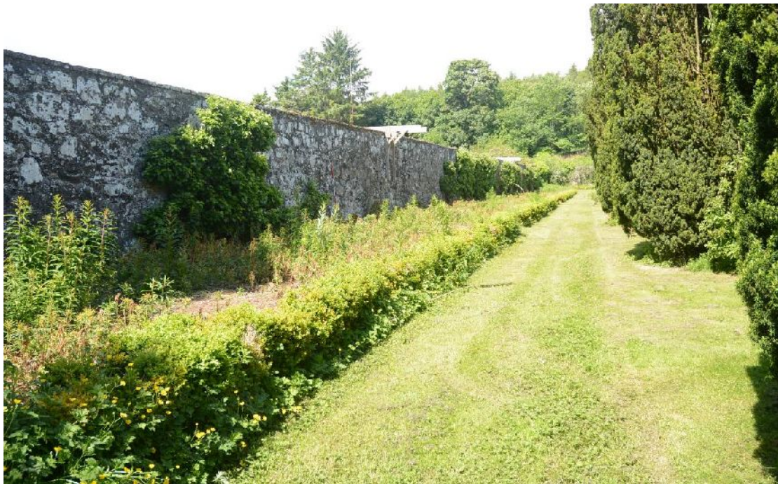
Illus 33 W wall looking N
