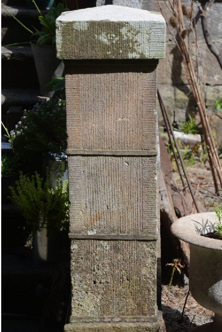
Illus 68 E side of steps. Detail of dressing on stonework of pillar
