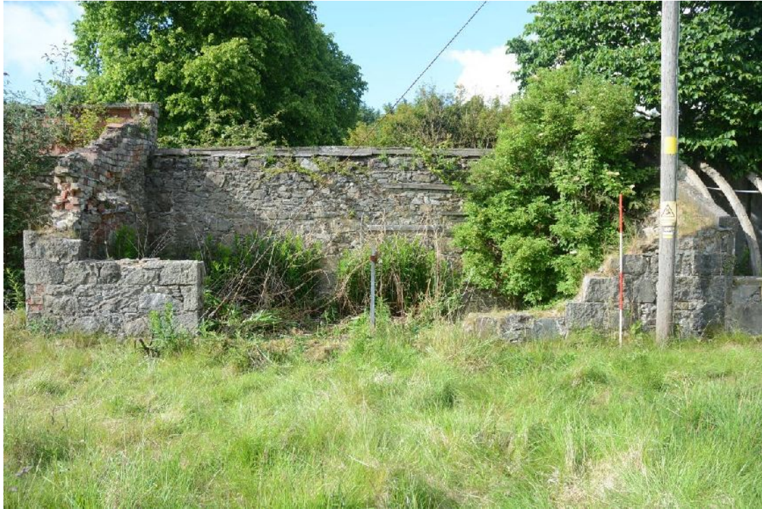
Illus 98 Boiler House 25, general view from S
