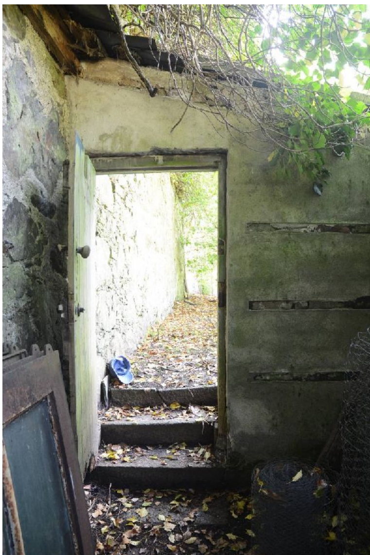
Illus 103 Building 17, inside of W wall showing scars of shelves.
