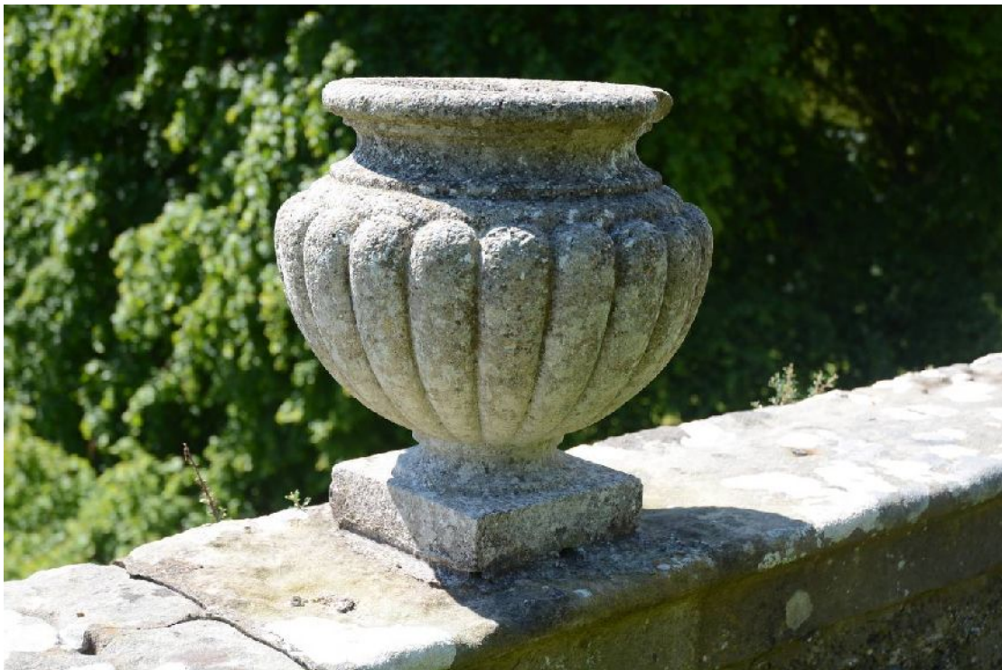
Illus 23 Wall 22. Detail of urn. Railing scars visible on wall top.
