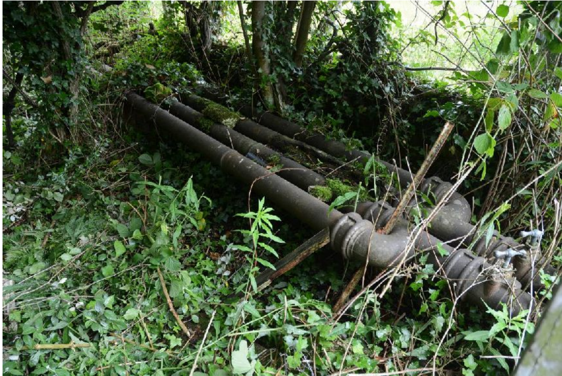
Illus 81 Greenhouse 27 showing water pipes and stopcocks.
