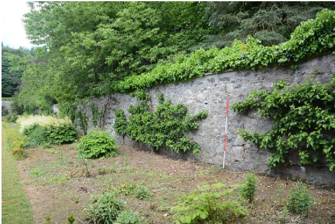
Illus 31 E wall looking N
