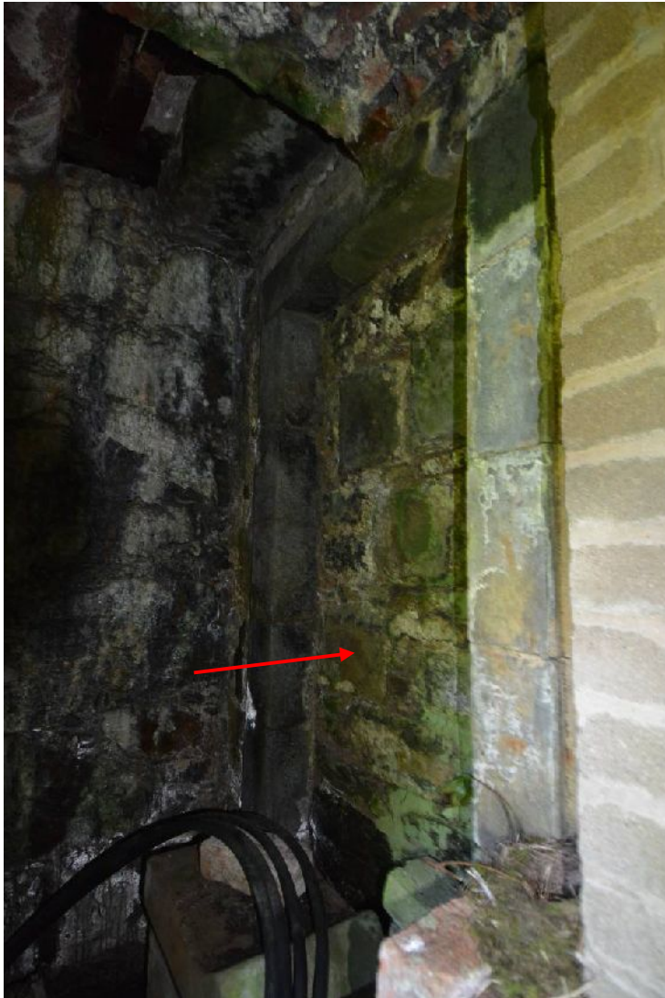
Illus 72 Blocked doorway (D4 marked by red arrow) below steps- this would have opened to ground floor of W end of garden house
