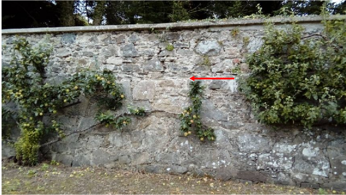
Illus 30 Detail of E wall interior showing change in stonework (red arrow)
