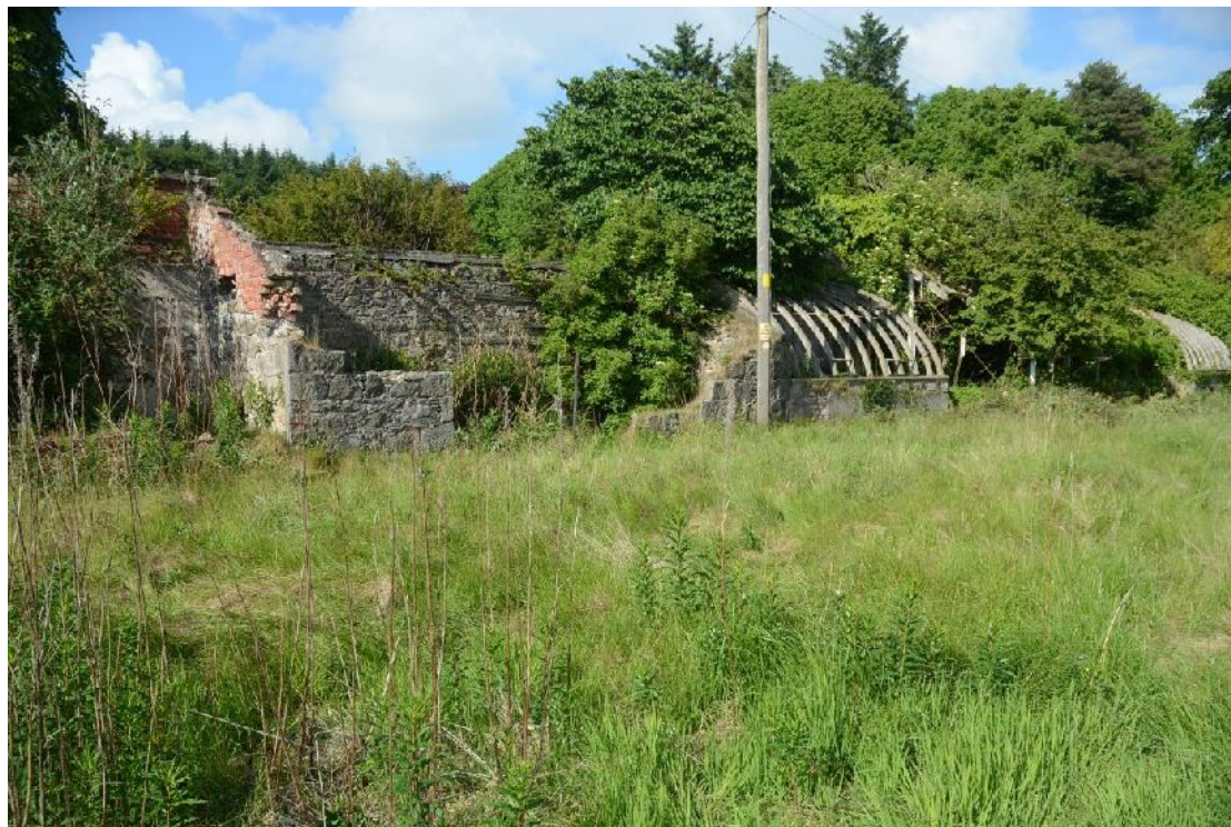
Illus 75 View of greenhouses from L to R: 24,25,26,27,28
