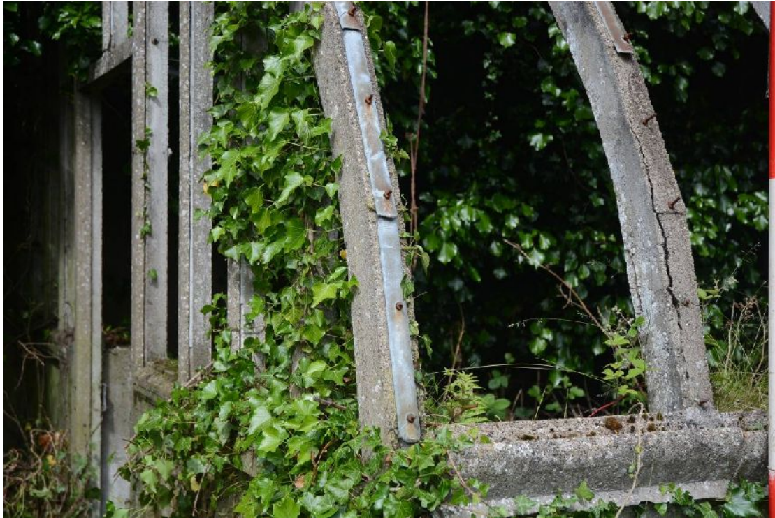
Illus 91 Greenhouse 28, detail of glazing bars and fixings
