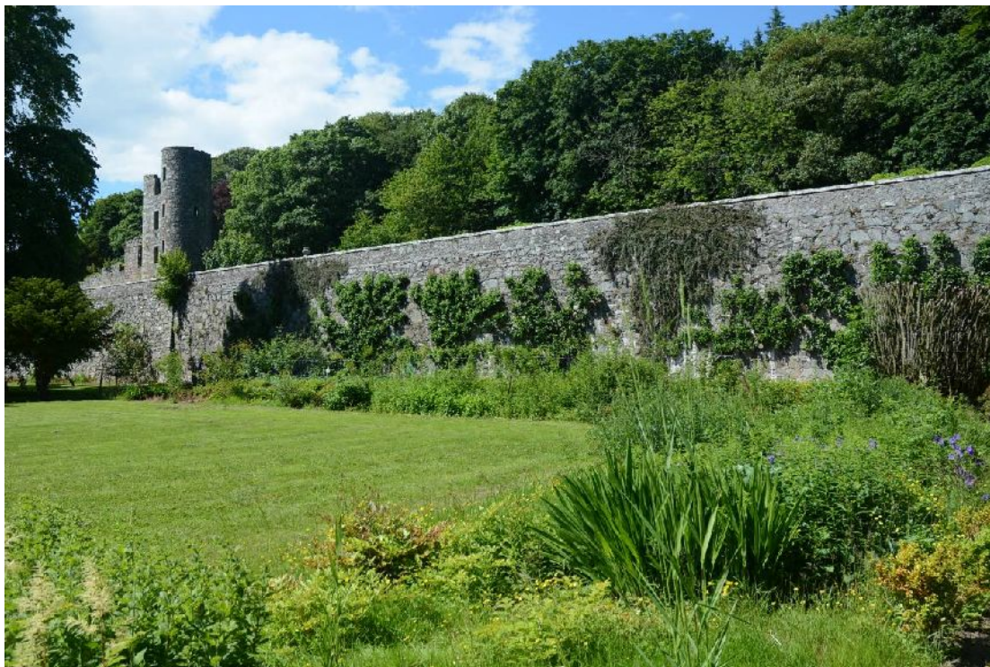
Illus 19 N wall E of Garden House, looking W
