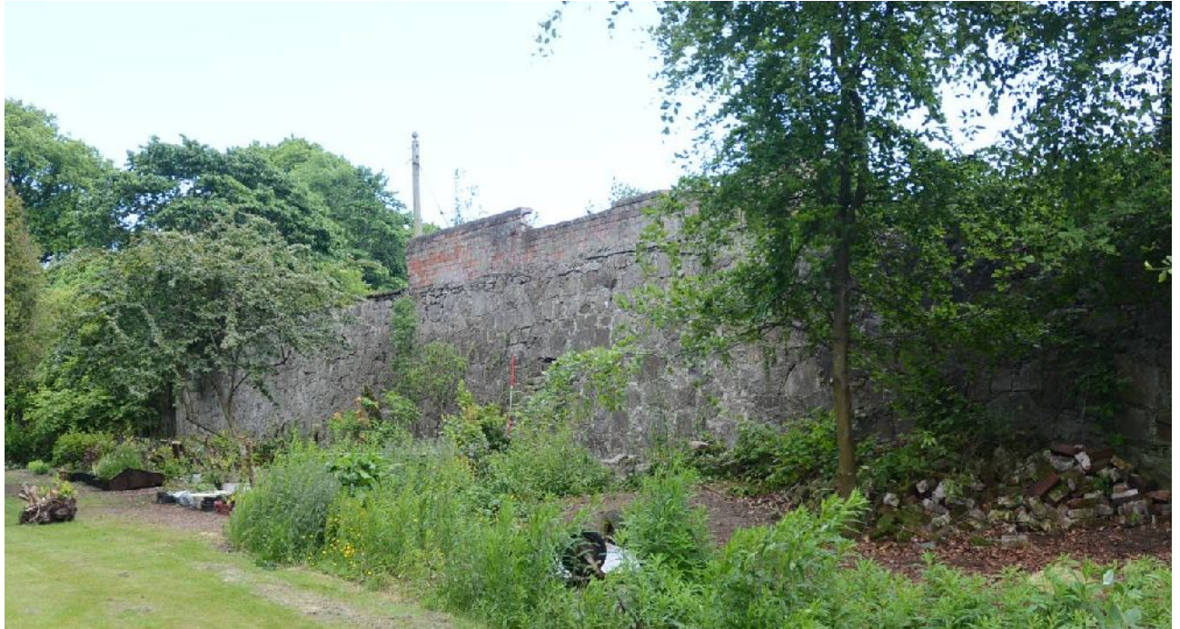
Illus 28 Detail of S wall showing wall top raised for the greenhouses on outside.
