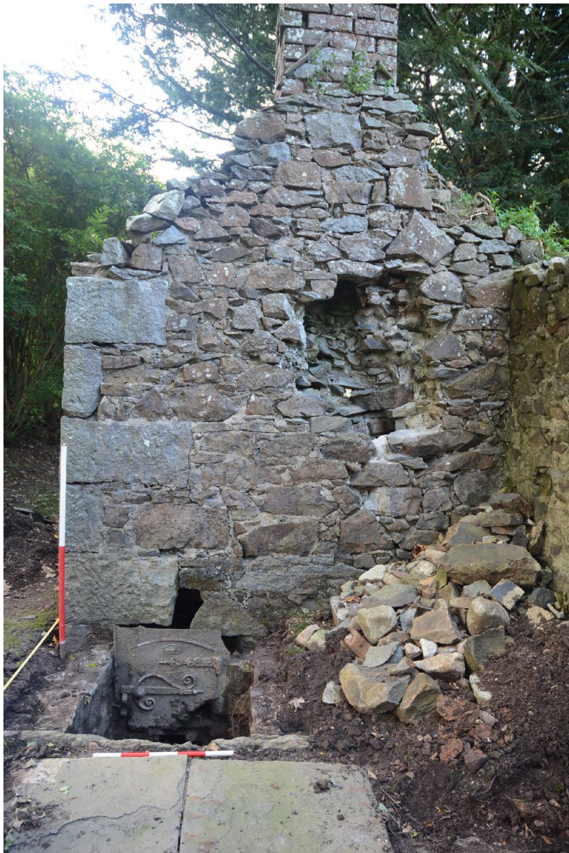
Illus 9 E side of W gable showing stoking pit
