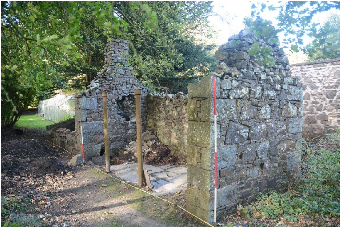
Illus 1 Building 1 from SE. Garden wall visible behind to RHS
