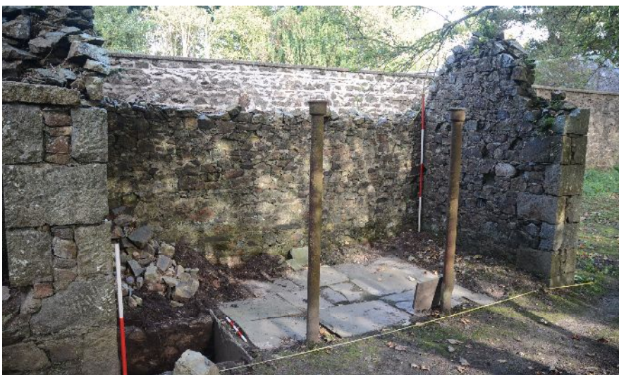
Illus 7 E end of building from S. Garden wall behind
