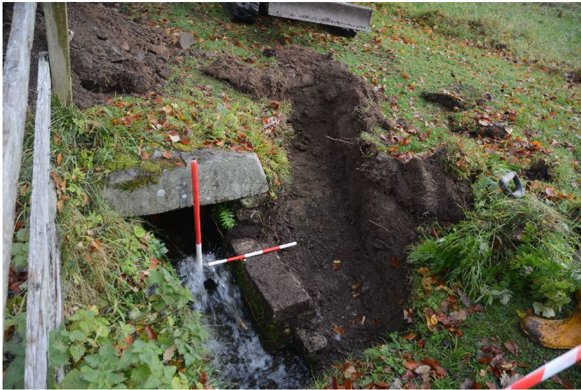
Illus 12 Culvert at W end of drain beside drive
