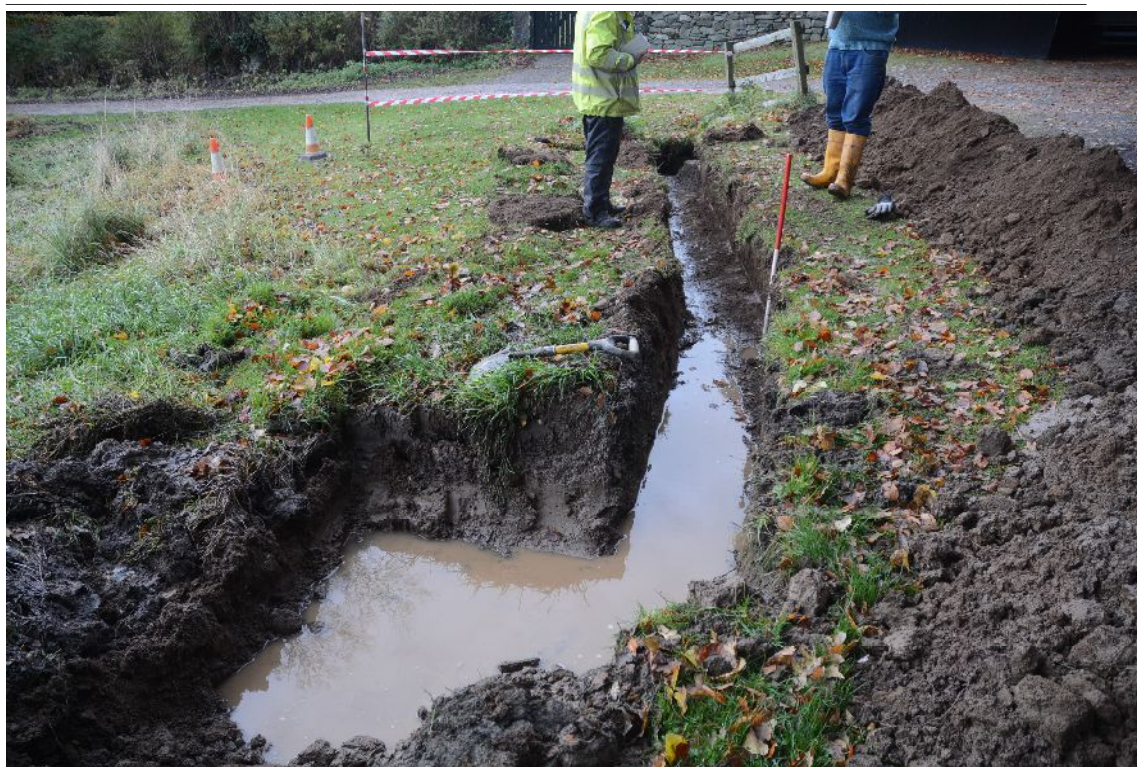
Illus 14 Drain looking W
