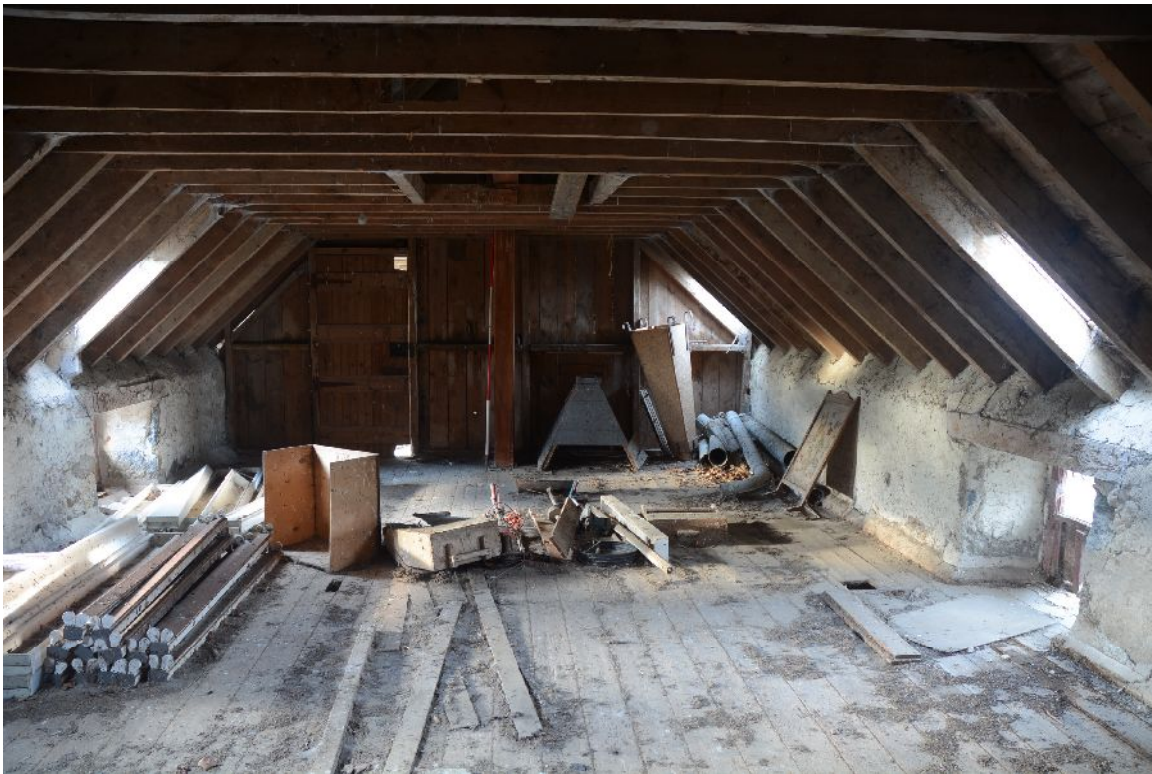
Illus 29 Grain loft (Area M) looking N. Ranging rod beside vertical grain chute
