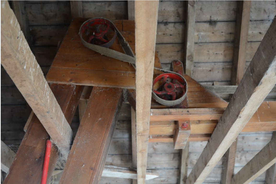
Illus 30 Grain chutes and pulley belts
