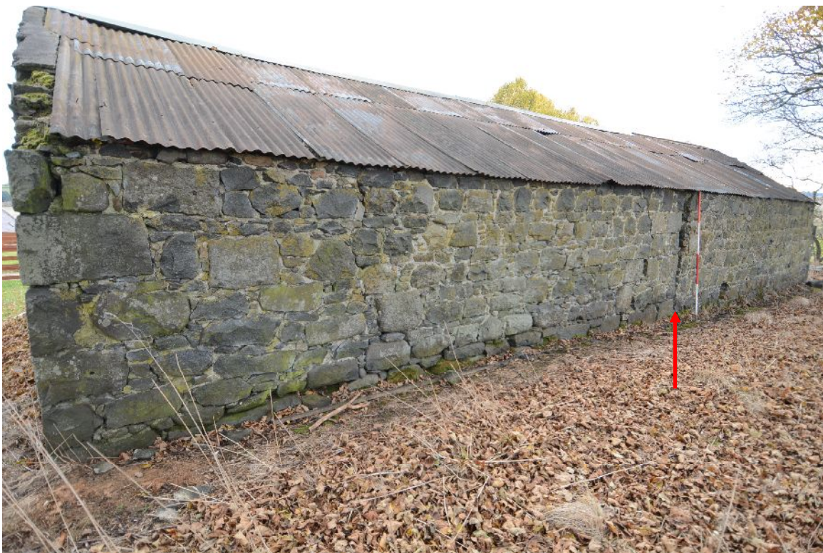
Illus 33 Building 2 from back. Arrow marks raggle which was probably W end of original steading as on 1871 OS map
