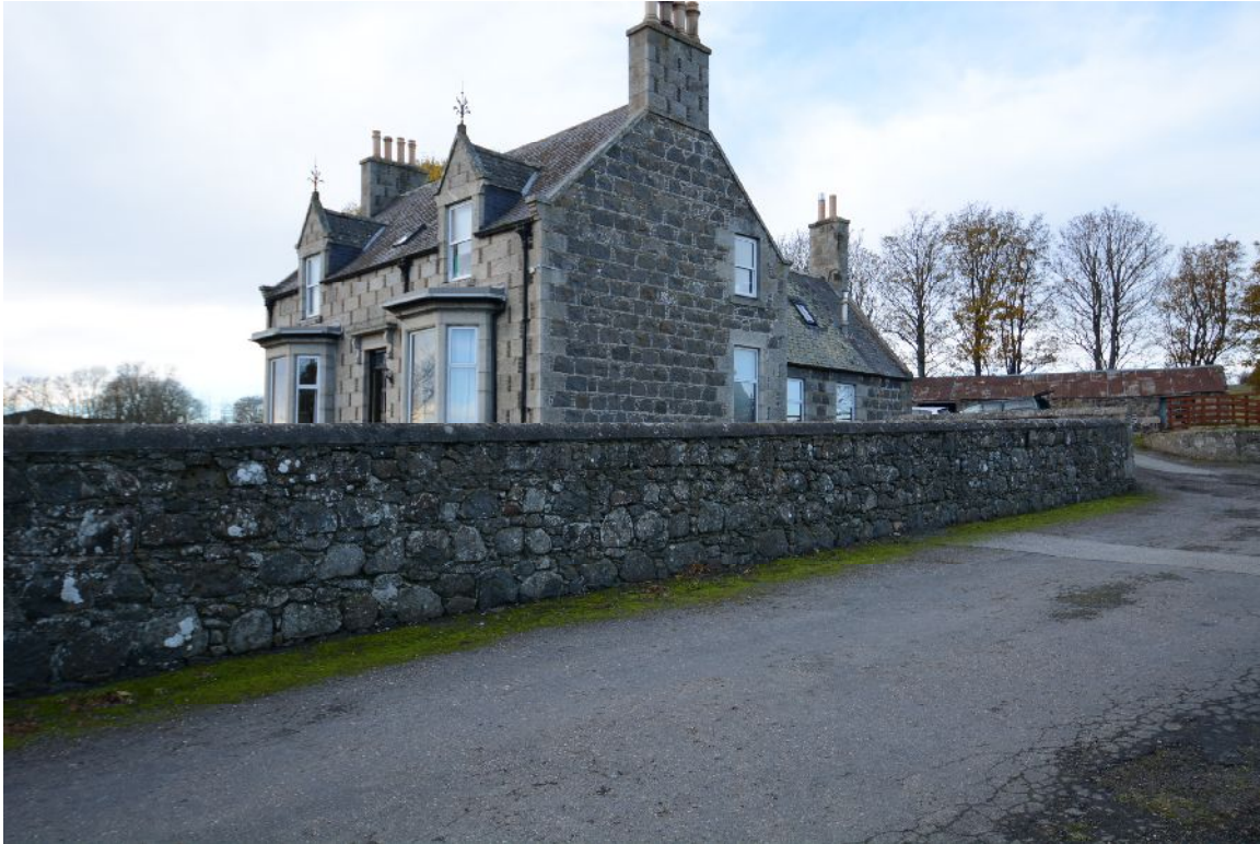
Illus 34 The farmhouse viewed from SE, from driveway between house and steading. Building 2 (cartshed) visible in background.
