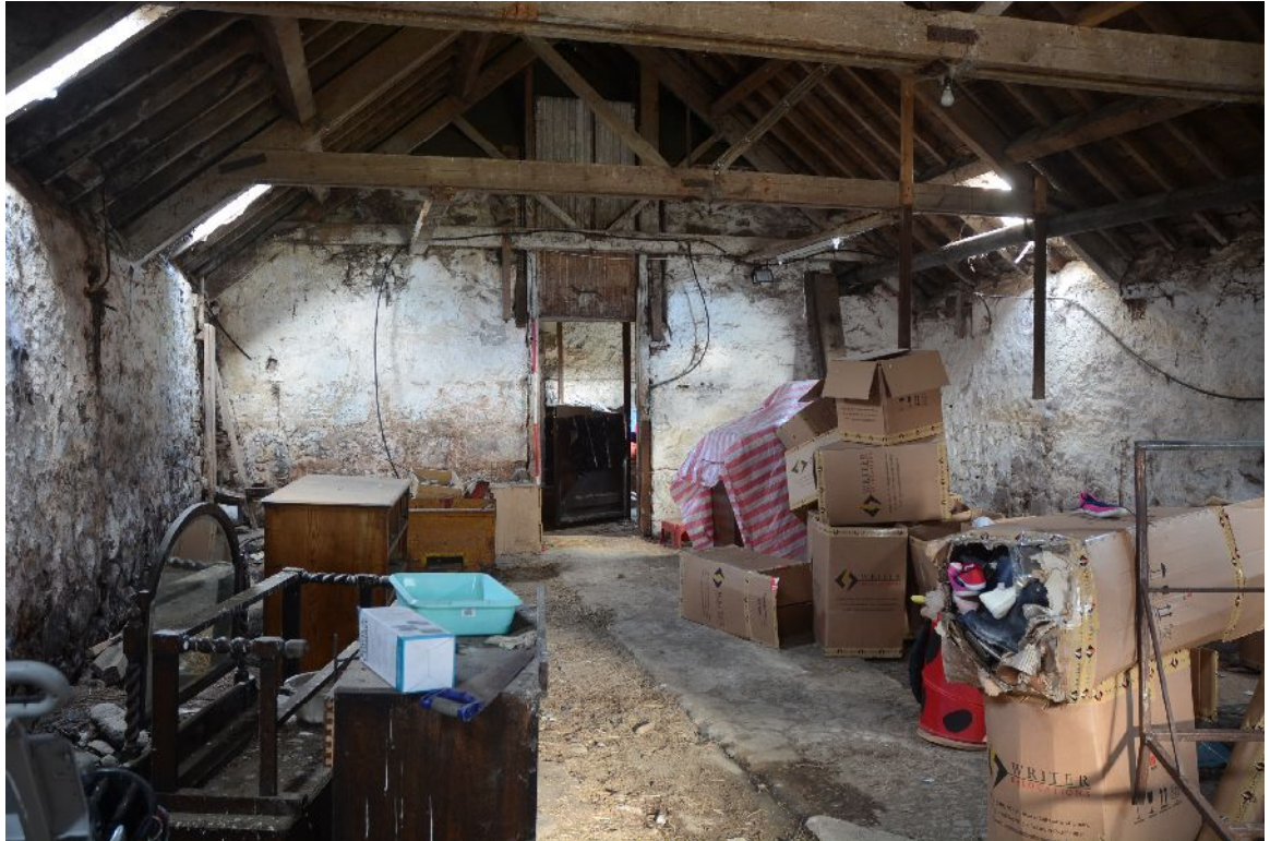
Illus 20 Interior of N Range Area B (W byre) looking E.
