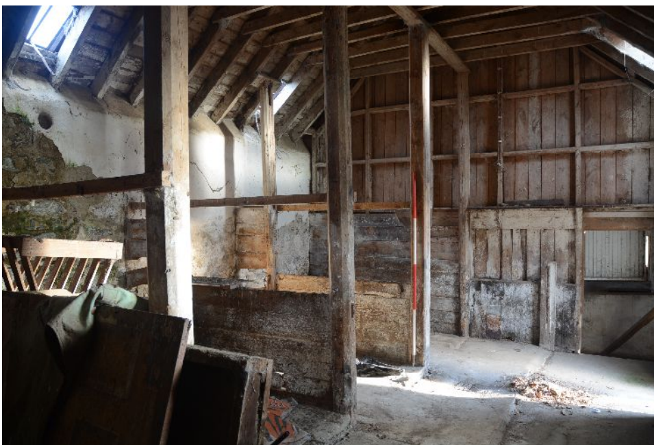
Illus 24 Stable (Area E) interior looking S
