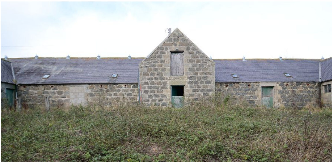
Illus 13 S wall N Range and Cross Range
