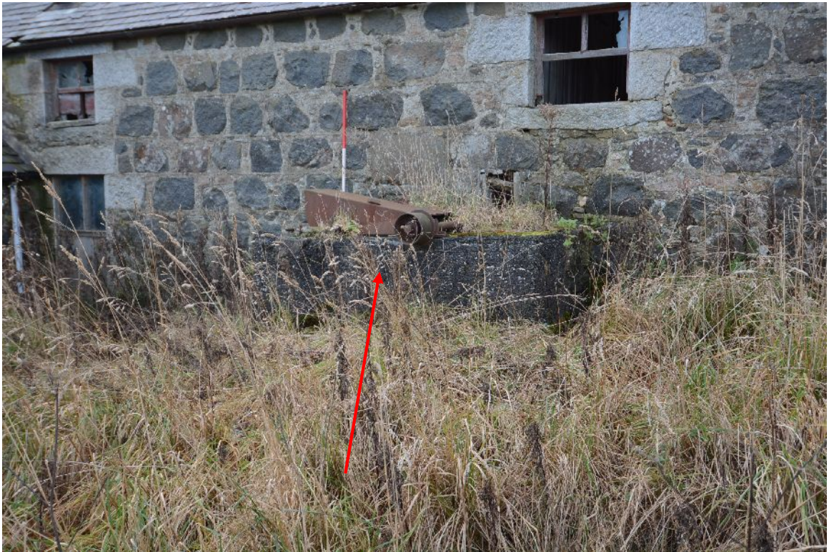
Illus 16 E wall of Cross Range with drive-shaft for thresher (red arrow)
