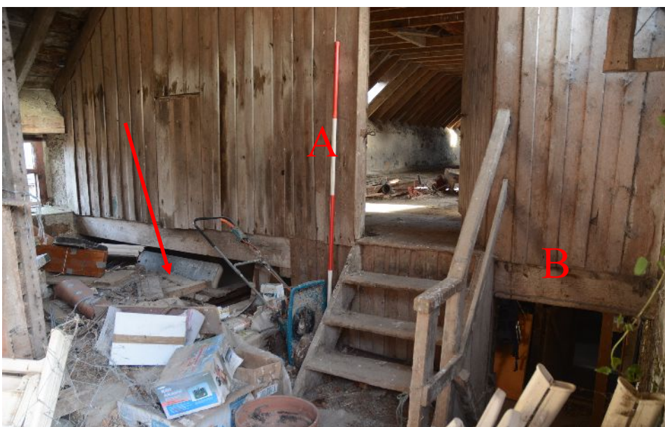
Illus 28 Door (A) into grain loft from sheaf barn Area L. On RHS stair down to straw barn (B) Arrow to thresher feed-in.
