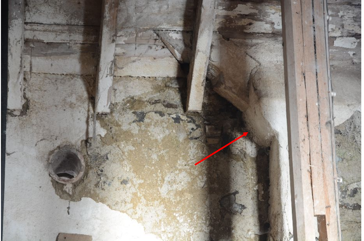
Illus 22 Truncated S end of gable of N range (Area D) now visible in stable Area E
