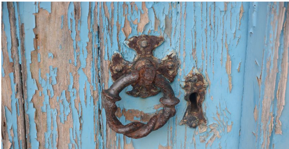
Illus 16 Late 19 th -century door fittings: door handle on D2
