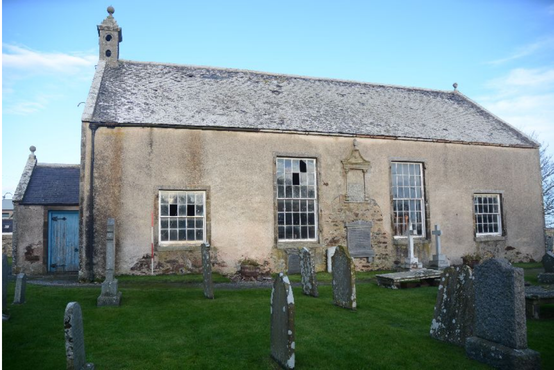
Illus 9 S wall. Porch on LHS
