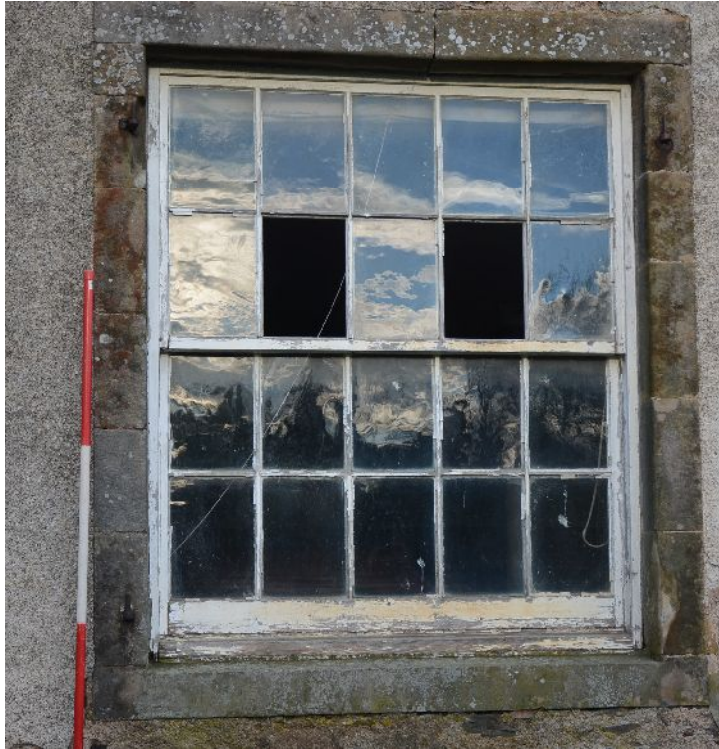
Illus 10 Detail of window W4 in S wall, showing ripples in glass
