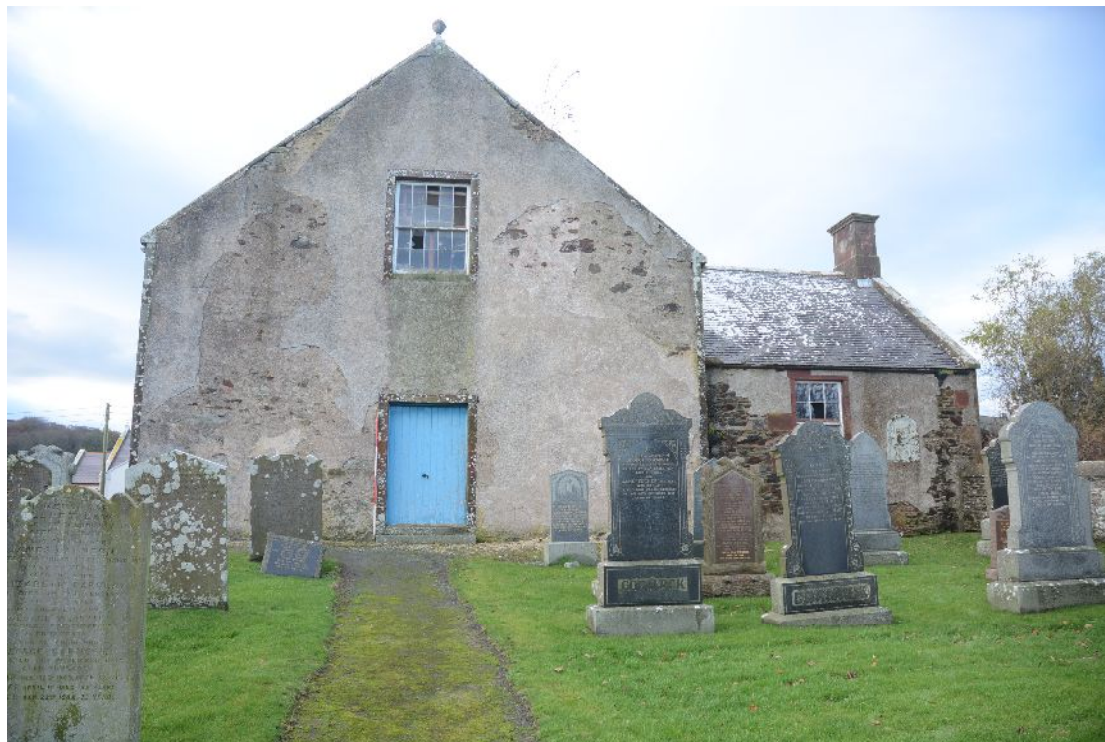
Illus 8 E wall, with vestry/session room on RHS
