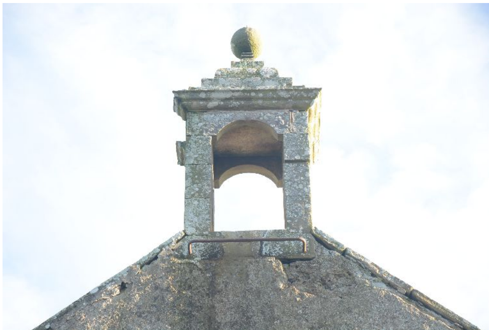
Illus 7 Bellcote from W. Note iron bar that restrained the bell rope
