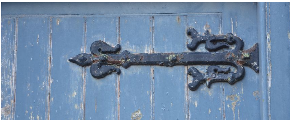
Illus 17 Late 19 th -century door fittings: hinge on D1 (same hinges on porch door D2)
