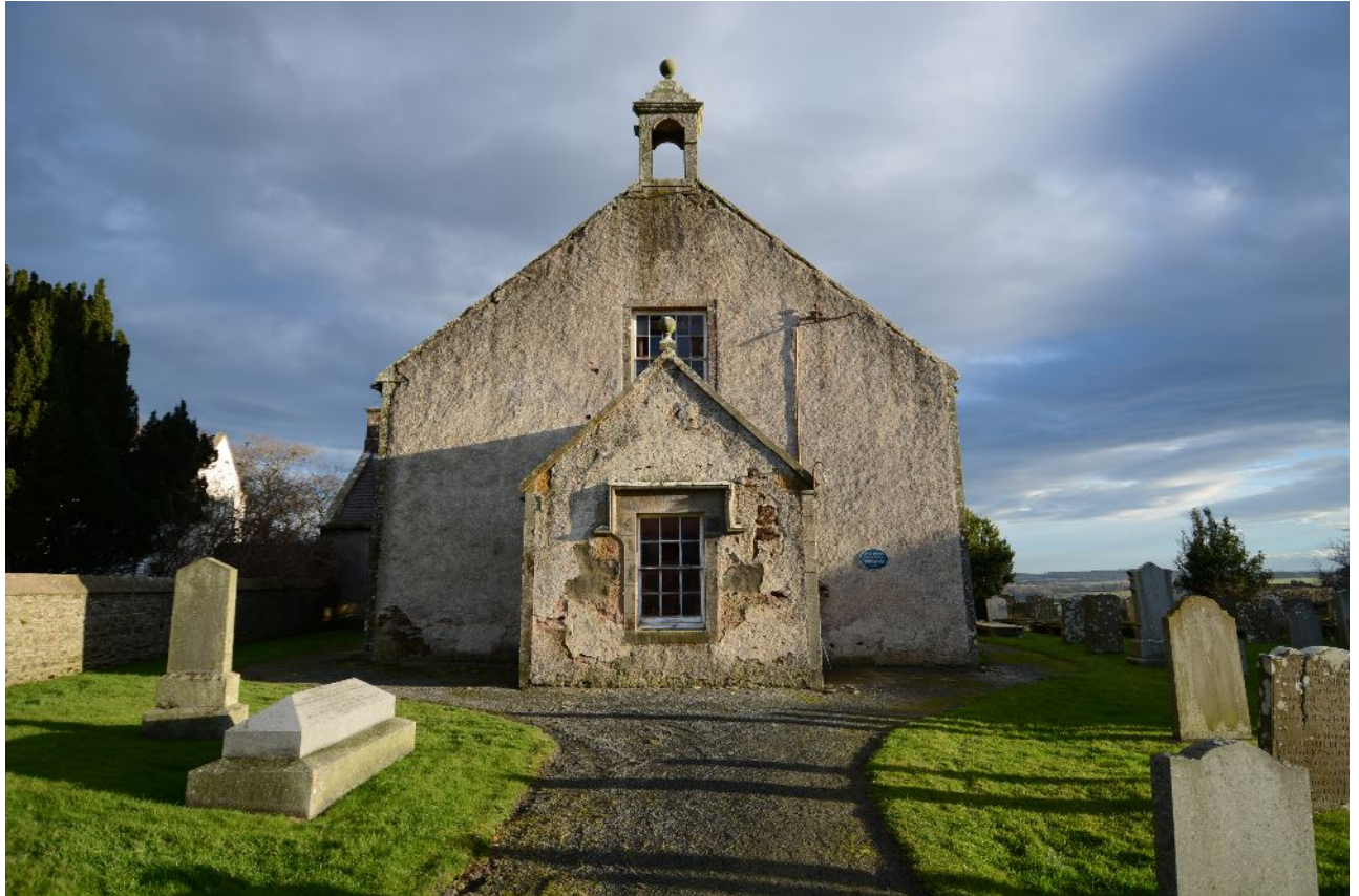
Illus 6 Alvah Church W wall and porch.
