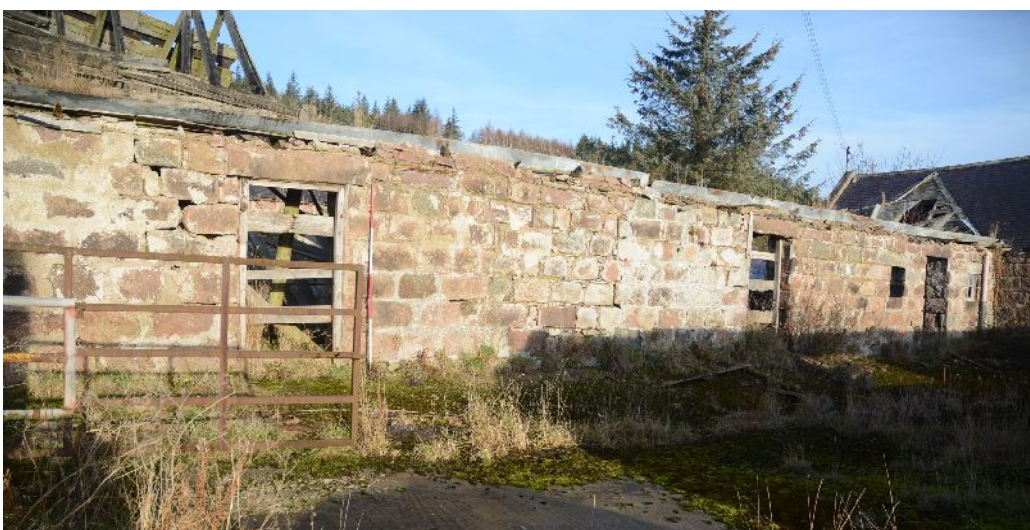
Illus 11 S wall of N range from court, looking NE
