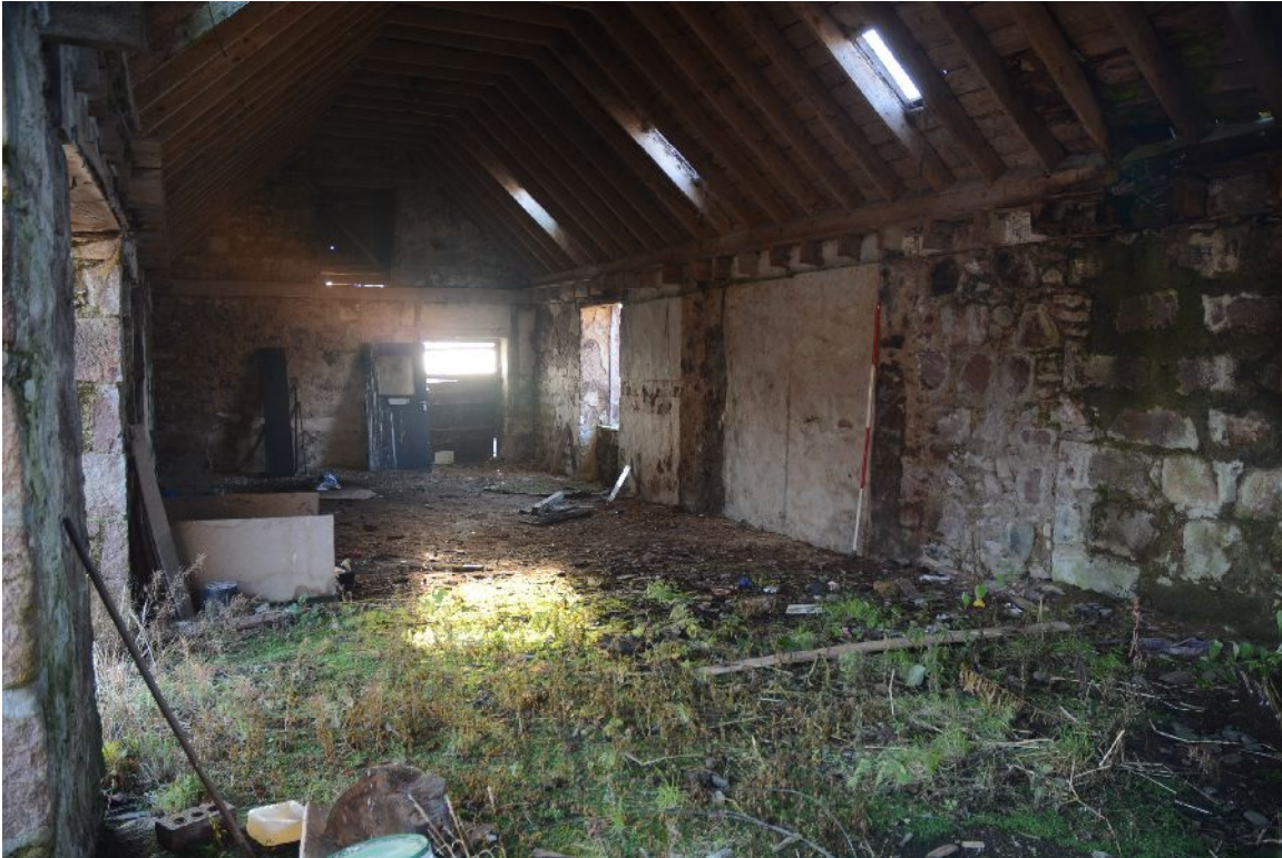
Illus 16 Interior of E range looking S. Stubs of loft joists visible.
