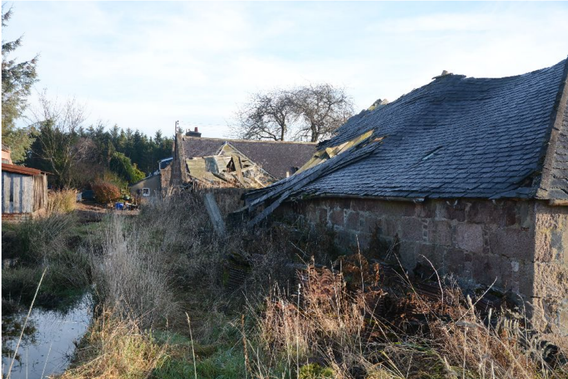
Illus 12 N wall of N range looking E
