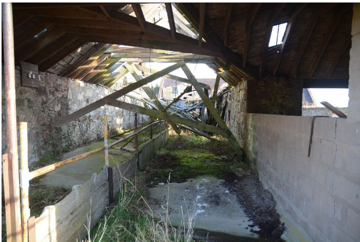
Illus 15 Interior of N range looking E
