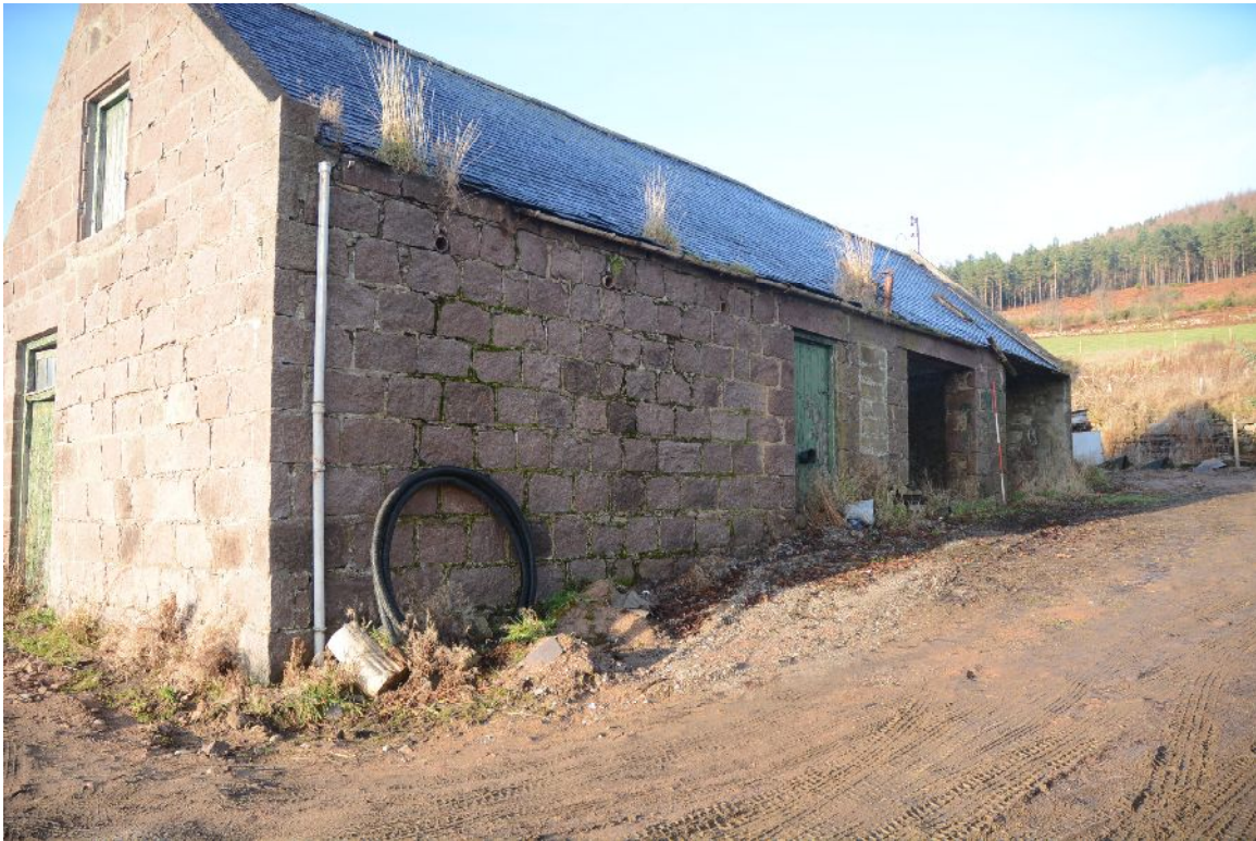
Illus 13 E wall of E range, looking N. Shows cart bays
