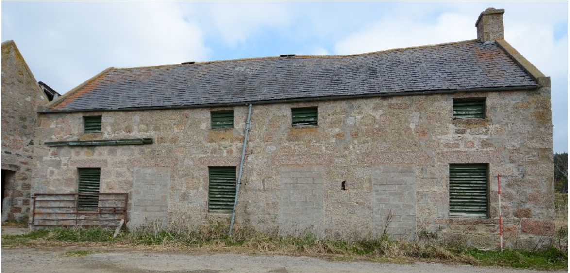
Illus 14 S wall of Building A
