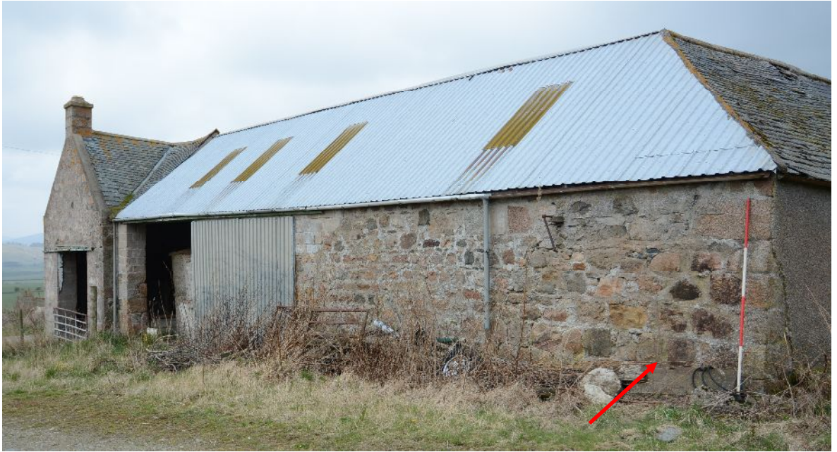
Illus 20 E wall of Buildings B and C, looking S. Note larger, squared blocks in wall where mill wheel shown on 1 st OS map (arrow)
