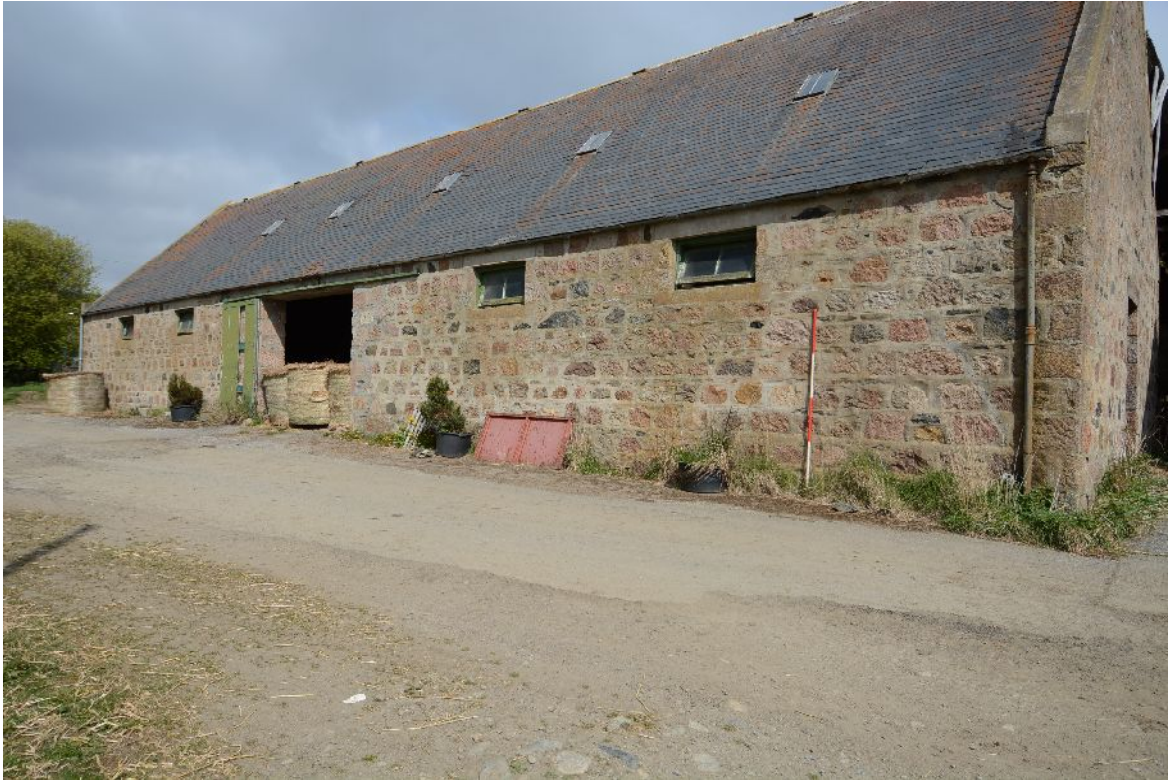
Illus 25 Exterior of S wall of Building G
