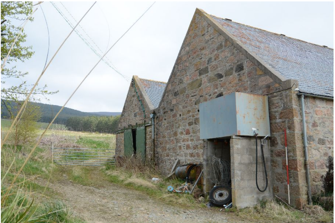
Illus 28 W gables of Buildings G (foreground) and H (with green doors)
