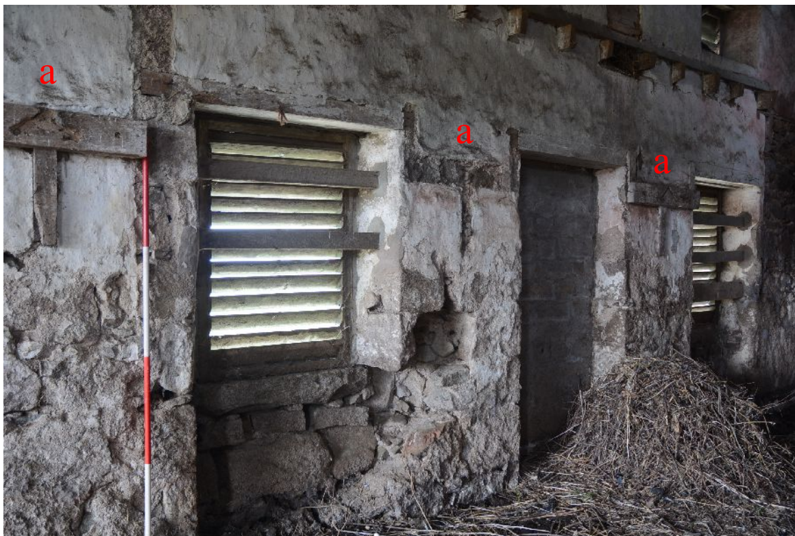
Illus 17 Interior of Building A looking W along S wall. Scars of harness supports marked (a).
