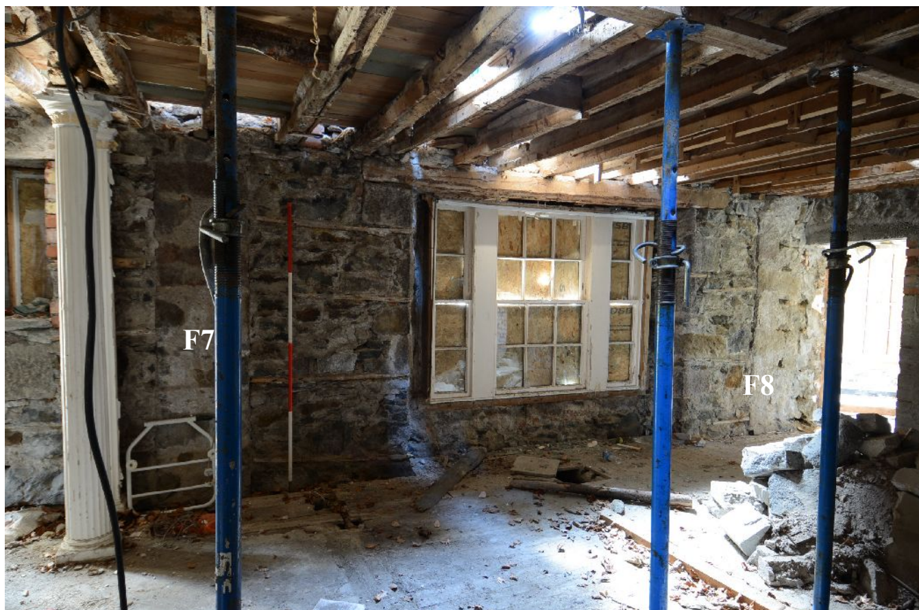
Illus 44 Room 3 Raggles of earlier walls on inside of S wall.
