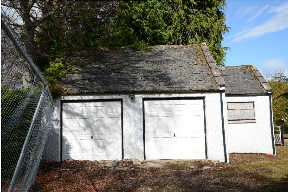
Illus 66 Garage (building C) from SW
