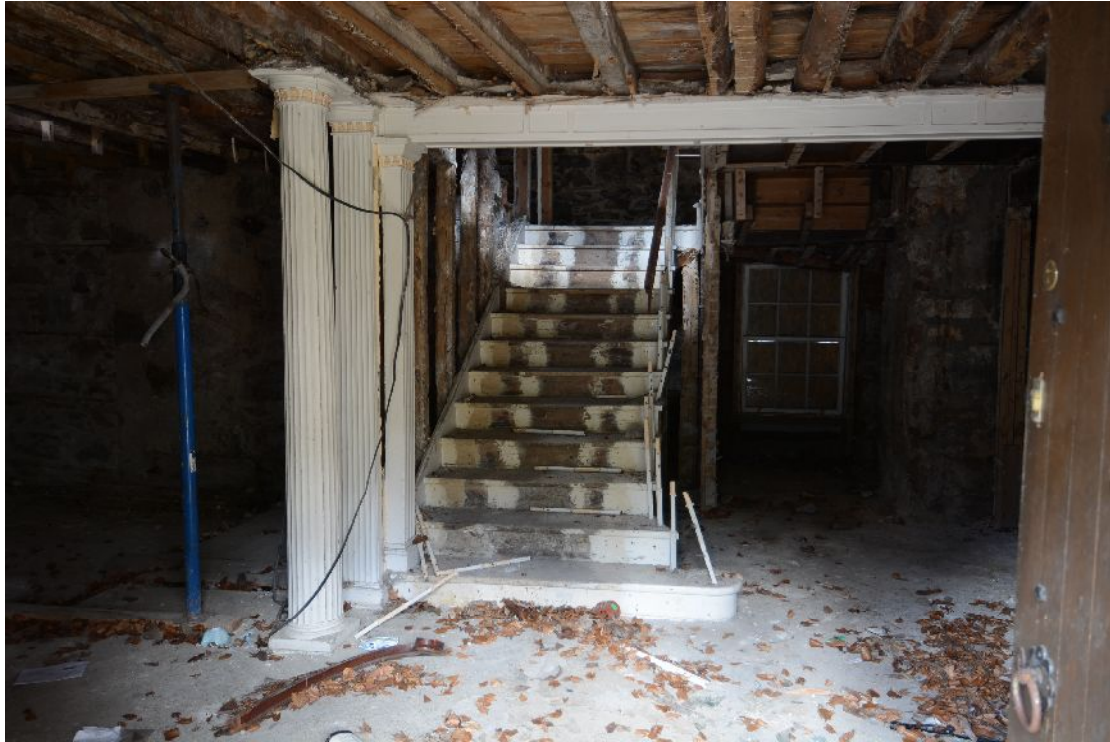
Illus 39 Entrance hall looking N to stair
