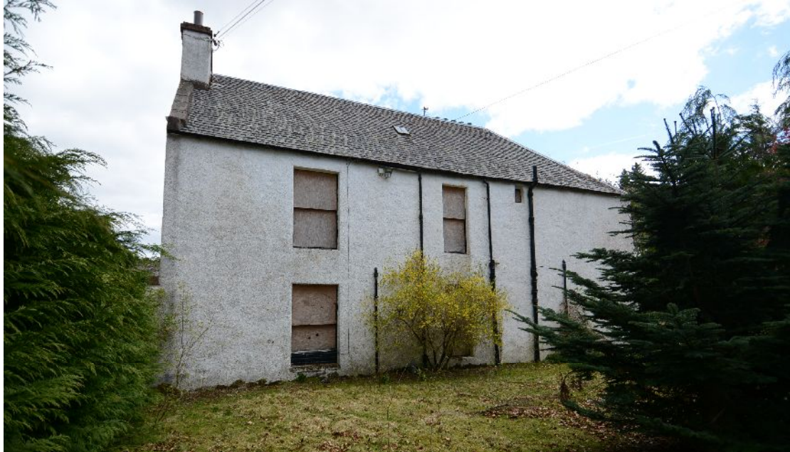
Illus 36 W facade of main building looking E
