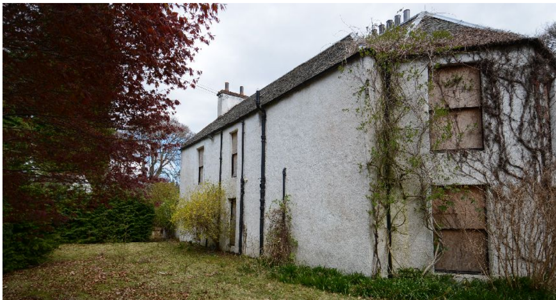
Illus 37 W facade of main building looking N
