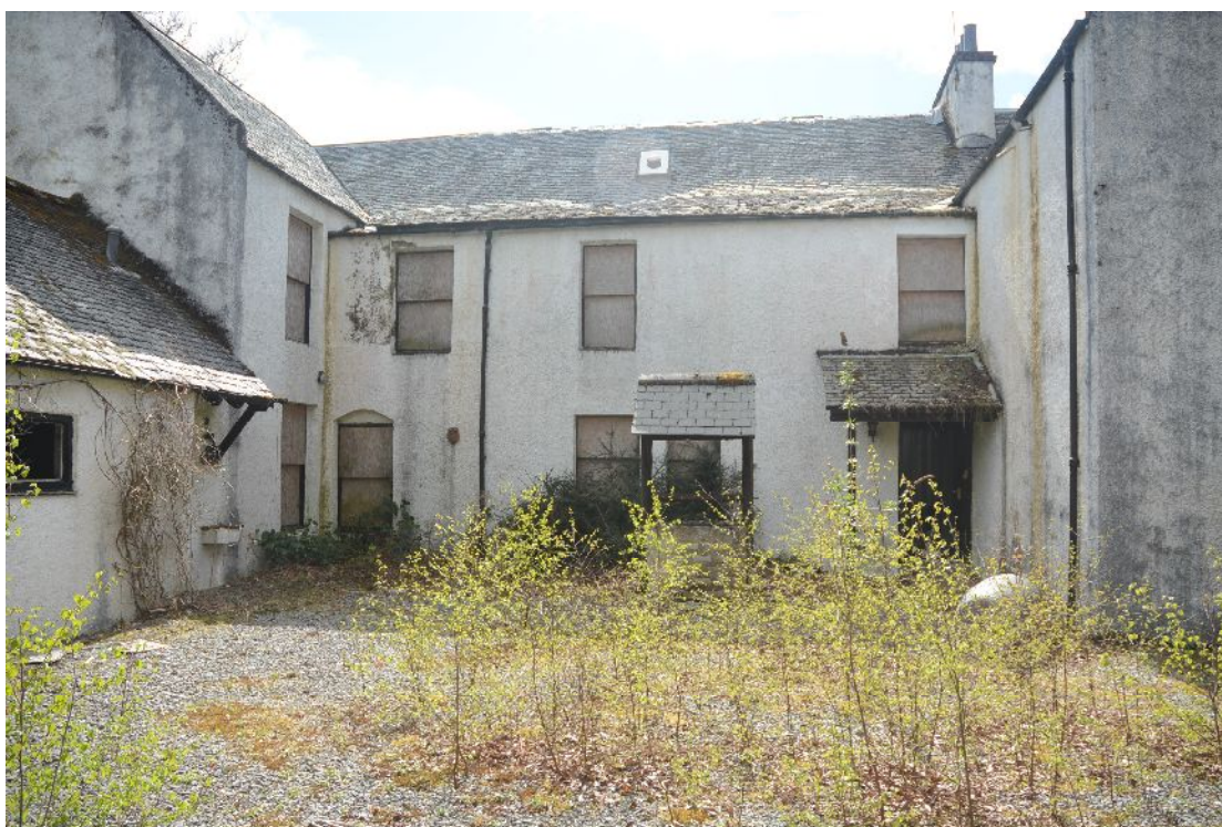
Illus 24 View from N into courtyard, showing lower pitch of roof over back passageway.
