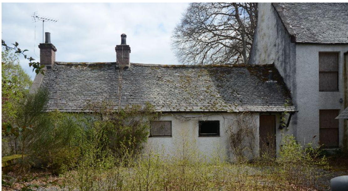
Illus 32 W wall of NE extension, facing into courtyard
