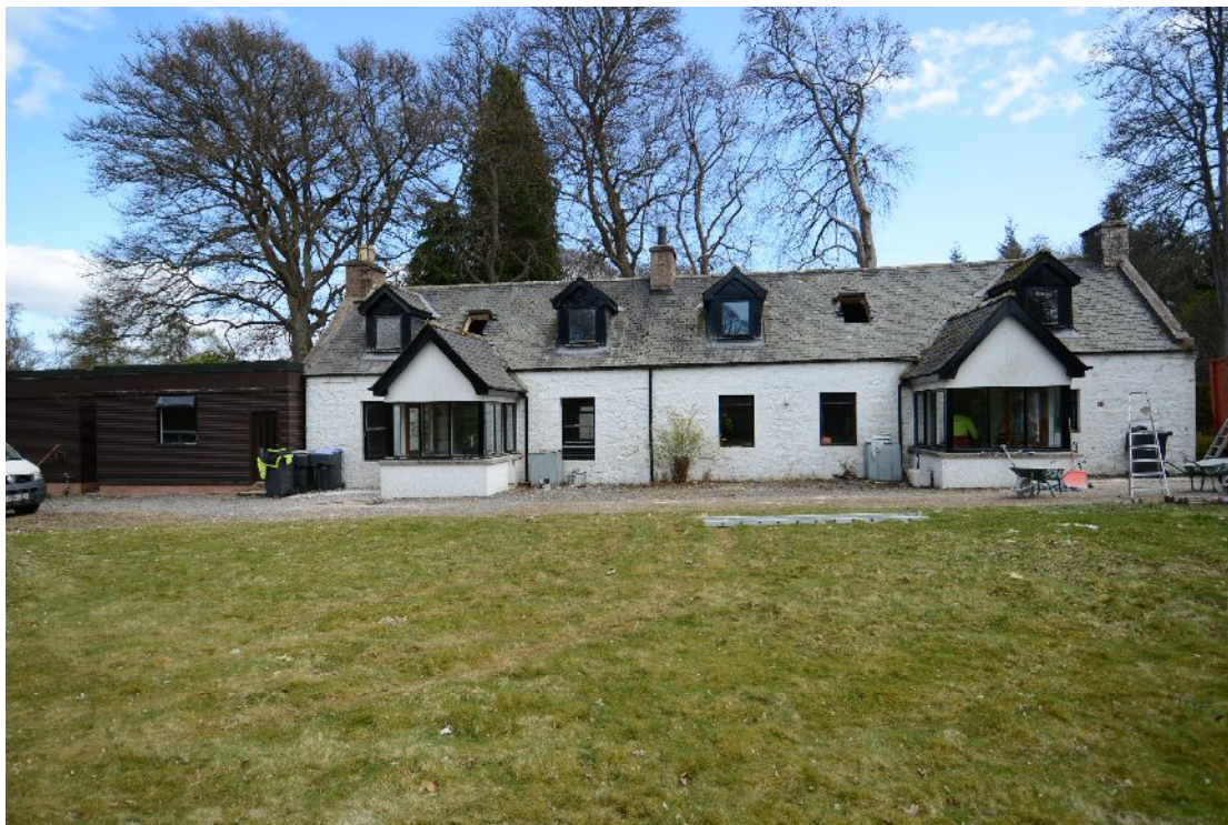
Illus 61 W elevation of coach house
