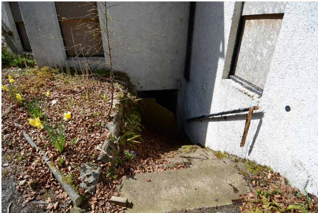
Illus 54 Cellar door looking W
