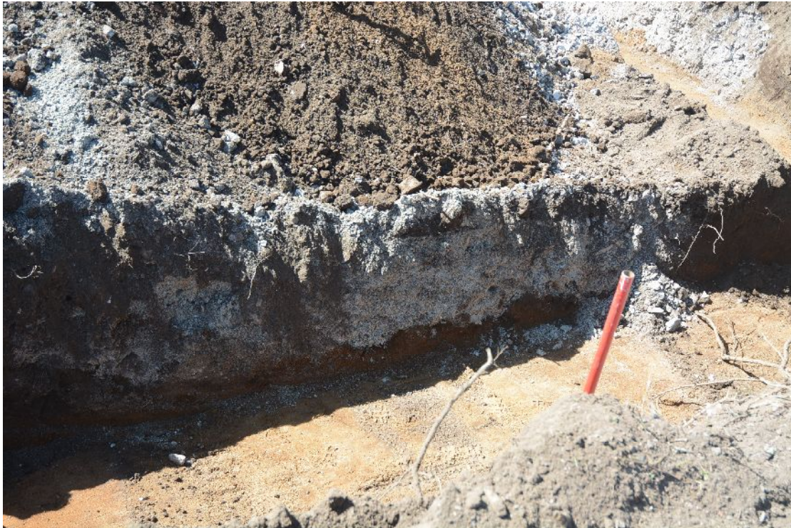
Illus 8 Trench 3 W section with sub-base to natural
