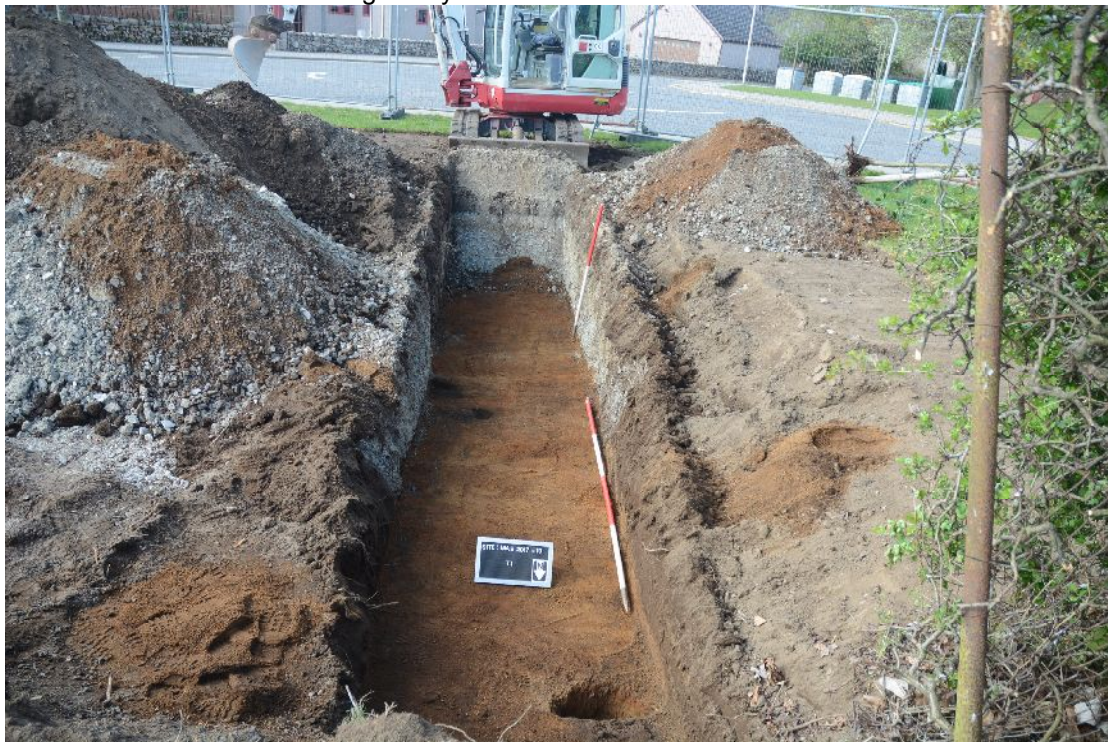
Illus 3 Trench 1 looking S. Contexts 1-3 shown excavated. Grey sub-base visible in sections.
