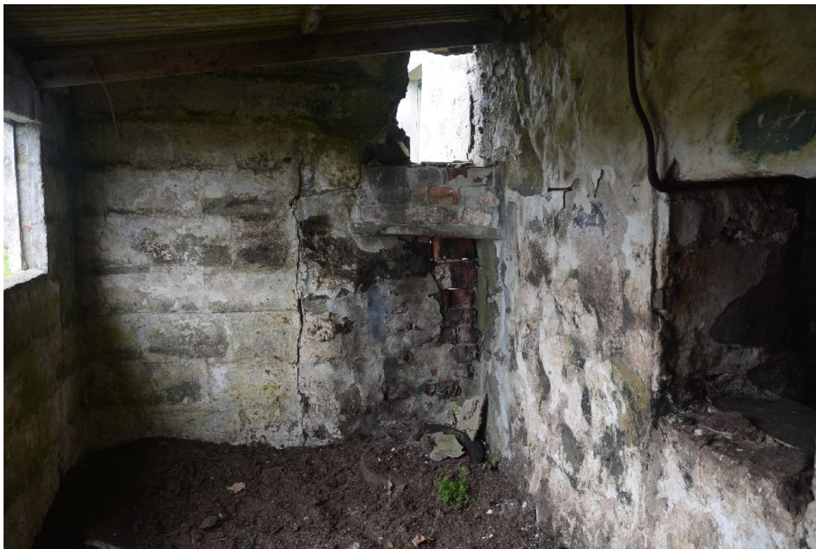
Illus 15 Building 4, Interior SW corner. Window into byre at RHS.
