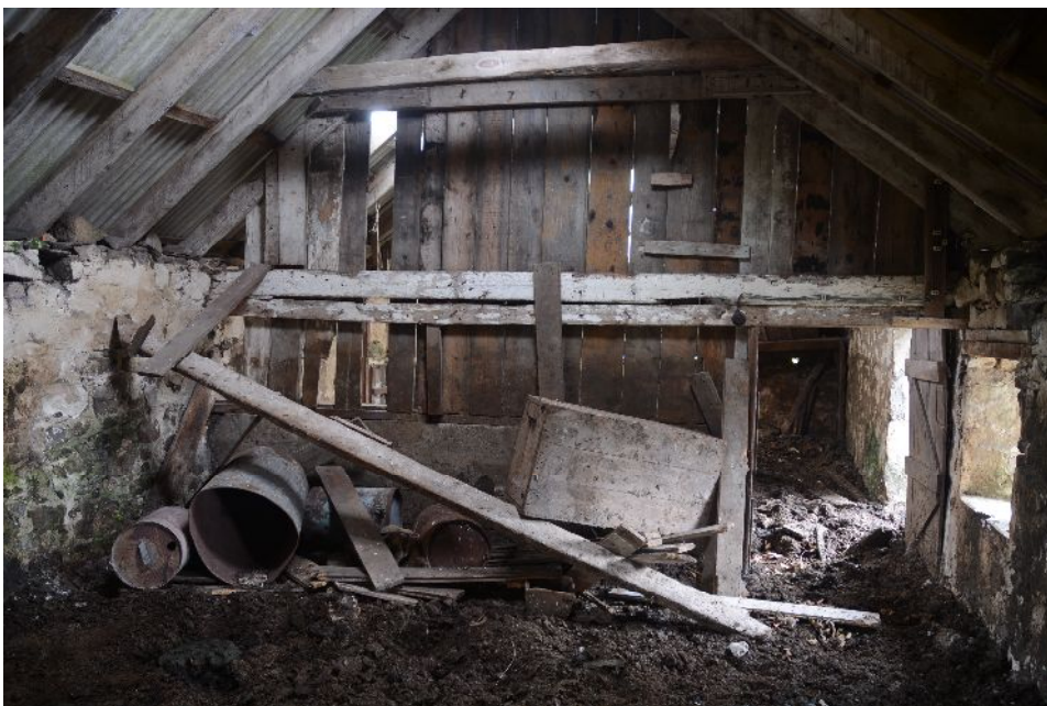
Illus 12 Building 2. Interior from door D5 looking N to partition.
