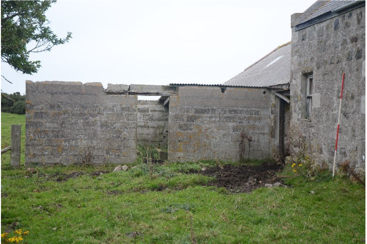
Illus 13 Building 3 looking N
