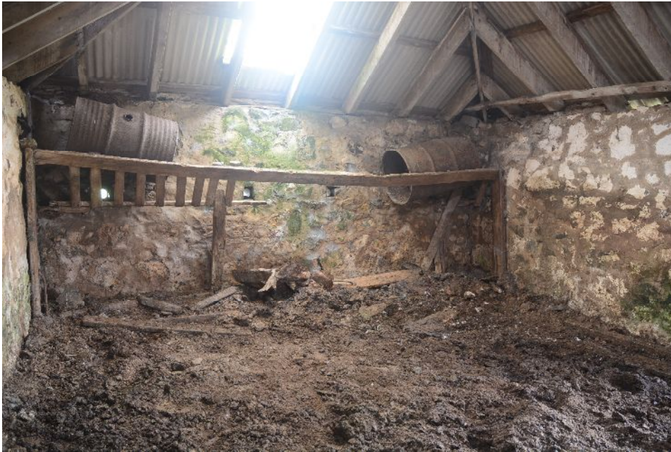
Illus 11 Building 2. Interior looking N, in N room
