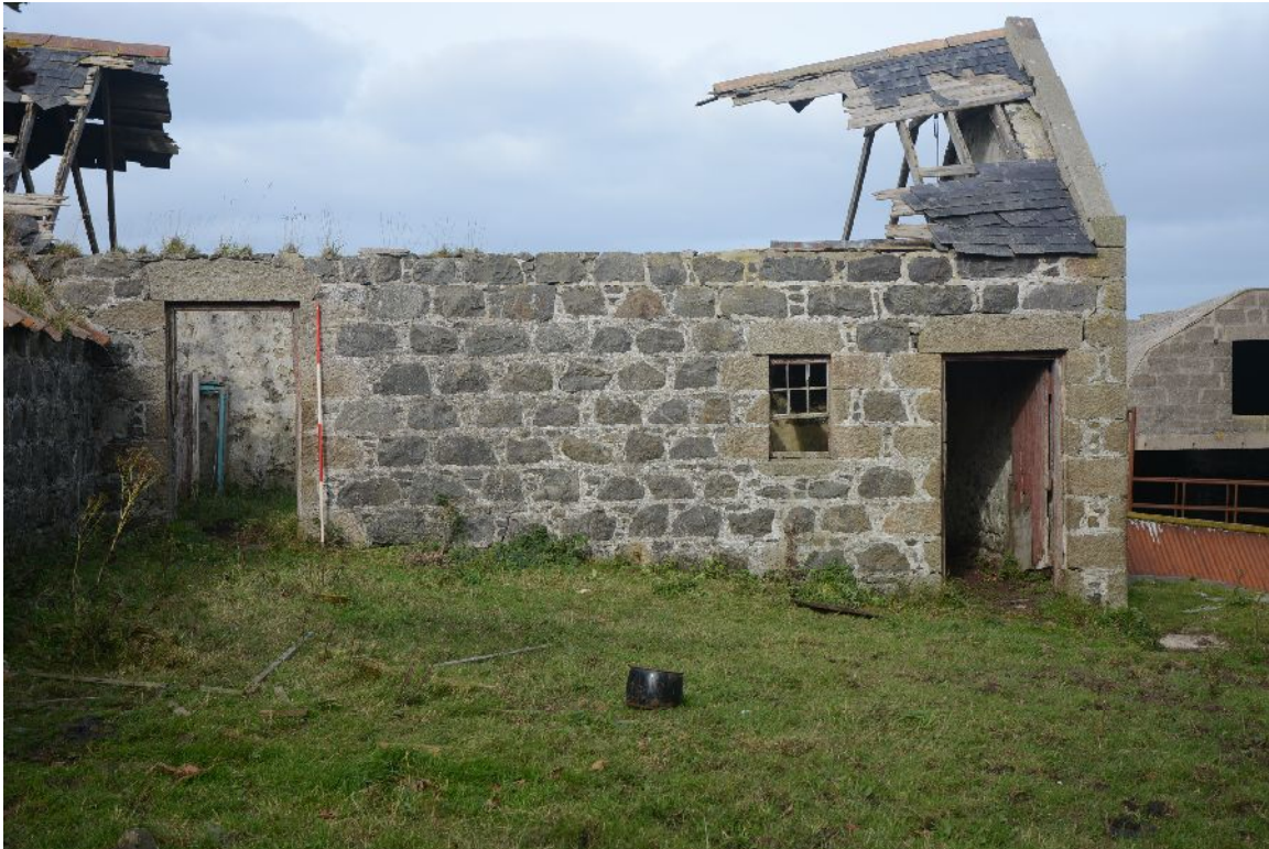
Illus 23 Building 3 N range S wall
