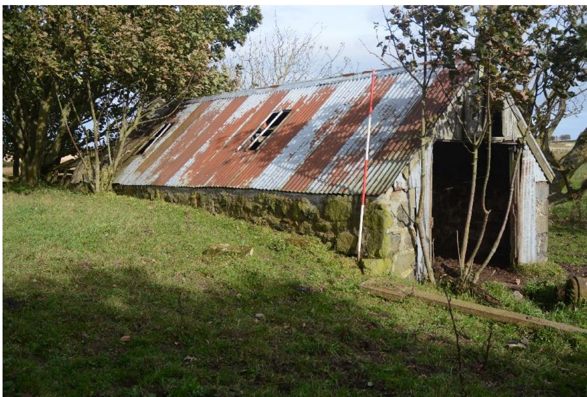
Illus 13 Building 2, W wall built into slope of hillside
