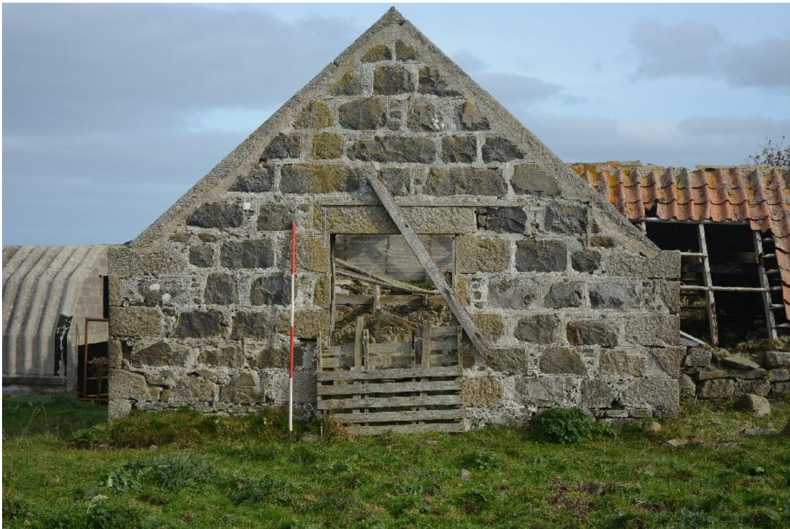
Illus 25 Building 3. N range W wall and door D4
