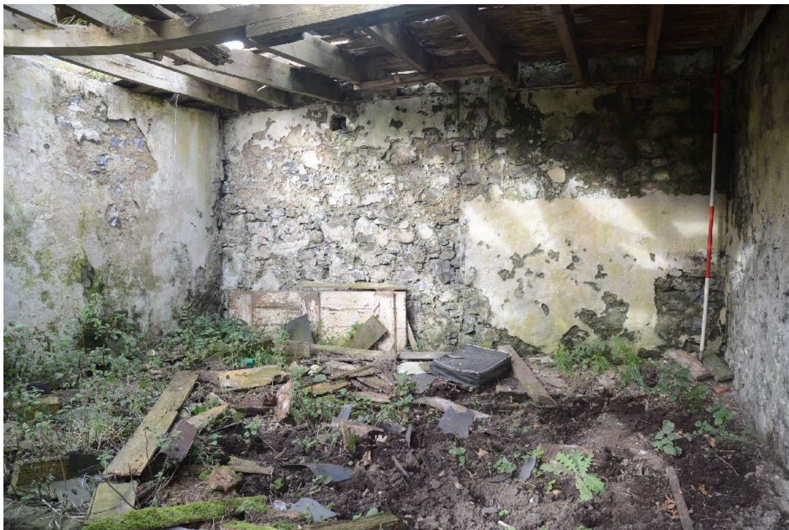
Illus 28 Building 3. N range, E room- probable stable with loft above.
