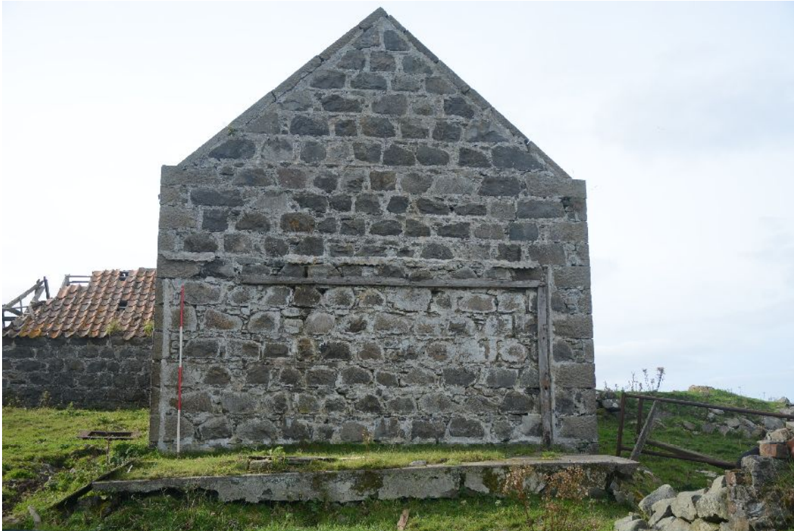
Illus 24 Building 3. N range, E wall with raggle of a lean-to.
