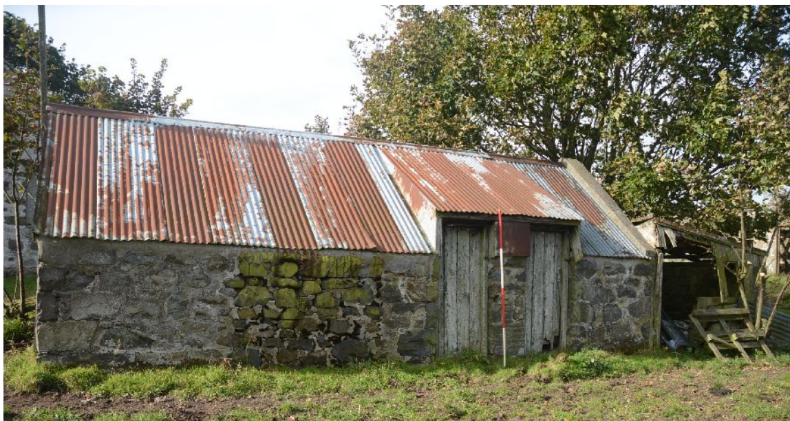
Illus 9 Building 2. E wall
