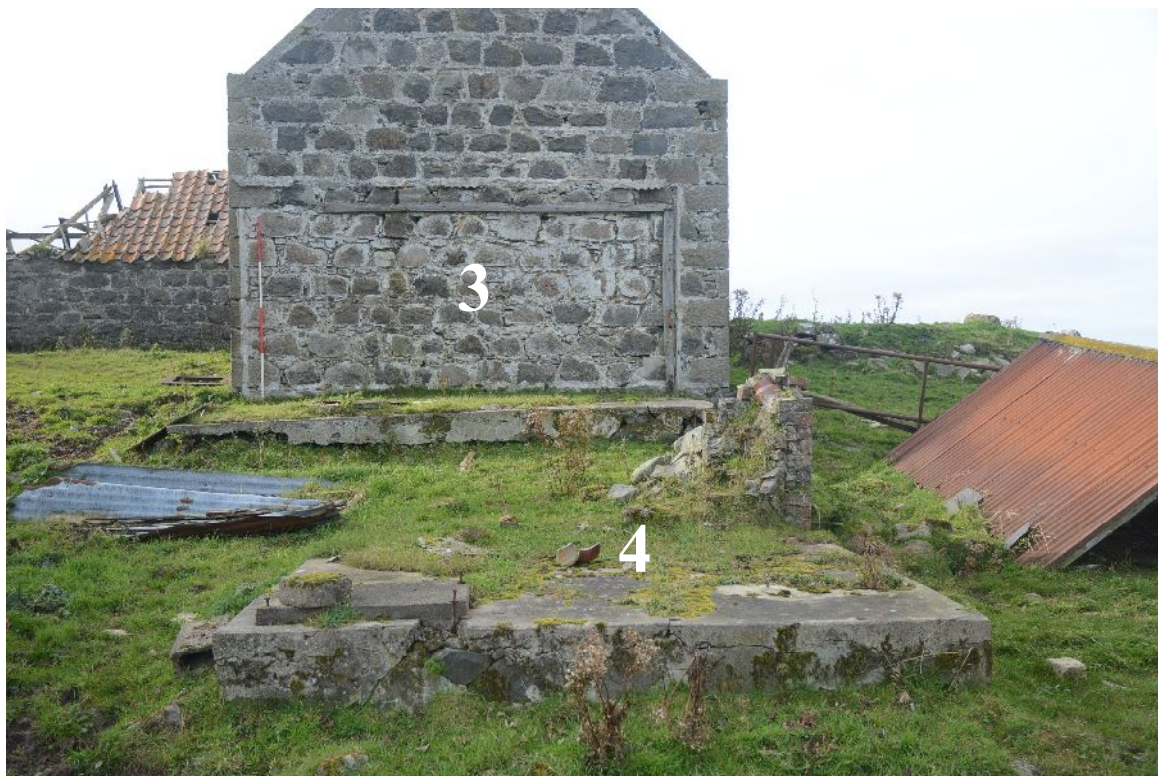
Illus 35 Concrete floor of Building 4
