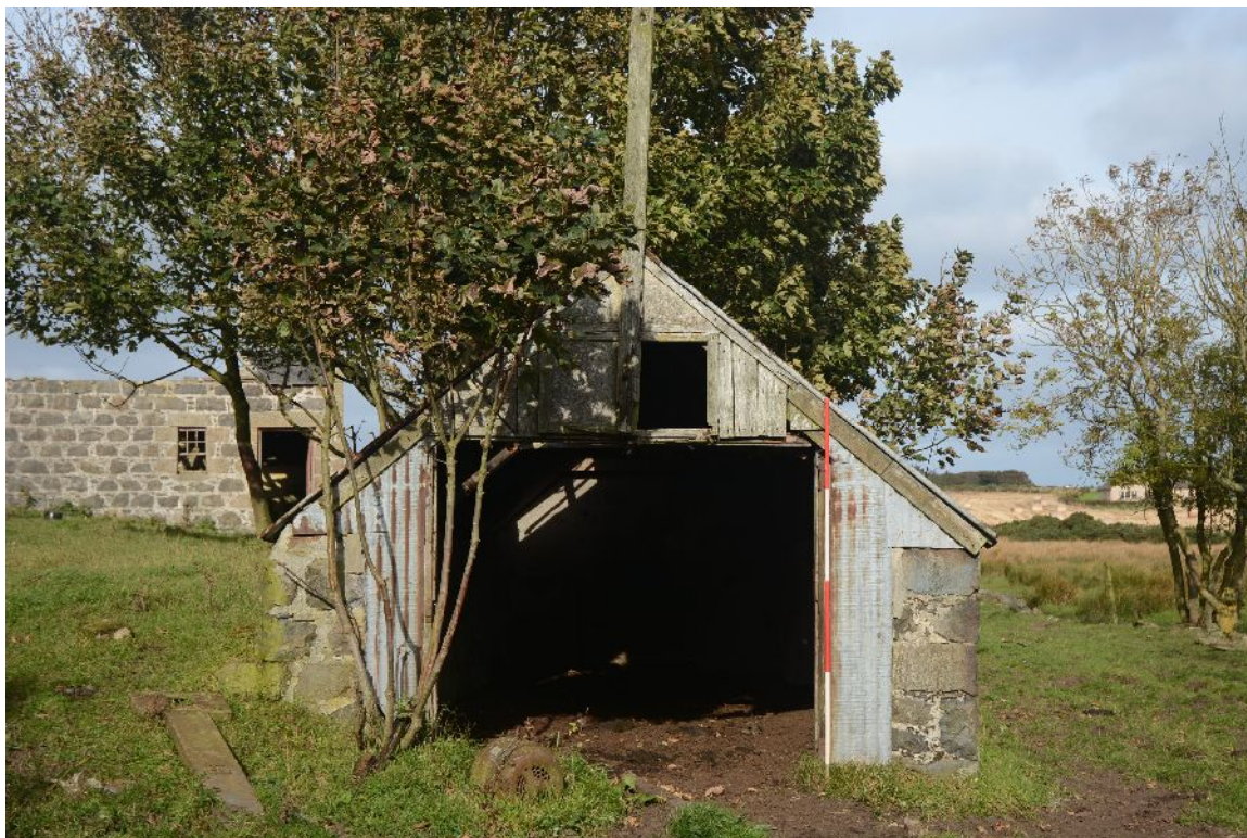
Illus 12 Building 2. S wall, D4
