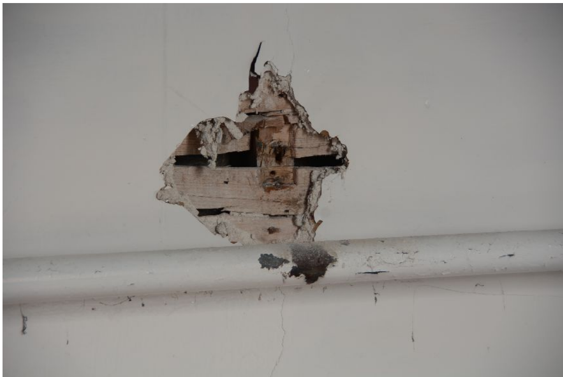
Illus 40 Lathe and plaster exposed on inside of N wall
