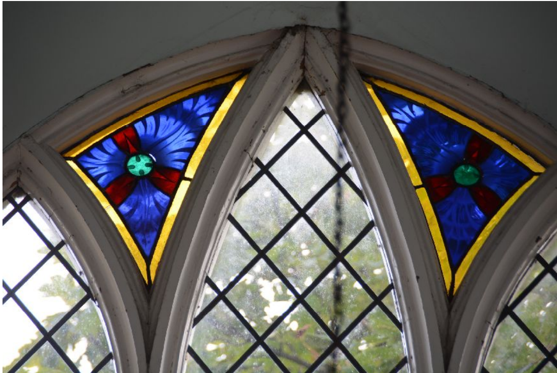
Illus 31 Detail of stained glass panels at top of W7
