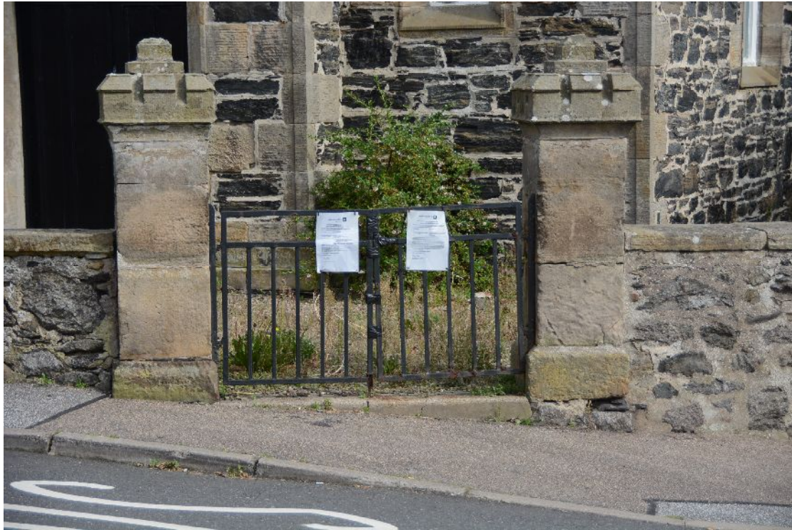
Illus 51 Entrance gate.
