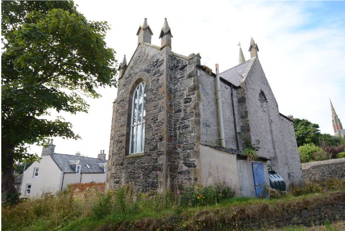
Illus 29 E gable from NE
