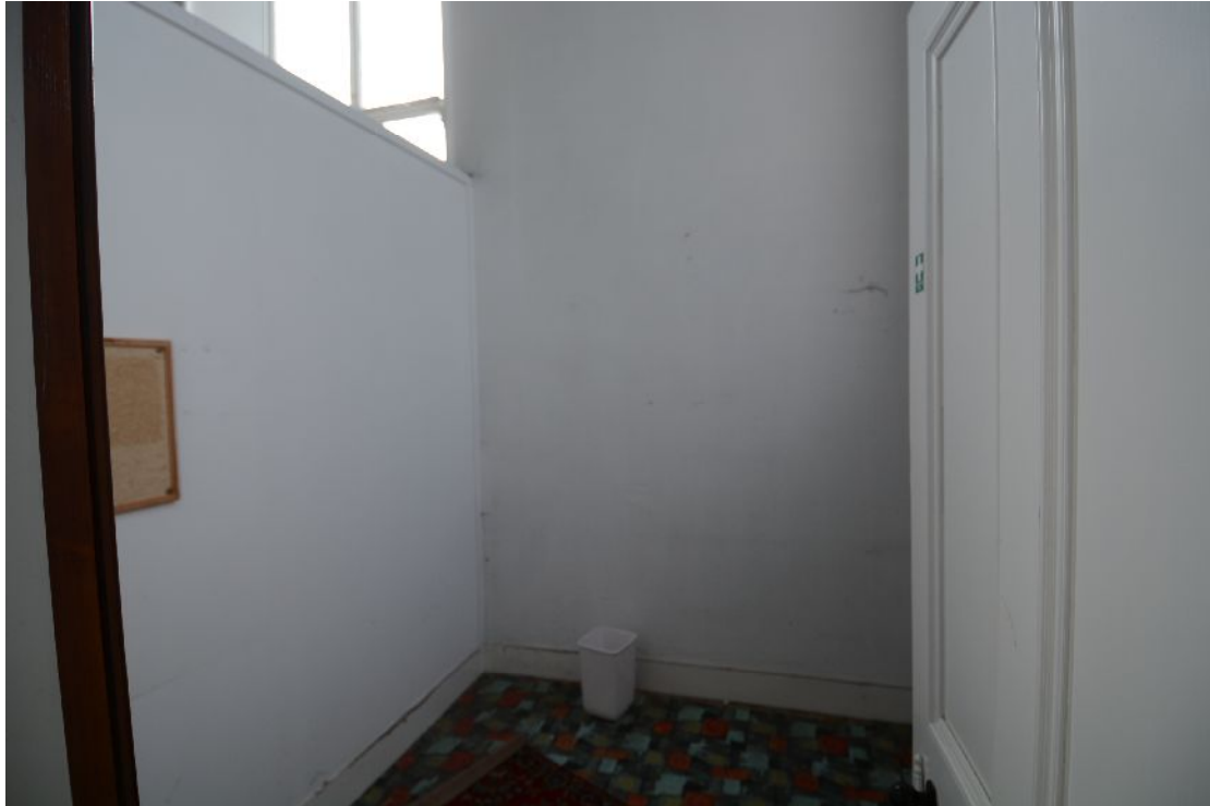
Illus 37 Partitioned room in NW corner
