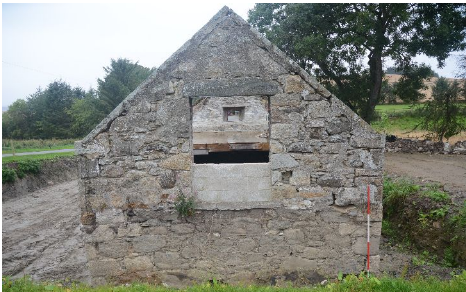
Illus 11 E wall and window W1
