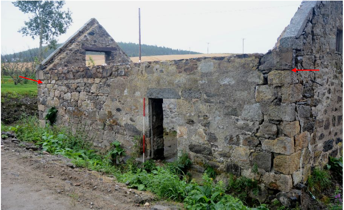
Illus 8 N wall, looking E. Arrows indicate two, possibly additional upper courses.
