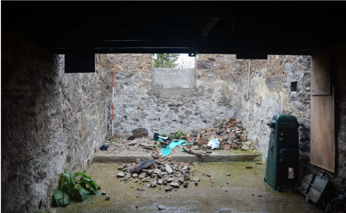
Illus 21 Interior looking E
