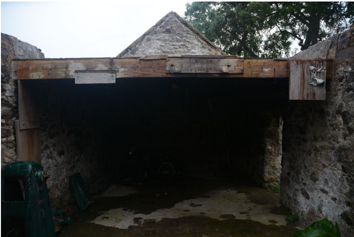
Illus 22 Interior looking W, with loft floor.
