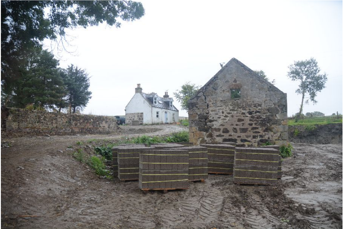
Illus 2 General view looking NE with the mill in the foreground, the house behind and the remains of the steading wall on the LHS.
