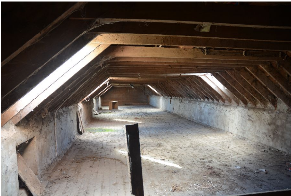
Illus 60 Building H. Interior of loft looking W from stair
