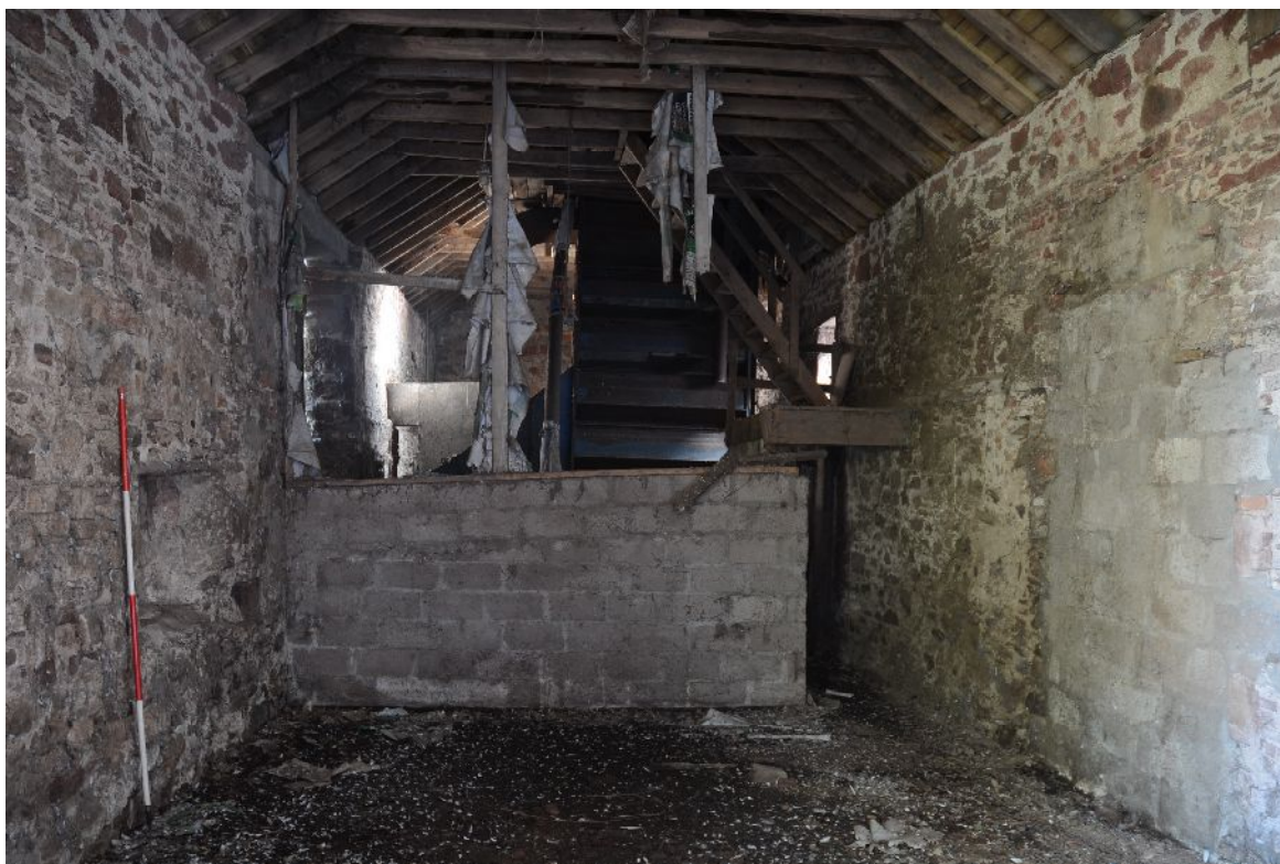
Illus 37 Building C interior looking S. Blocking F2 on RHS
