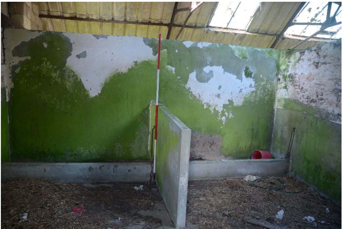
Illus 46 Building D. SW corner. Tied cattle stalls.
