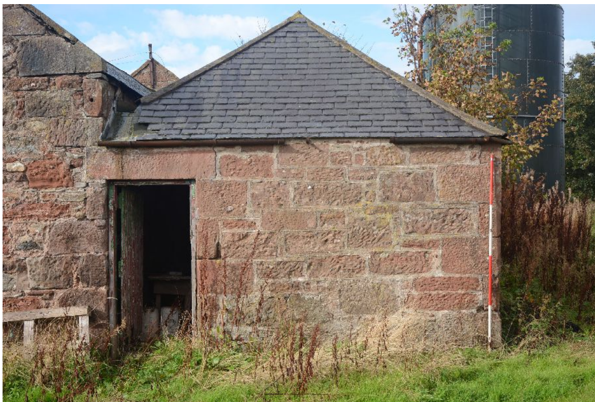
Illus 17 S wall of Building A, with D1
