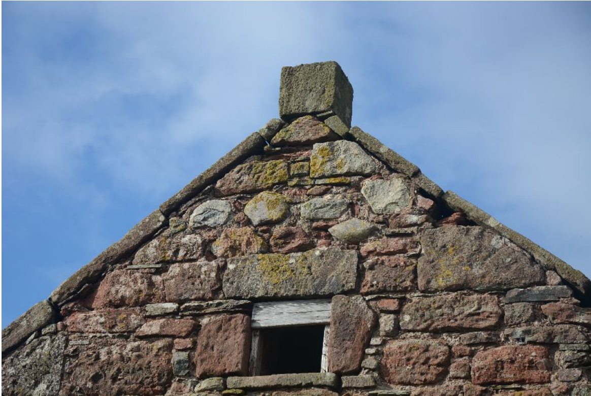
Illus 25 Building B S gable finial and F1 vent
