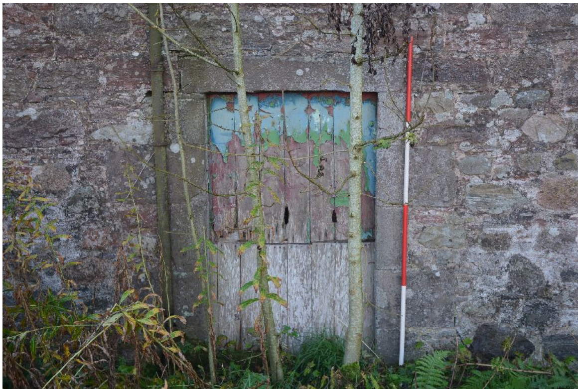
Illus 29 Building C, door D11
