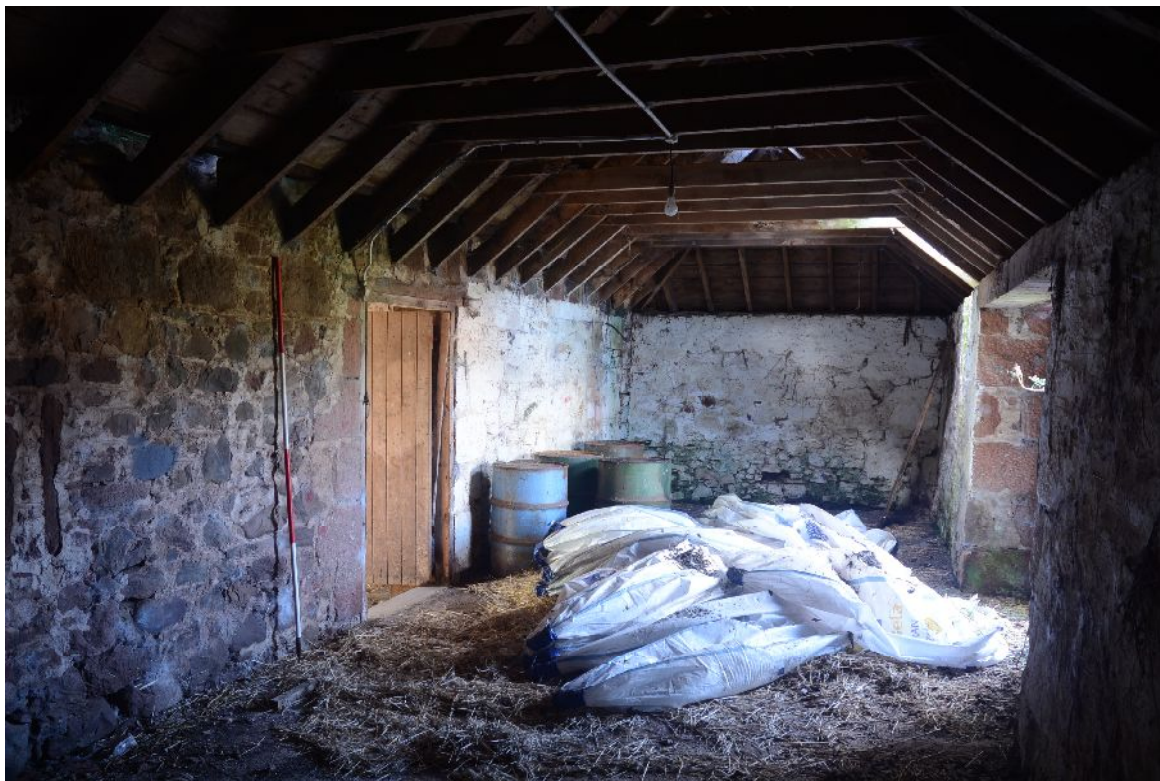
Illus 21 Building A, Area A2, looking N
