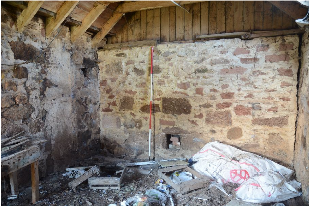
Illus 20 Building A, area A1 looking N from door D1
