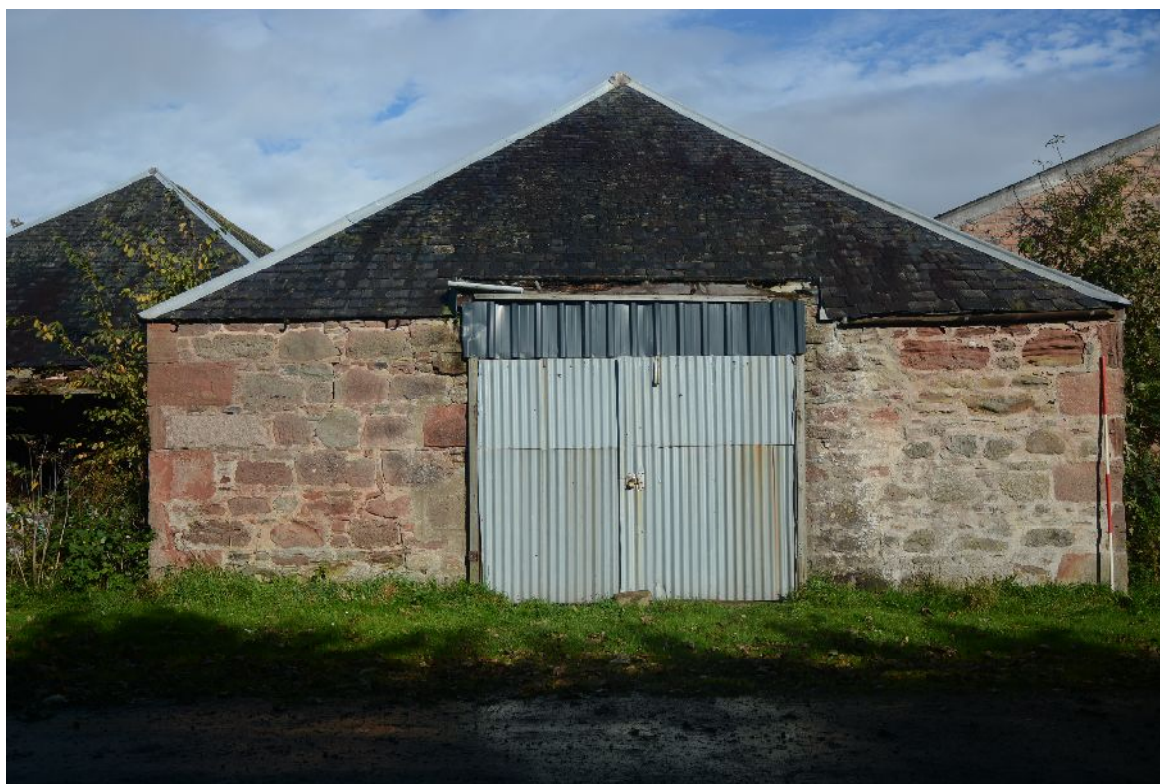
Illus 49 Building F from W. Door D23.
