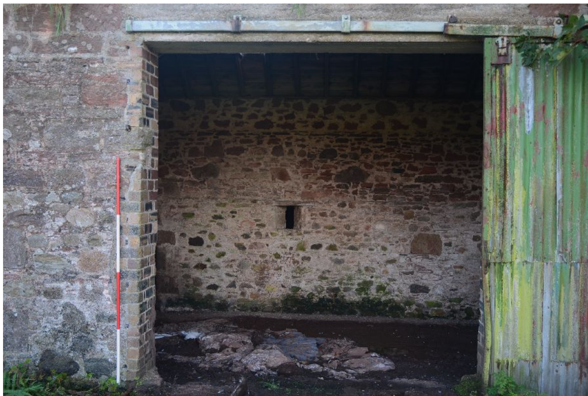
Illus 28 Building C, door D10
