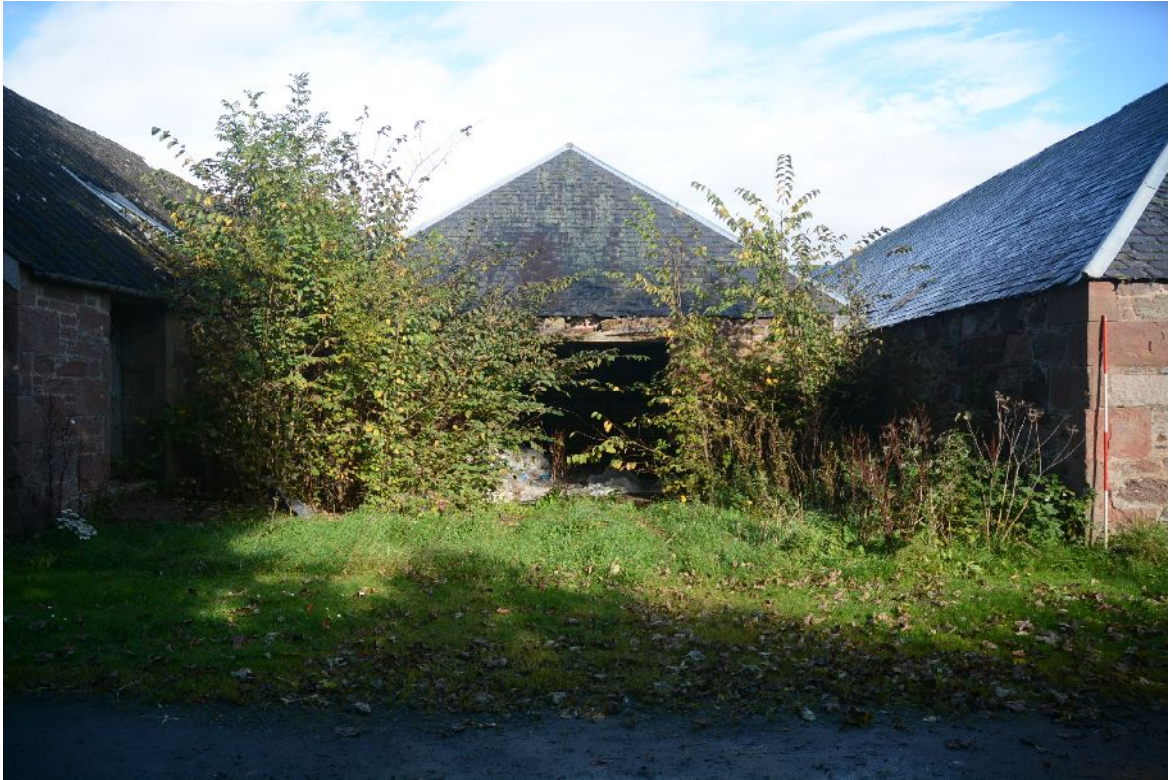
Illus 47 Building E. Roofed cattle court from W. Door D21.
