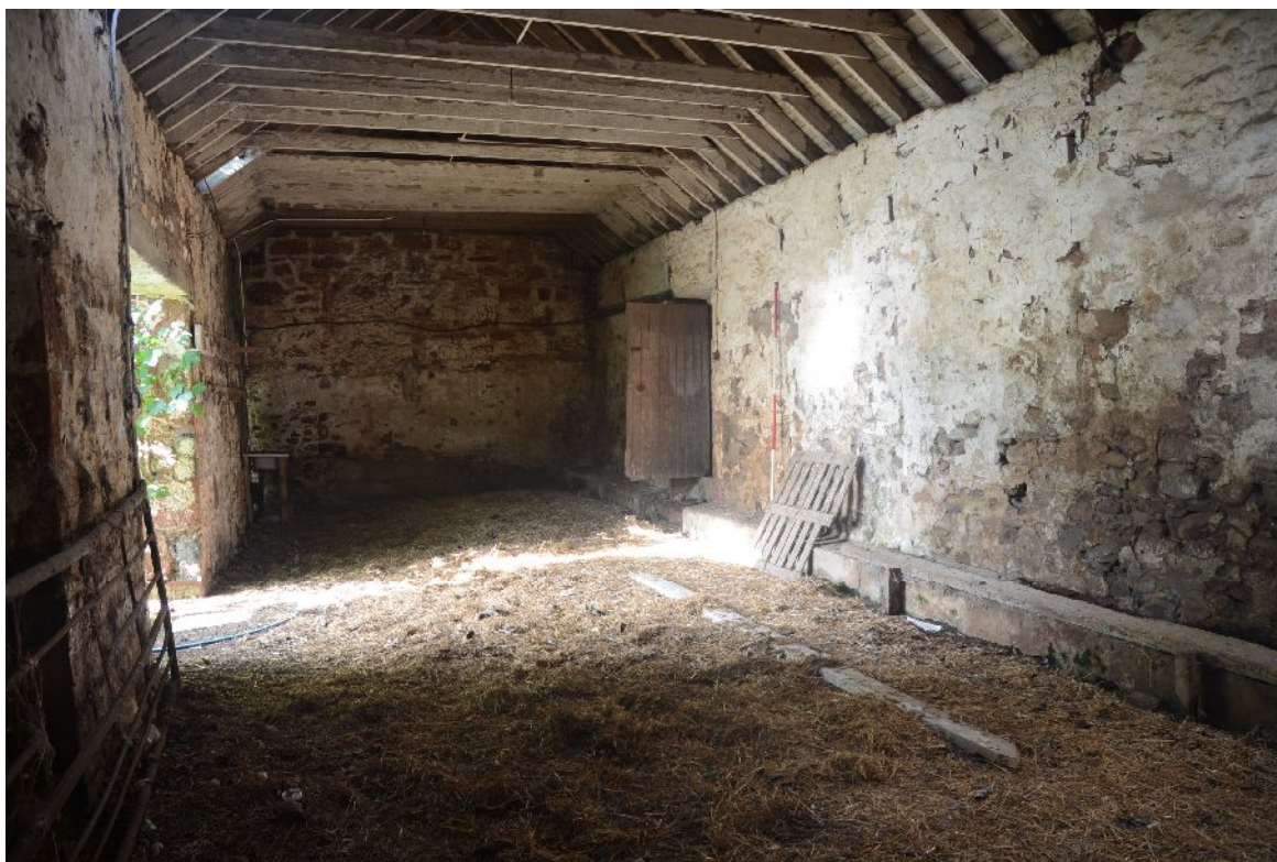
Illus 26 Building B looking N
