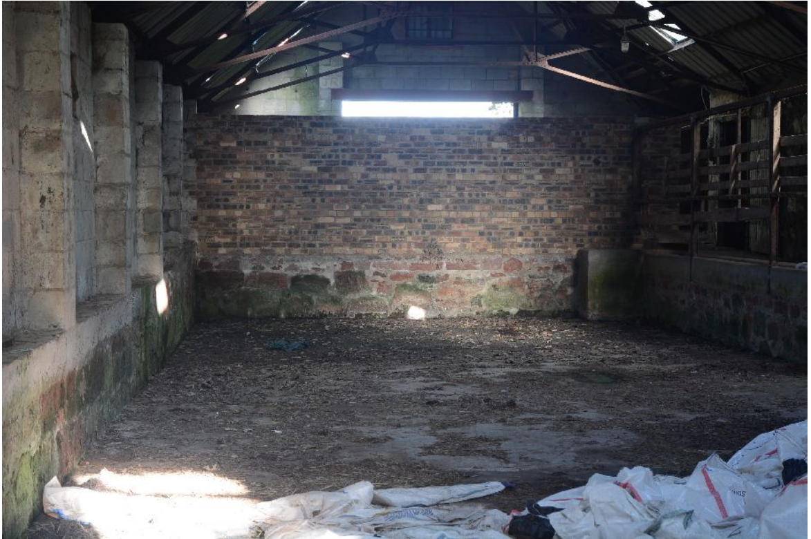
Illus 45 Building D interior looking E to partition, showing brick wall on sandstone base wall The SW corner was partitioned off and formed two tied cattle stalls.
