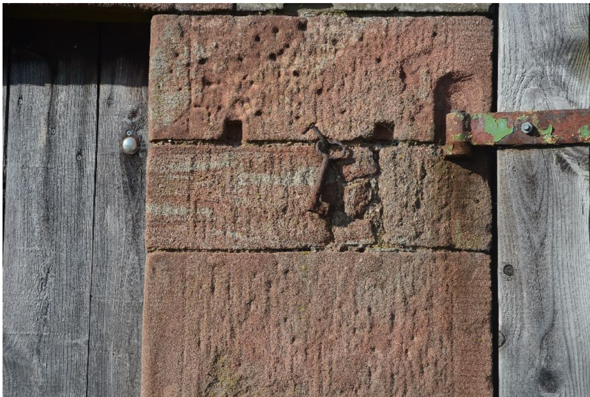
Illus 65 Building H . S wall. Key on nail beside door D29.
