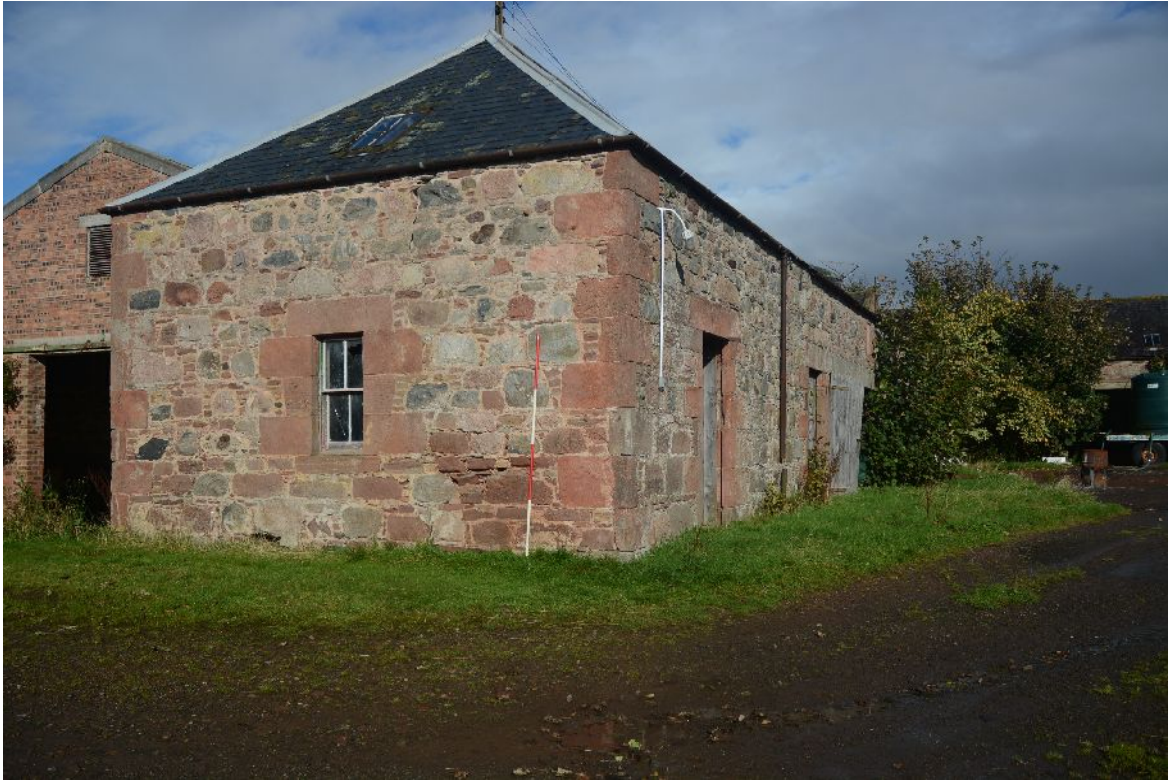
Illus 57 Building H. W wall.
