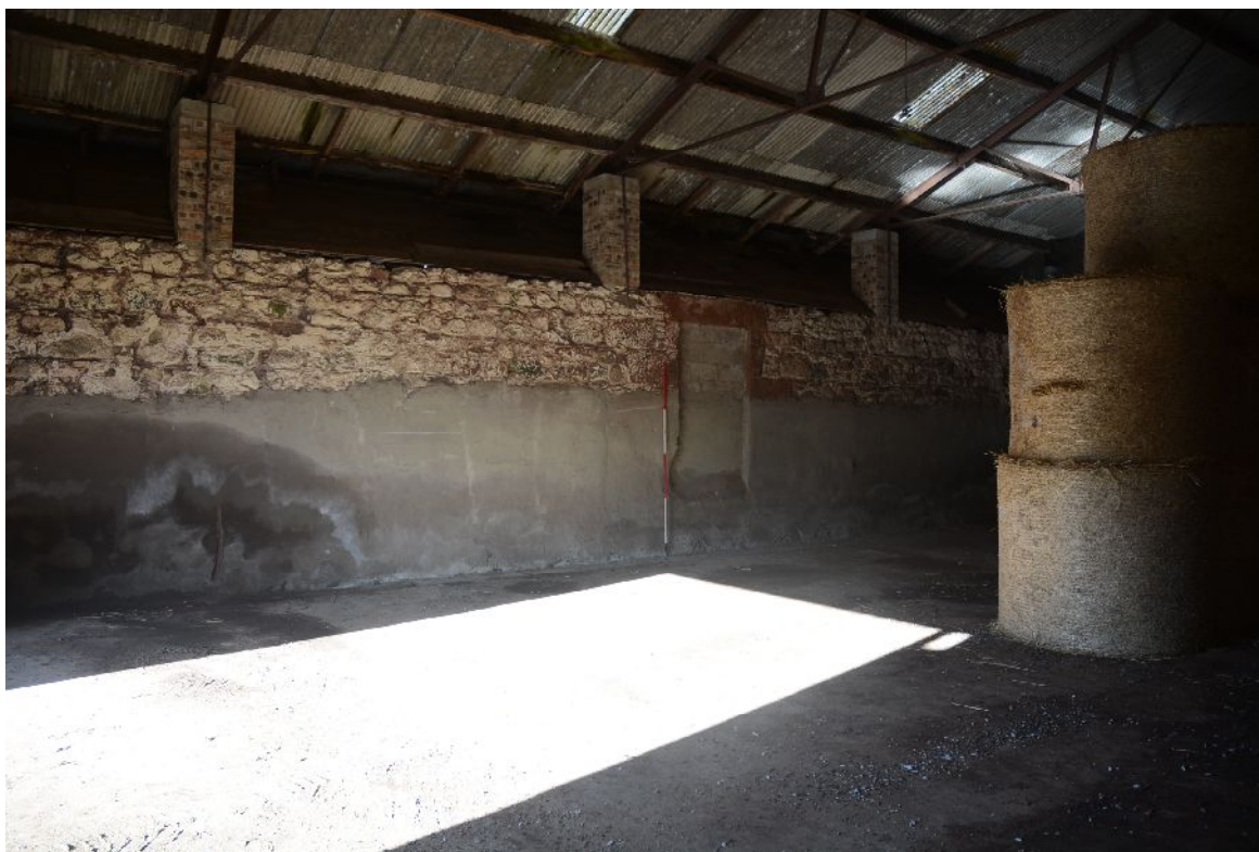
Illus 53 Building G. Interior looking NE. Door D24
