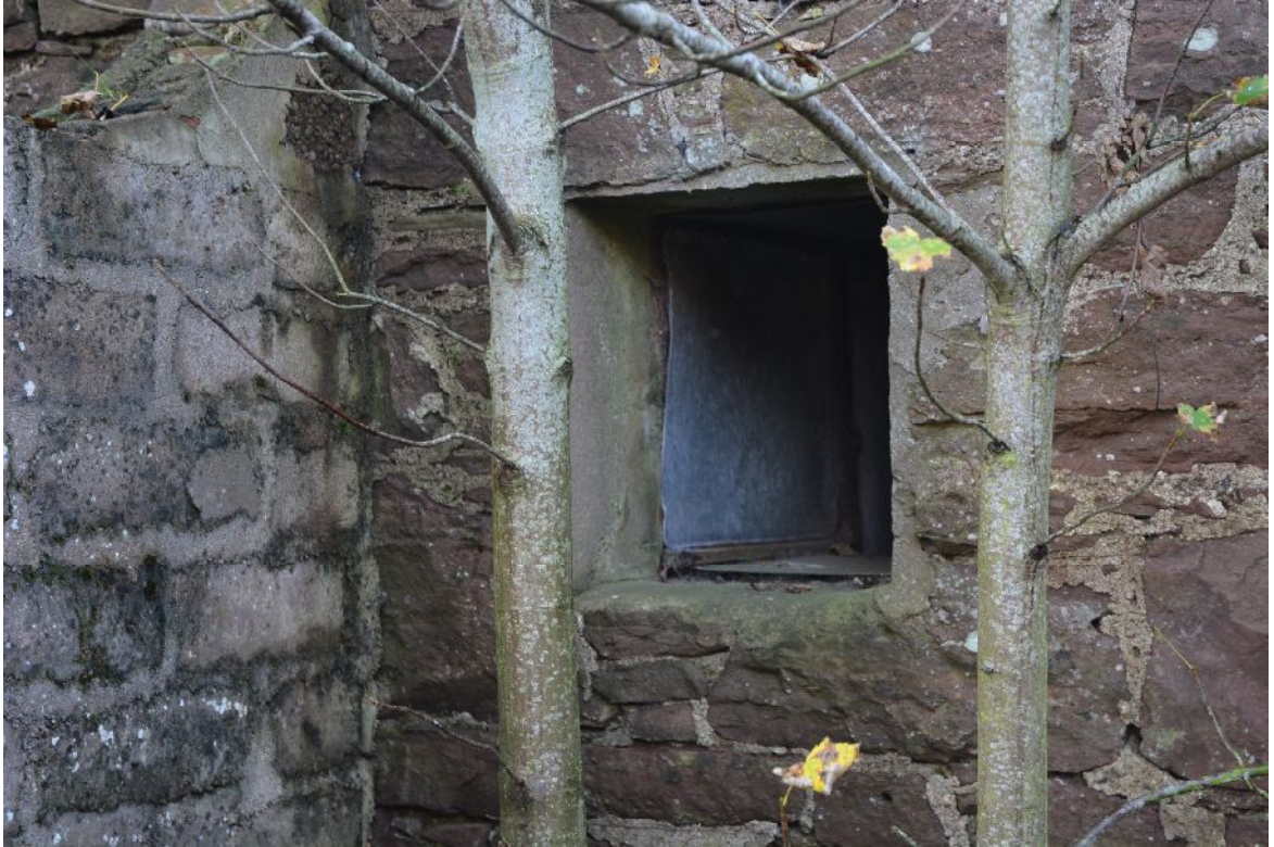
Illus 31 Building C, F5, grain chute
