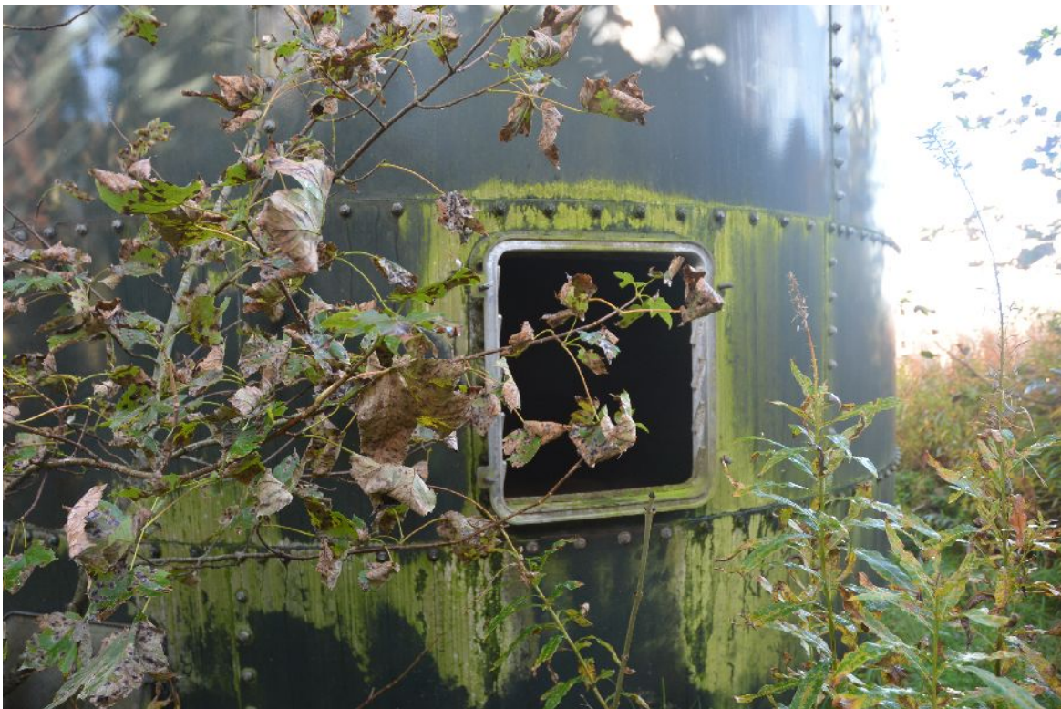
Illus 32 Hatch in grain tower opposite F5 chute opening
