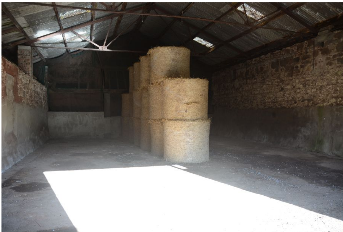
Illus 52 Building G. Interior looking E
