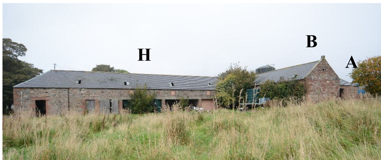
Illus 22 The steading from S, showing Buildings A, B and H
