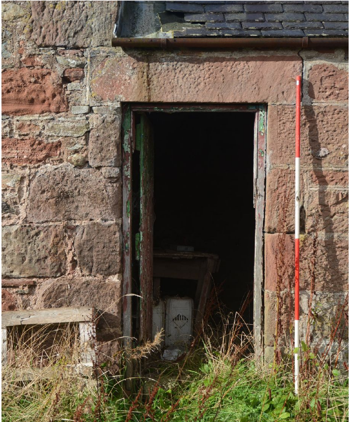
Illus 19 Building A, door D1
