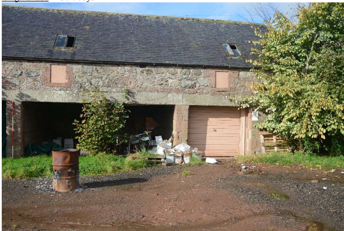
Illus 55 Building H. S wall detail of doors D32-D34
