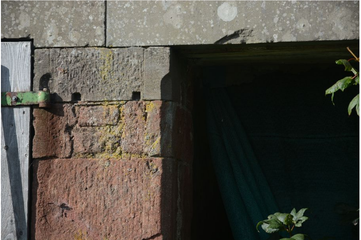
Illus 56 Detail of stonework between doors D29 and D30
