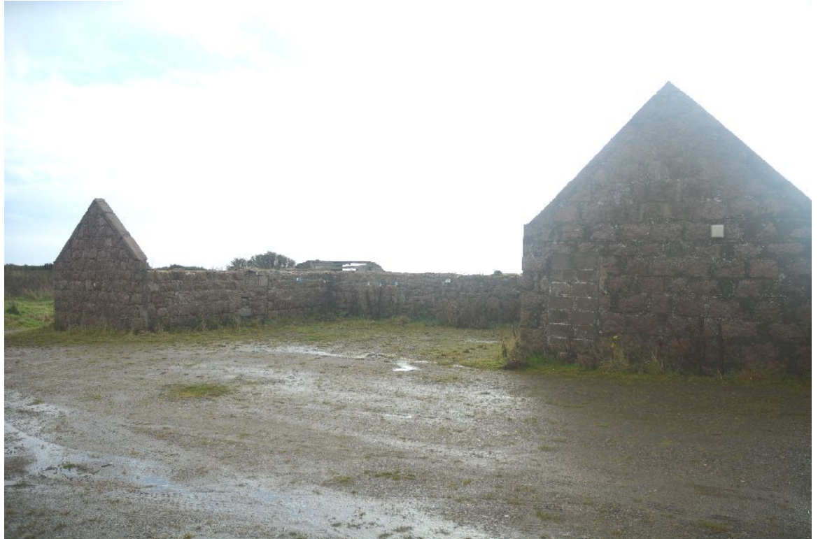
Illus 13 Building 2 (background LHS) with gable of Building 1 (RHS) looking SE
