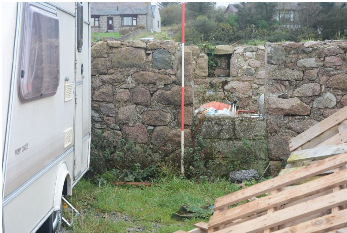
Illus 19 Building 2. Recess F5 seen through partly blocked door D3
