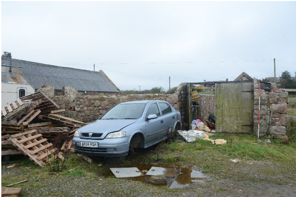
Illus 14 Building 2 S elevation
