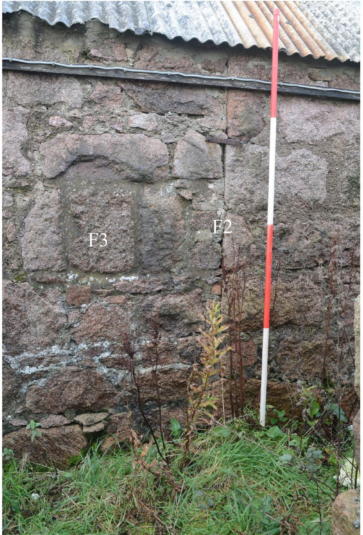
Illus 11 Building 1. E wall. F2 building line and F3 blocking. Ranging rod lies against original rybats.
