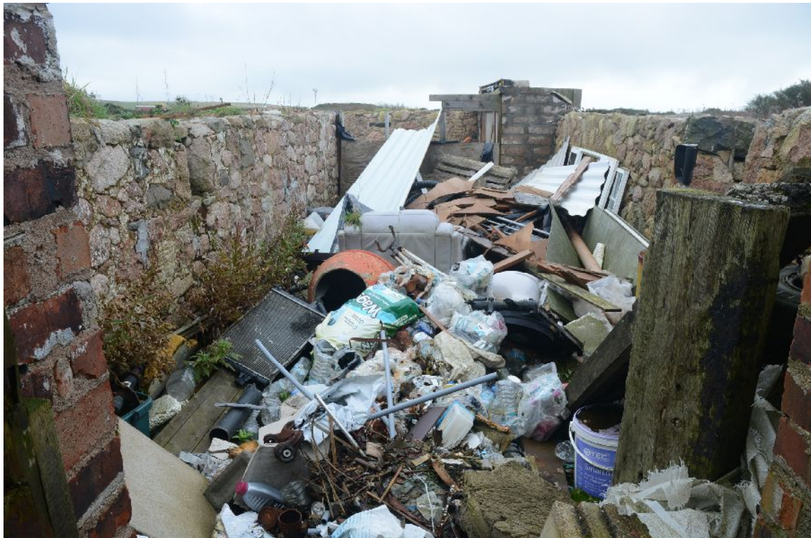
Illus 21 Building 2. Interior of W Range from door D4
