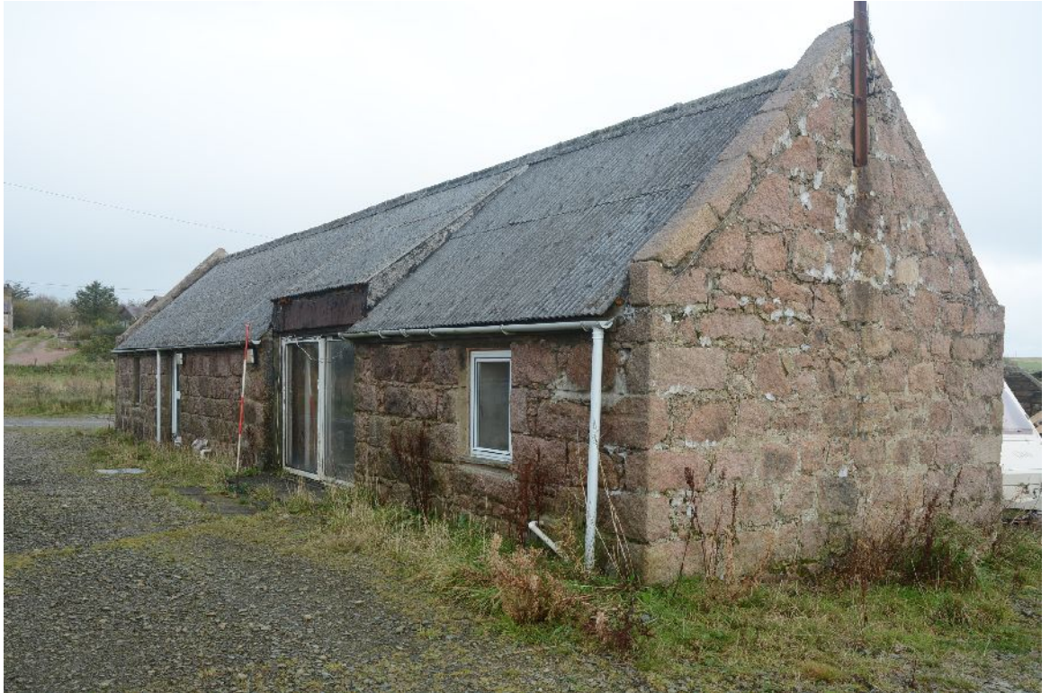
Illus 12 Looking N along W wall with modern windows and doors
