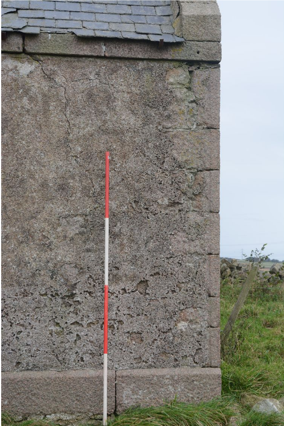
Illus 11 Farmhouse N end of front (E) wall showing ashlar basal course and raised margins on quoins.
