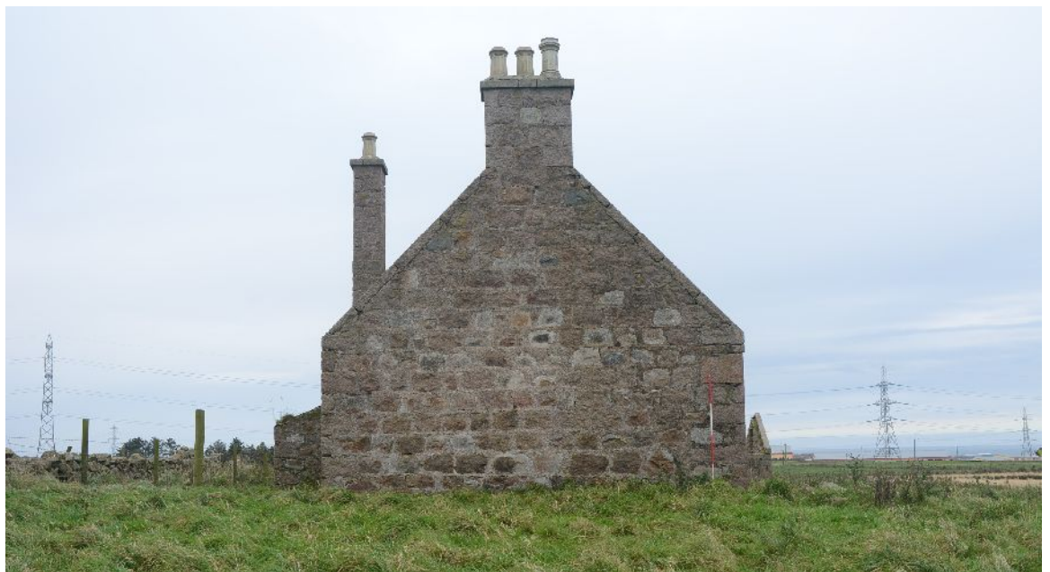
Illus 10 Farmhouse E gable, showing well coursed rubble.
