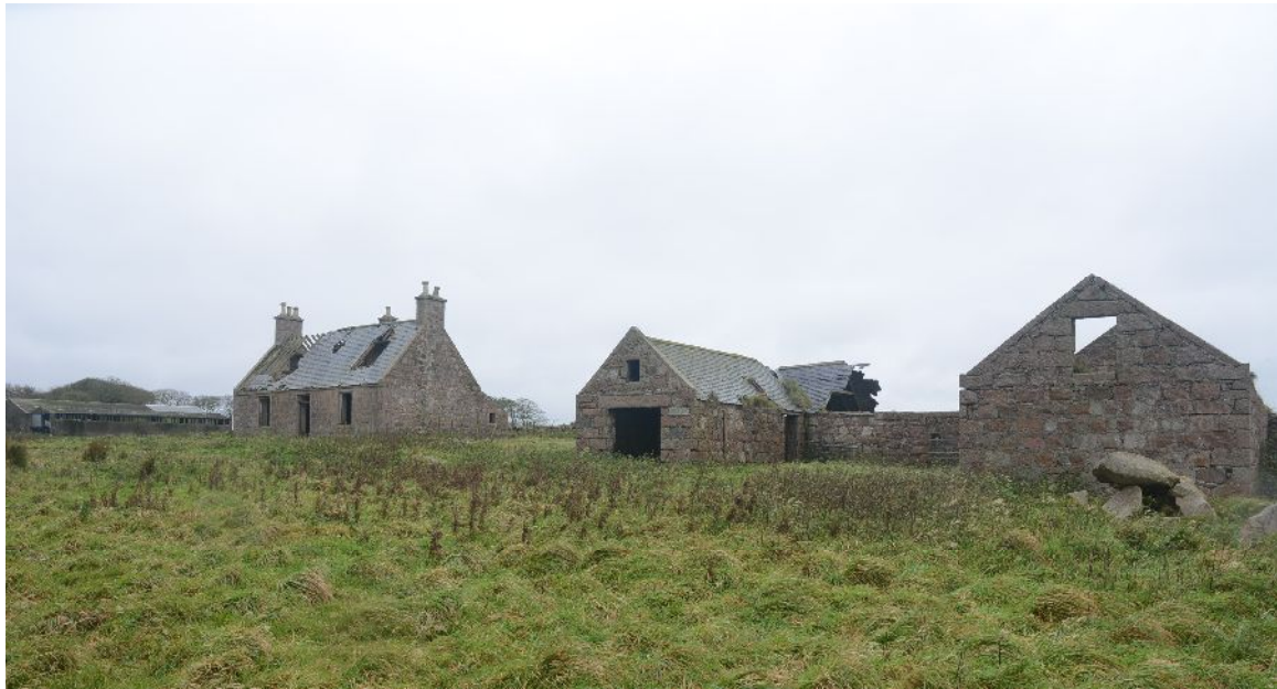
Illus 3 Cowhills, House (LHS) and Steading (RHS), looking SW
