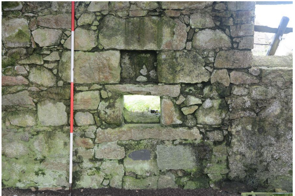
Illus 26 Mill shaft holes F1 and F2, window W1 to RHS
