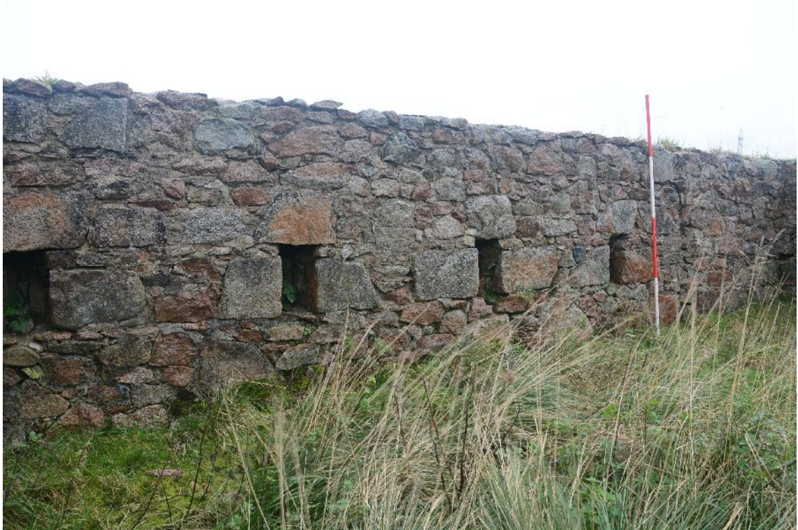
Illus 35 W Range- byre looking W. Detail of vents.
