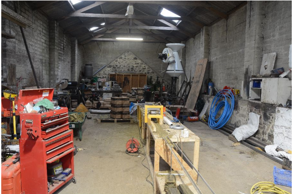
Illus 11 Looking S inside the upper floor of the central range of Building B. Note the original S gable of the loft, with walls raised with concrete blocks.
