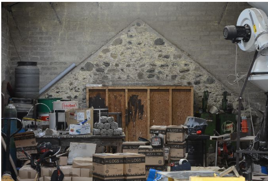
Illus 12 Detail of Building B original S gable of loft
