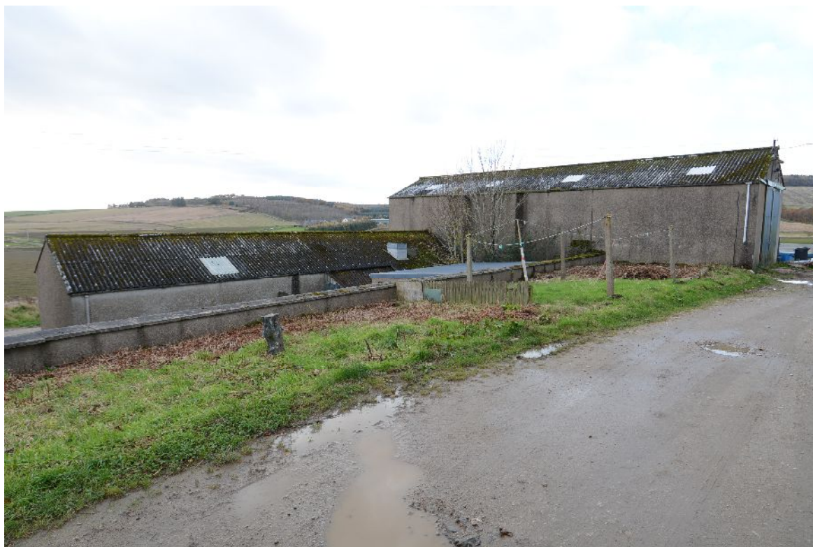
Illus 10 N elevation of Building B looking W
