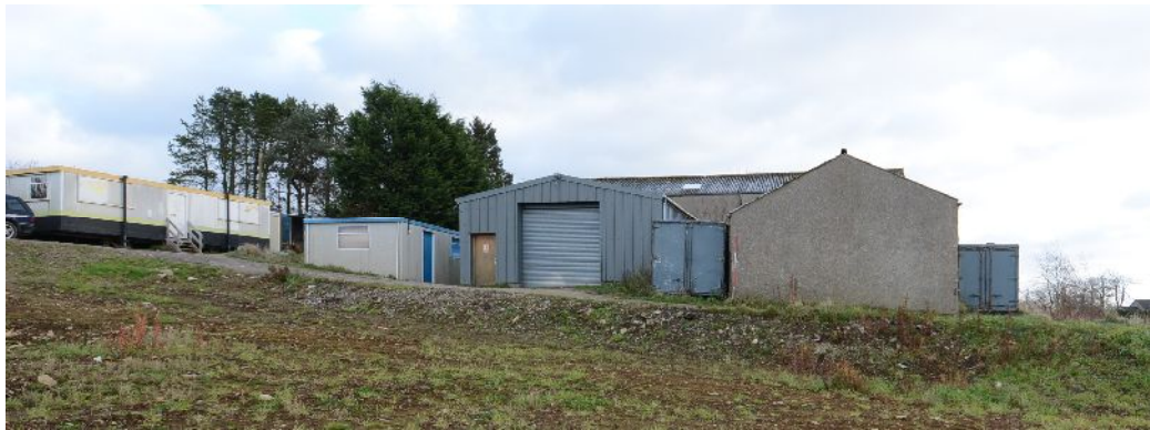
Illus 6 General view looking E showing modern sheds etc (G,F,E,D) and W gable of Building B (west)
