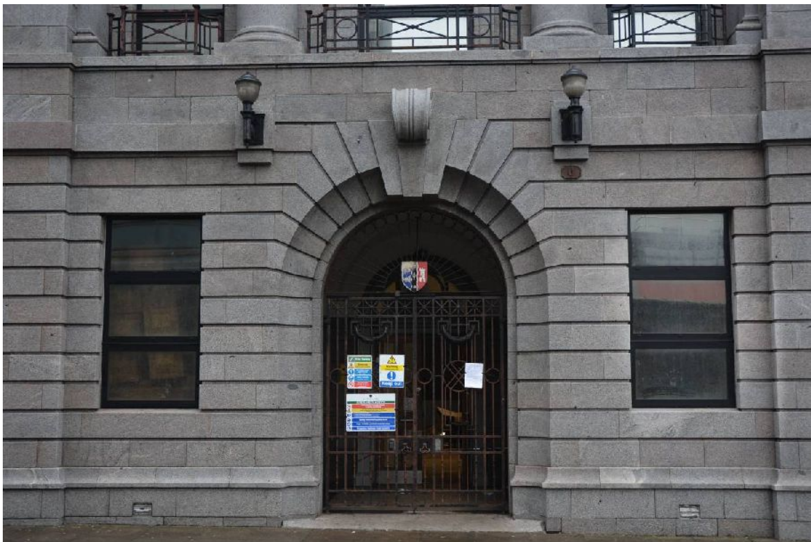
Illus 22 Detail of the St Andrew Street entrance
