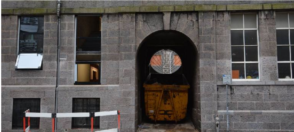
Illus 38 NW entrance from John Street from street (photo 56)
