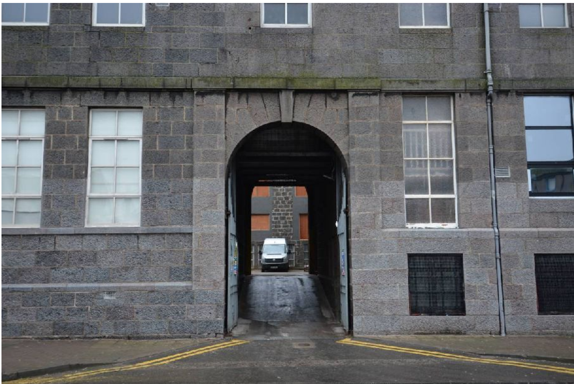
Illus 37 SW entrance from John Street from street (photo 51)
