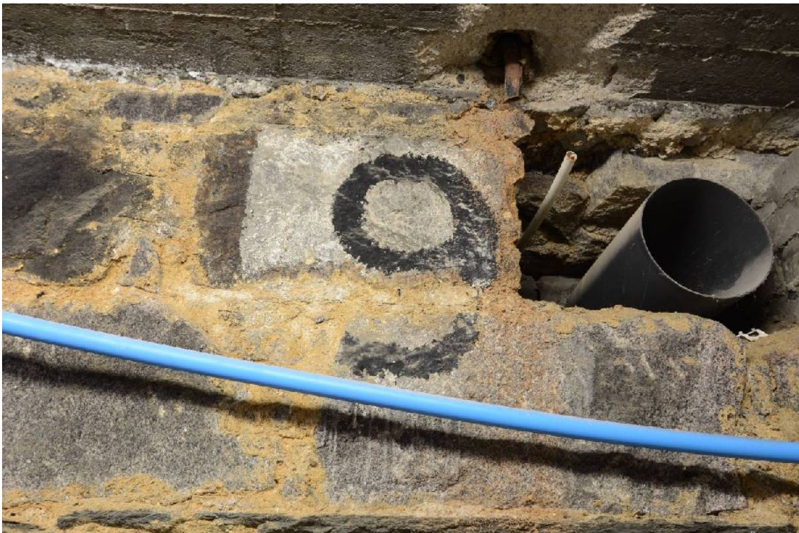
Illus 49 Muster point number on basement wall (photo 45)
