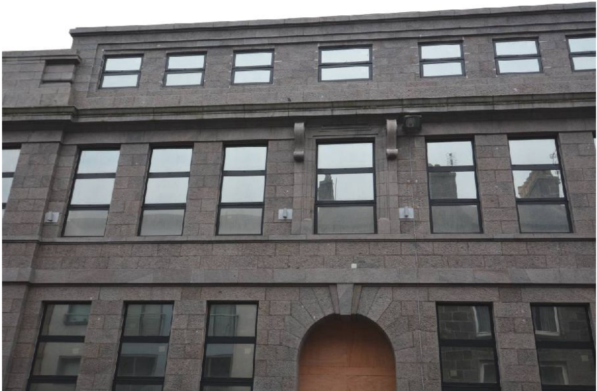
Illus 30 Charlotte Street entrance with window above. Note the windows on the top floor are new insertions. (photo 63)
