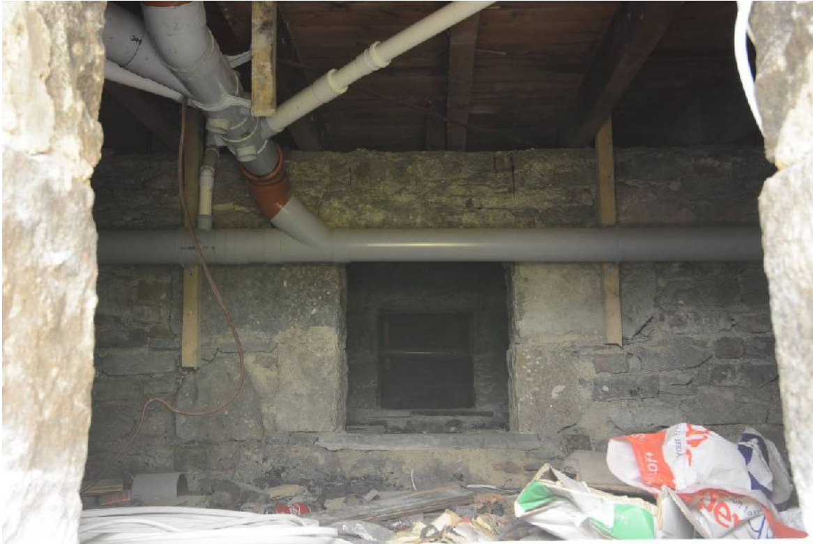
Illus 46 Looking through opening into service voids (photo 44)
