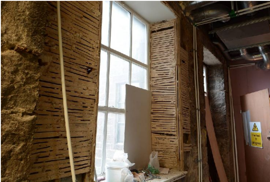
Illus 13 Lathe and plaster surviving beside window (photo 22)
