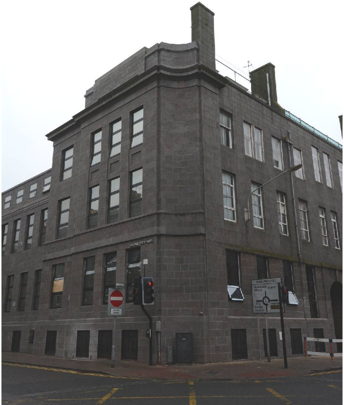
Illus 10 John Street/Charlotte Street corner showing concave corner stonework (photo 58)
