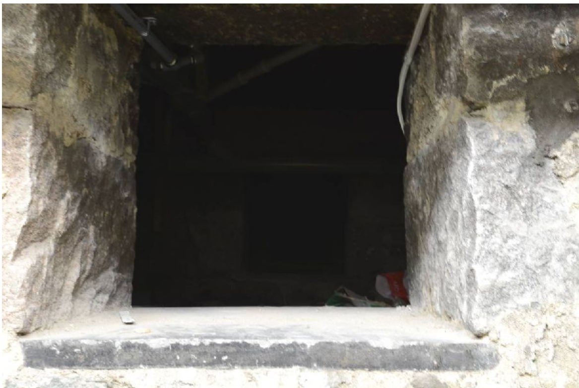
Illus 45 Opening between basement passage and service void (photo 43)
