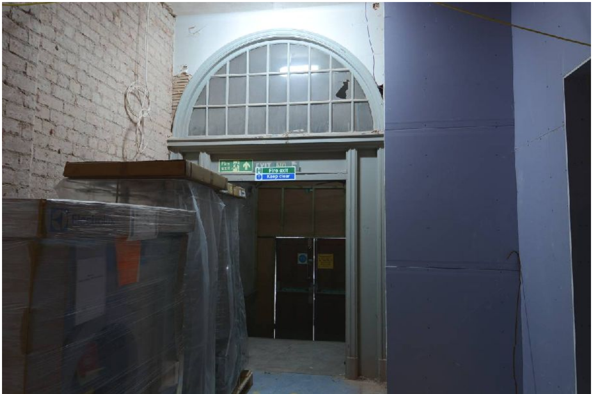
Illus 31 Charlotte Street entrance from inside (photo 25)
