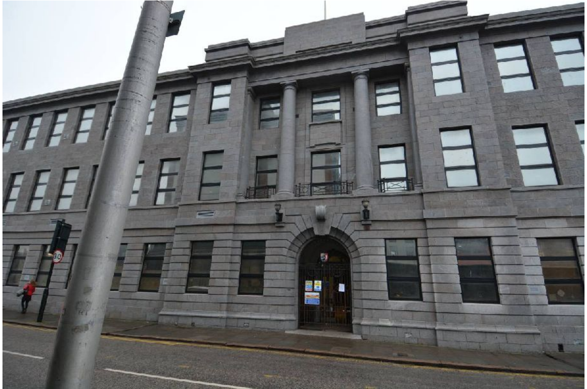
Illus 21 The St Andrew Street entrance.
