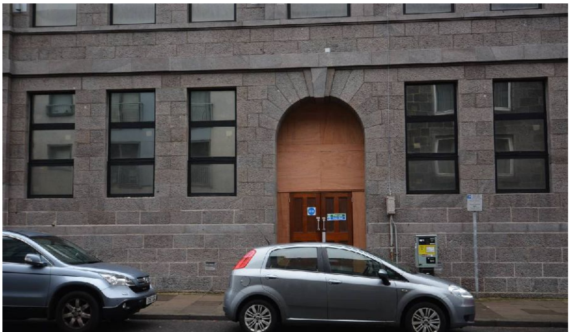
Illus 29 Charlotte Street entrance at ground level (photo 62)
