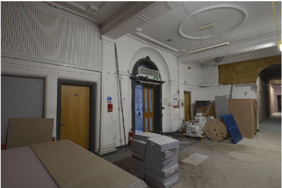
Illus 25 Entrance hall inside the St Andrew Street entrance
