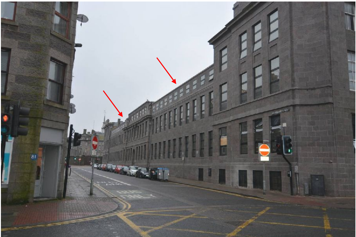
Illus 63 Charlotte Street roof garden (red arrows), now roofed and with windows replacing railings
