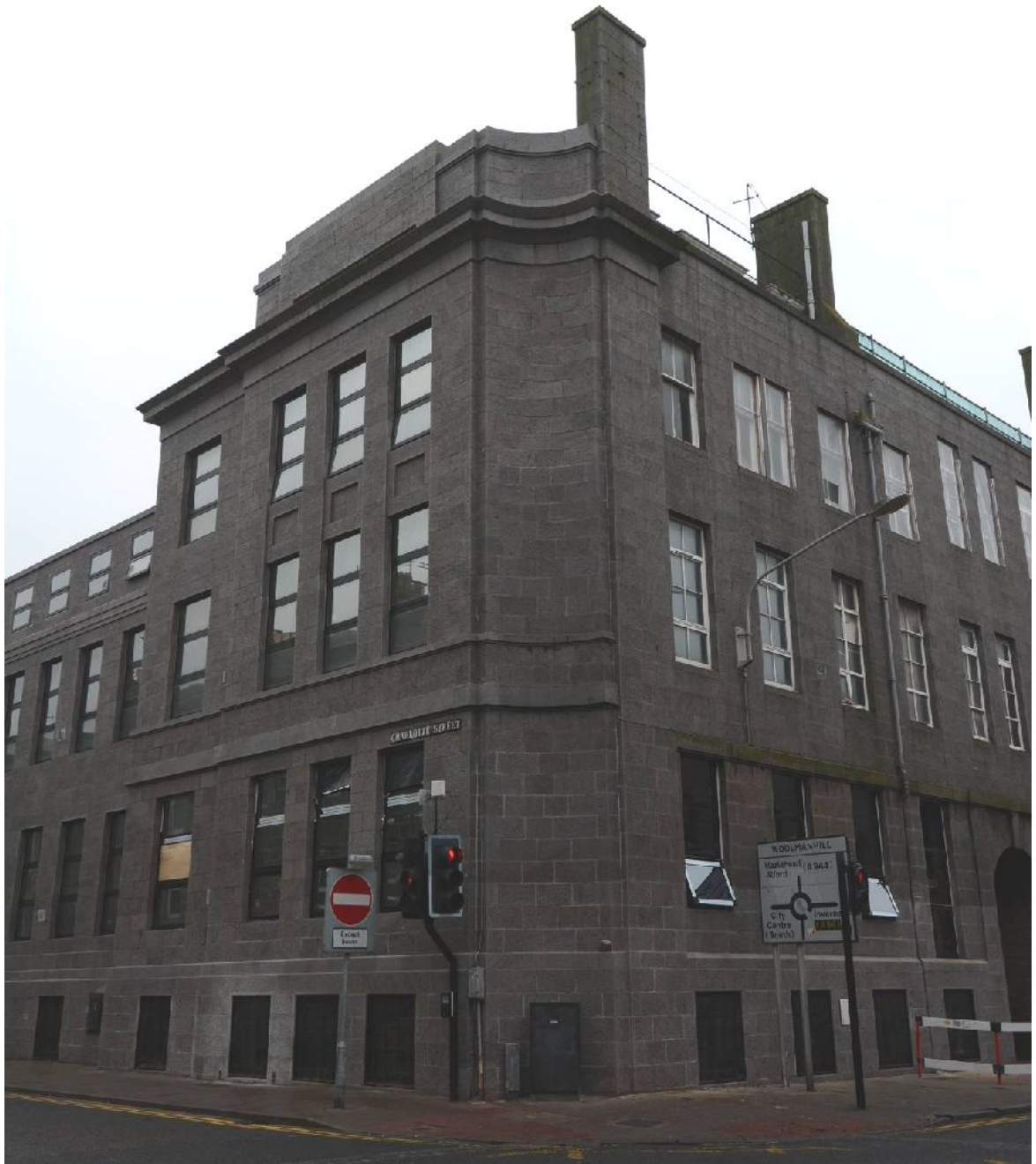
Illus 15 New windows on Charlotte Street (LHS) and original windows on upper floor on John Street facade (RHS) (photo 58)
