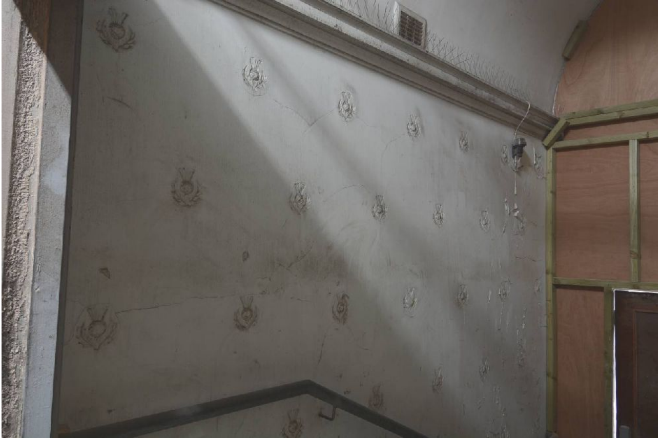
Illus 32 Charlotte Street entrance from inside (photo 27). Plasterwork in lobby.
