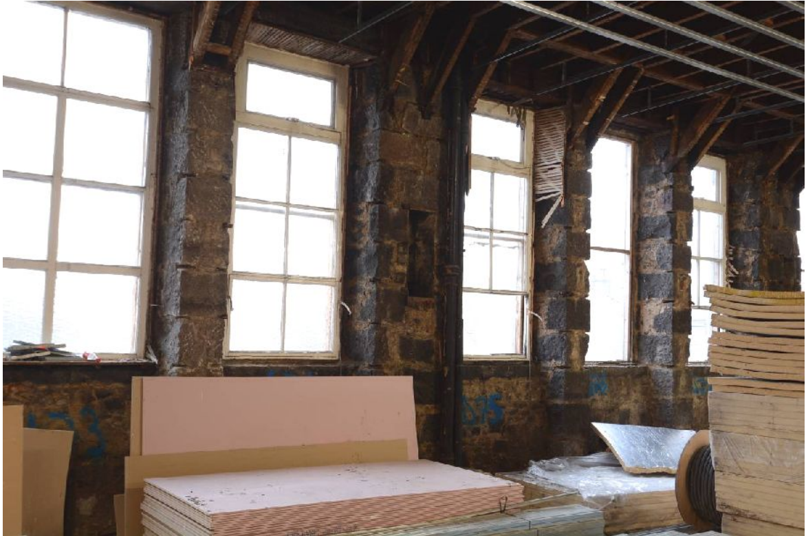
Illus 59 Inner face of wall on John Street facade (photo 8)
