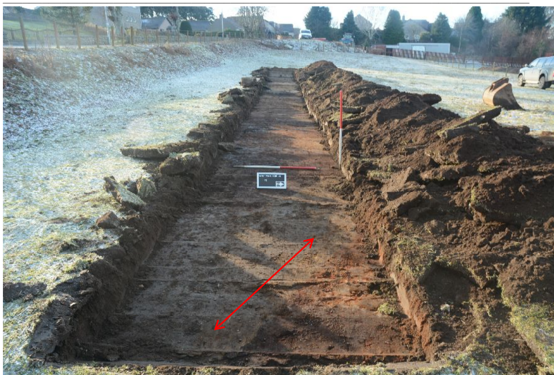
Illus 10 Trench 3 looking W. Service trench (context 5) marked by red arrow
