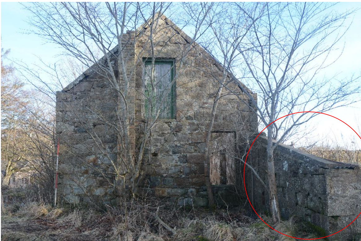
Illus 16 W gable of the N range and NW corner of the court wall with indication of low lean-to roof (inside red circle).
