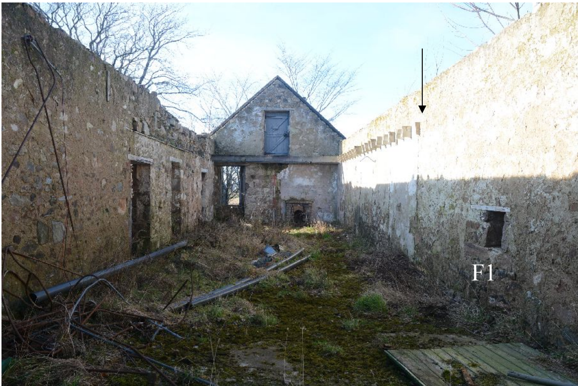
Illus 10 N Range, interior looking W. Arrow shows E limit of loft. F1= horsemill shaft hole.
