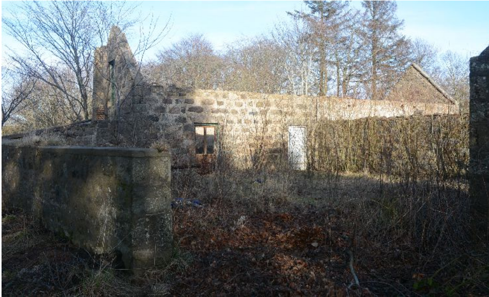
Illus 15 Opening into the court. The coping is visible on the nearest section of the W wall.
