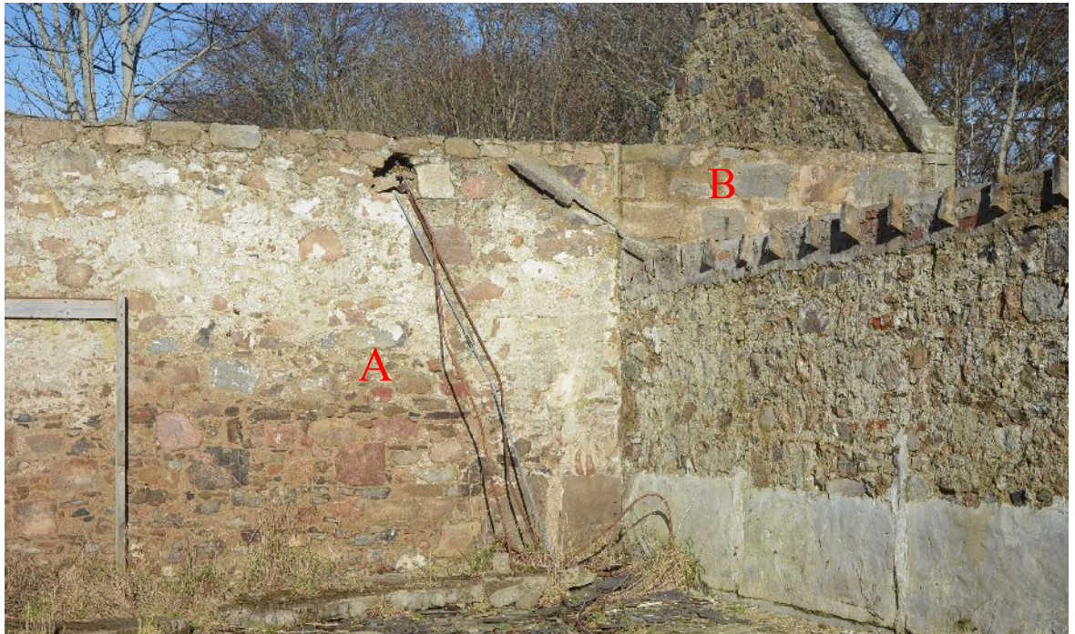
Illus 6 Looking N inside the E range. Note the difference in stonework inside (A) and outside in the E facade (B).
