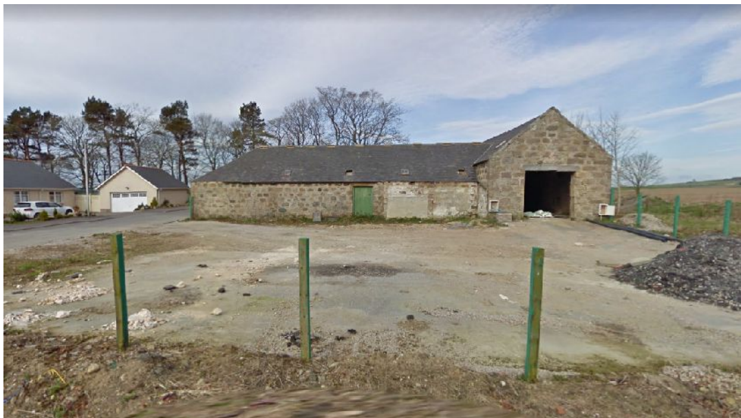
Illus 7 Roofs in 2011 as shown on Google Street View. Copyright www.google.co.uk
