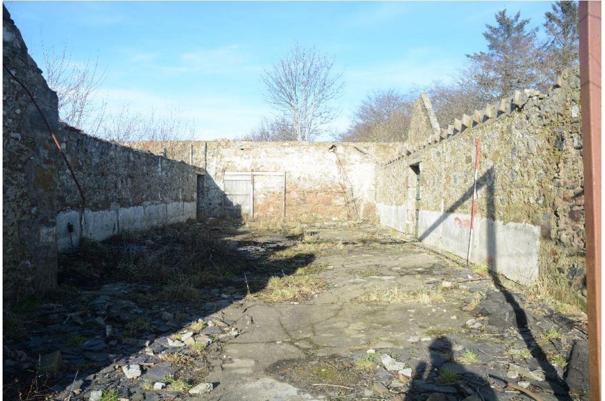
Illus 13 E Range. Interior looking N
