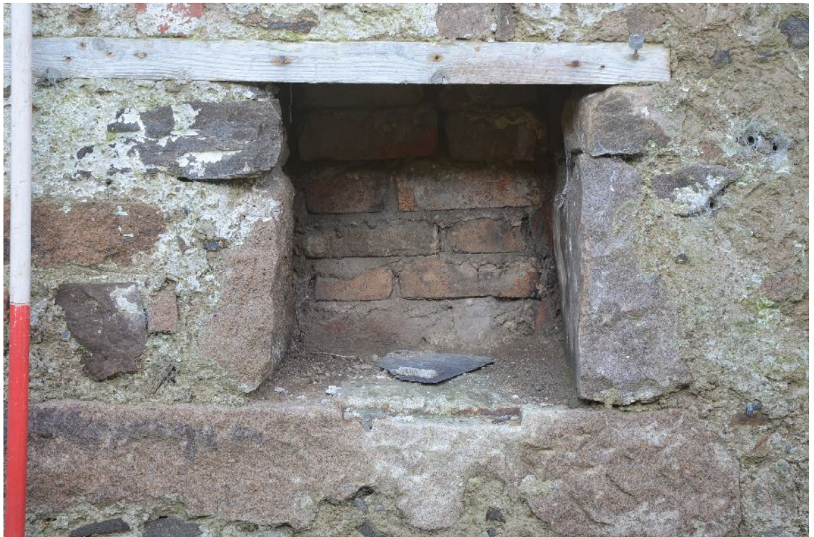
Illus 11 Detail of blocked shaft hole F1
