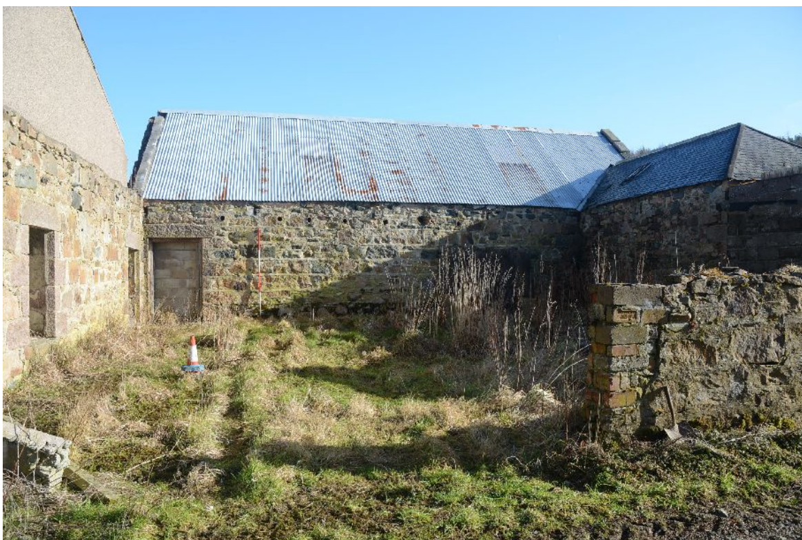
Illus 10 General view of steading looking W into Court
