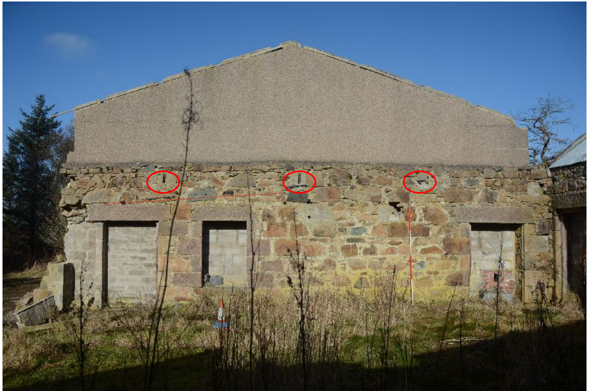
Illus 19 S face of the N wall of the Dung Court with the gable of the secondary N building built on it. The red circles mark timber slots associated with a roofing of the Court. The dotted line below them appeared to be tar or felt, presumably also associated with the Court roof.
