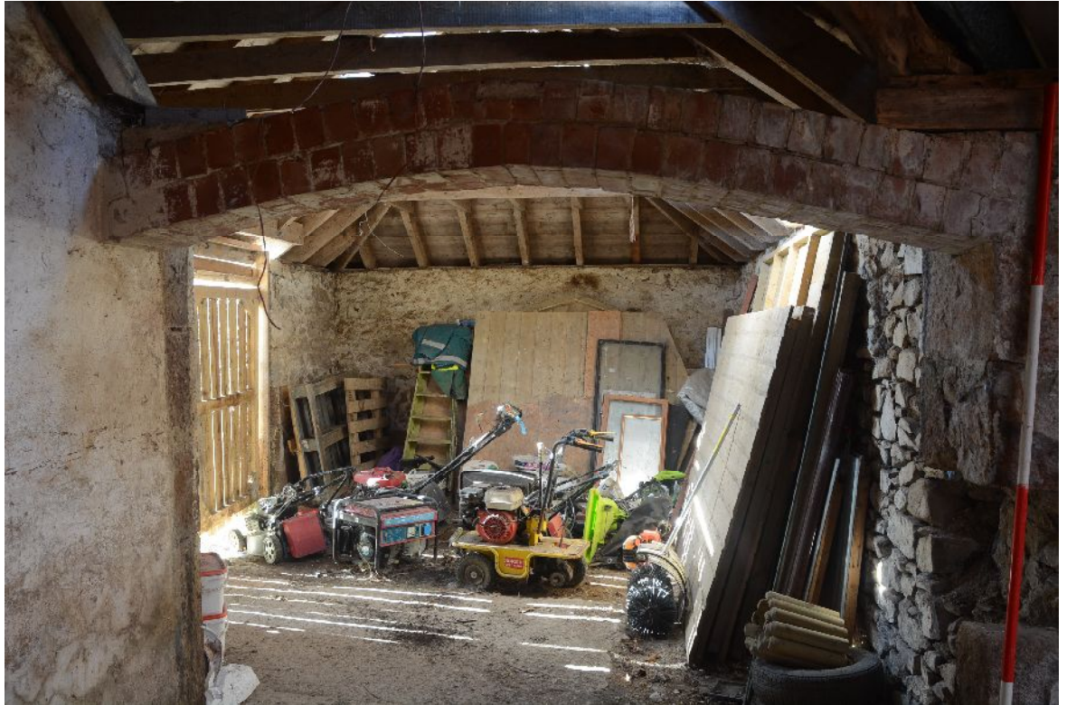
Illus 18 Looking into Building A through brick arch F4
