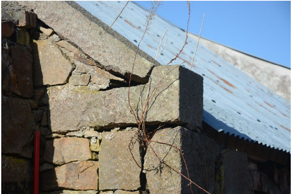
Illus 12 Granite skeuputt at SE corner of East Range.
