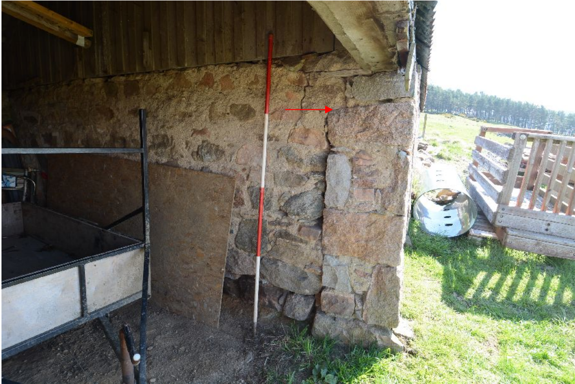
Illus 11 E side of door D4, showing column between D4 and D5. Arrow shows change in stonework at top of wall
