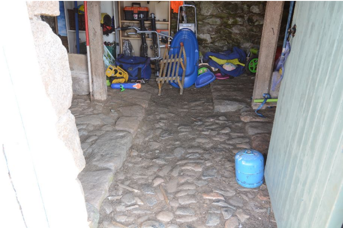
Illus 16 Interior of C showing central drain in cobbled floor.
