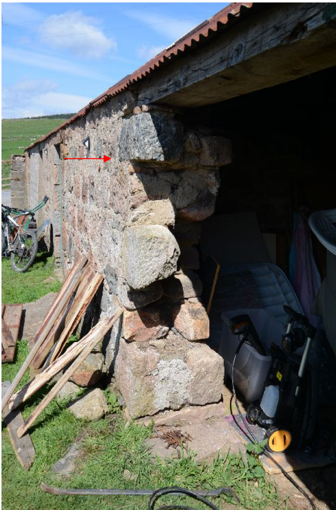
Illus 10 W side of door D4. Arrow shows change in stonework at top of wall
