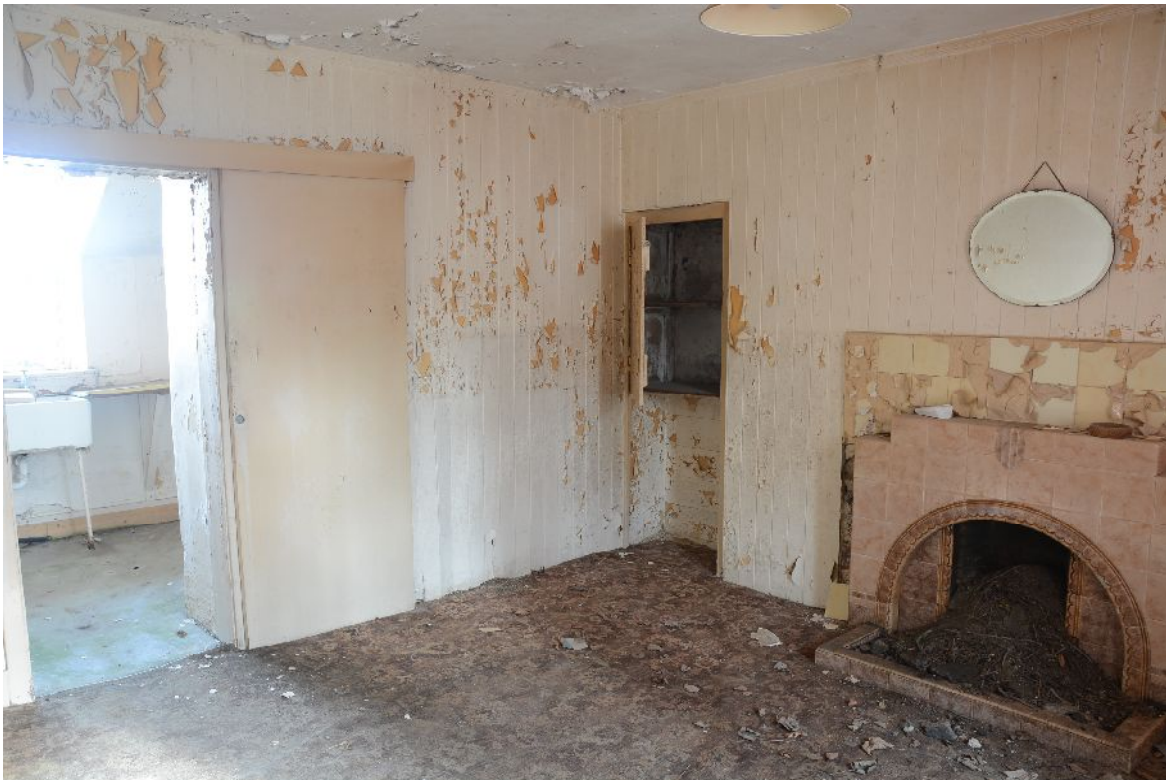
Illus 16 Ground floor. E room/ living room, looking through to kitchen
