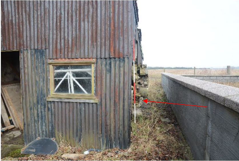
Illus 15 Wash-house from S with arrow indicating stone flue for boiler
