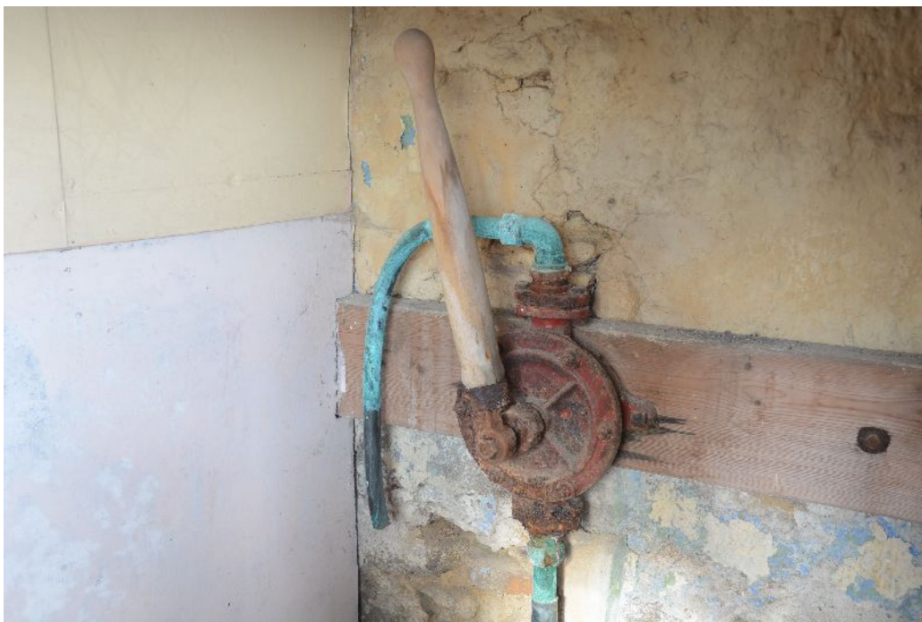
Illus 9 Pump behind door in NW corner of porch
