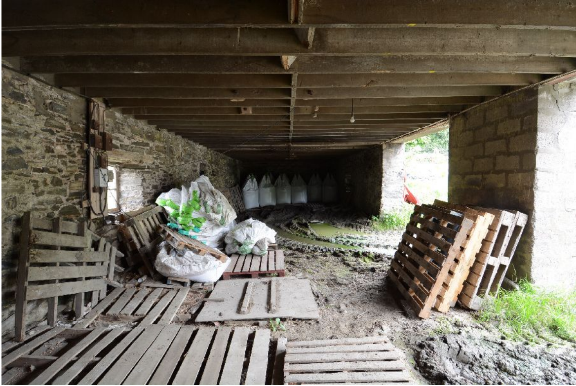
Illus 13 Interior at ground level looking N
