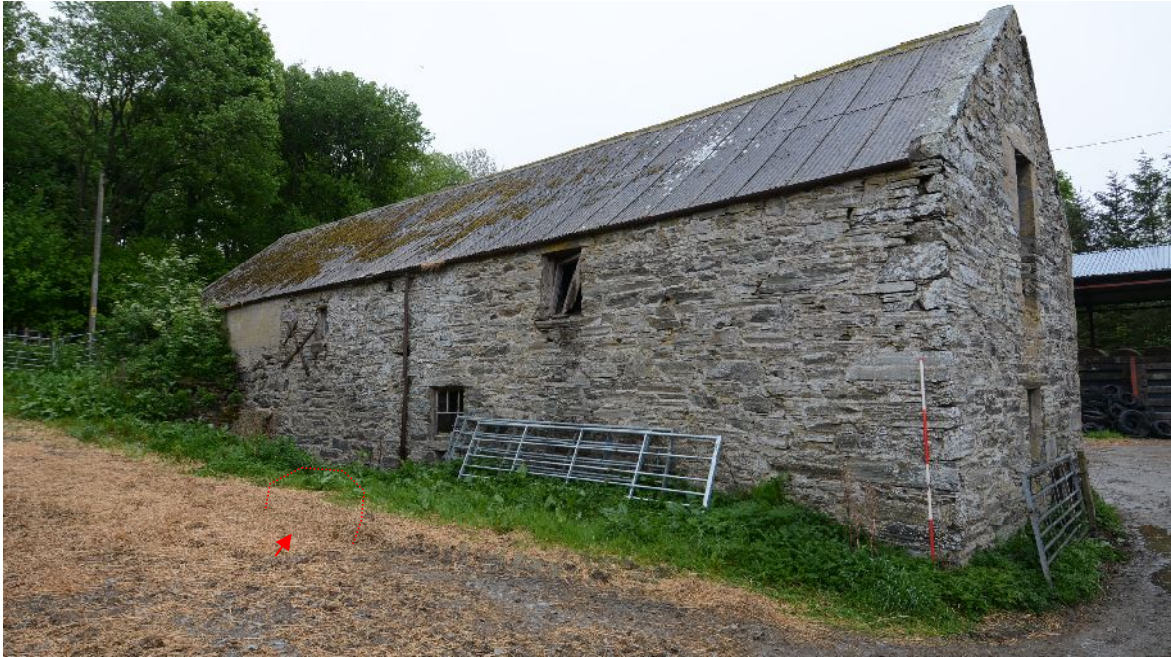
Illus 8 W elevation looking N. Dotted line indicates the approximate position of the water wheel, just visible in the differential weathering of the stone. The arrow indicates F1, the blocked axle hole.
