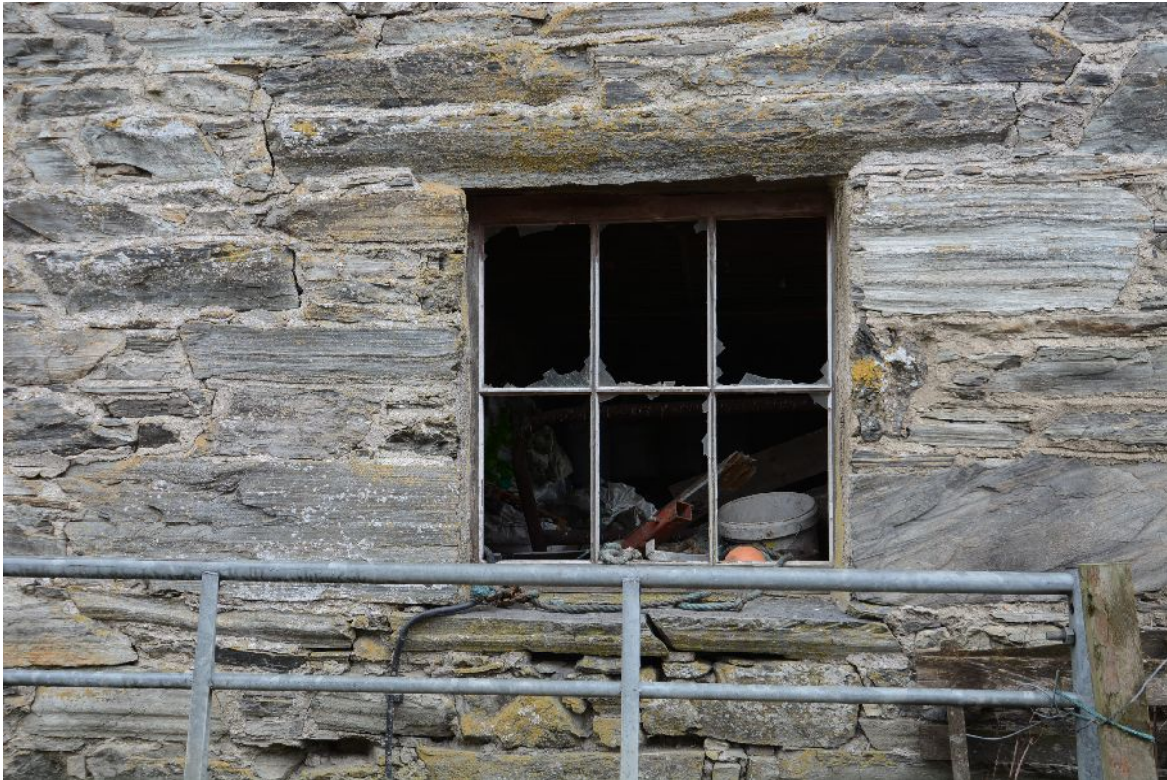
Illus 7 S wall and window W5 showing detail of stonework
