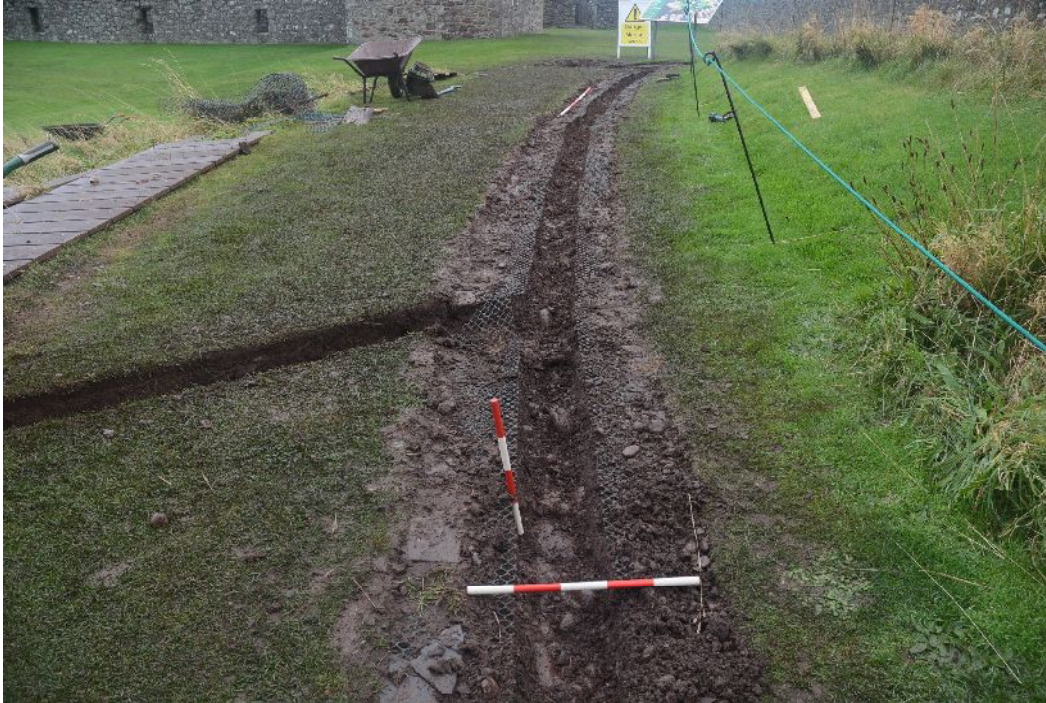
Illus 6 The walkway looking E after excavation.
