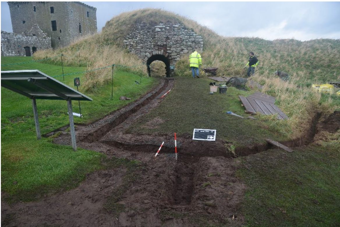
Illus 8 Looking W to pend showing side drains
