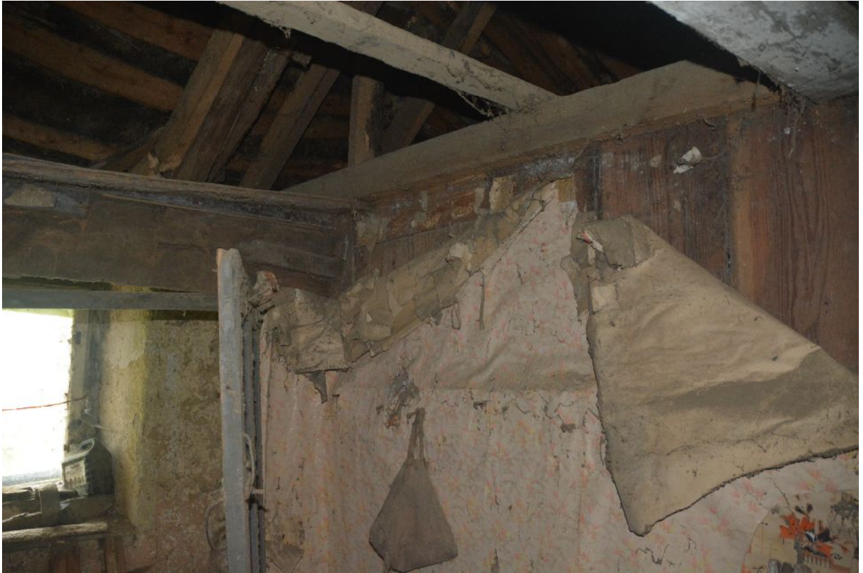
Illus 12 Inside room 2 looking towards passage and W2, showing wallpaper on internal wooden partition wall.
