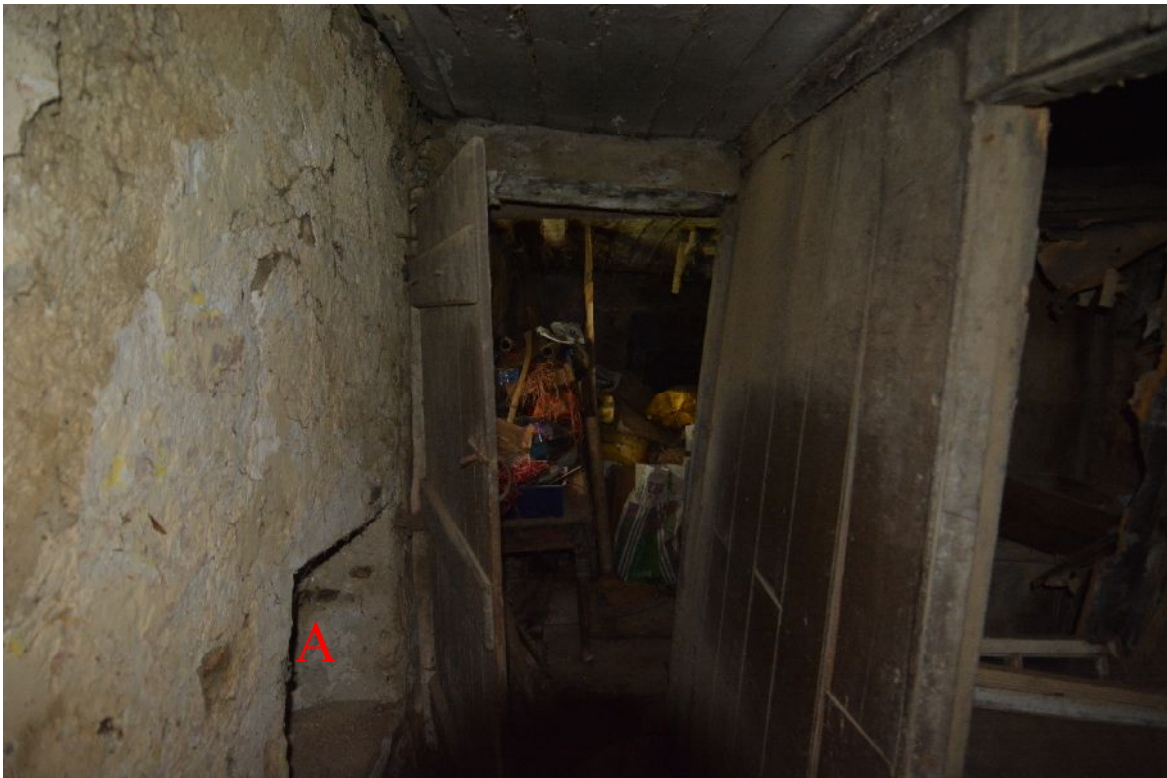
Illus 27 Passage, looking towards kitchen showing alcove on inner face of the front wall (A). Room 1 on RHS
