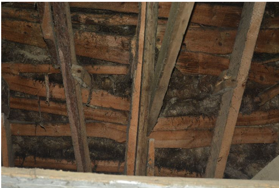
Illus 13 Underside of roof from within cottage
