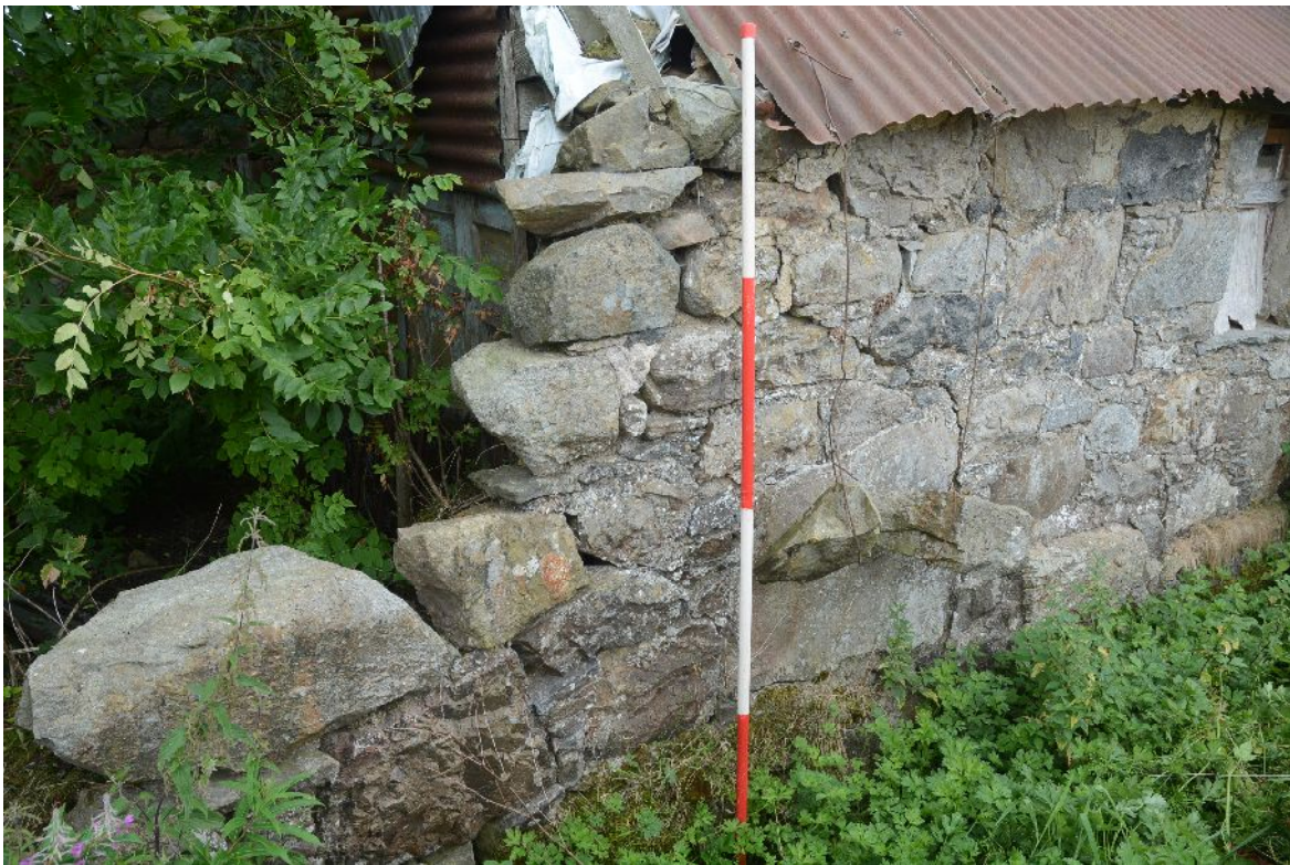
Illus 8 N wall. Junction between main cottage and E end.
