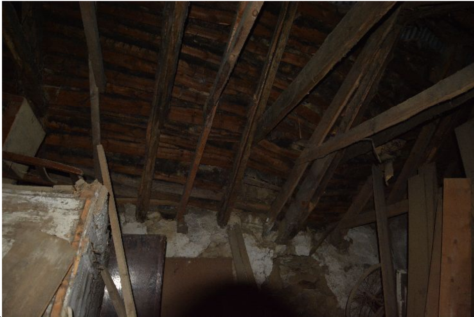
Illus 15 Roof structure in Room 1
