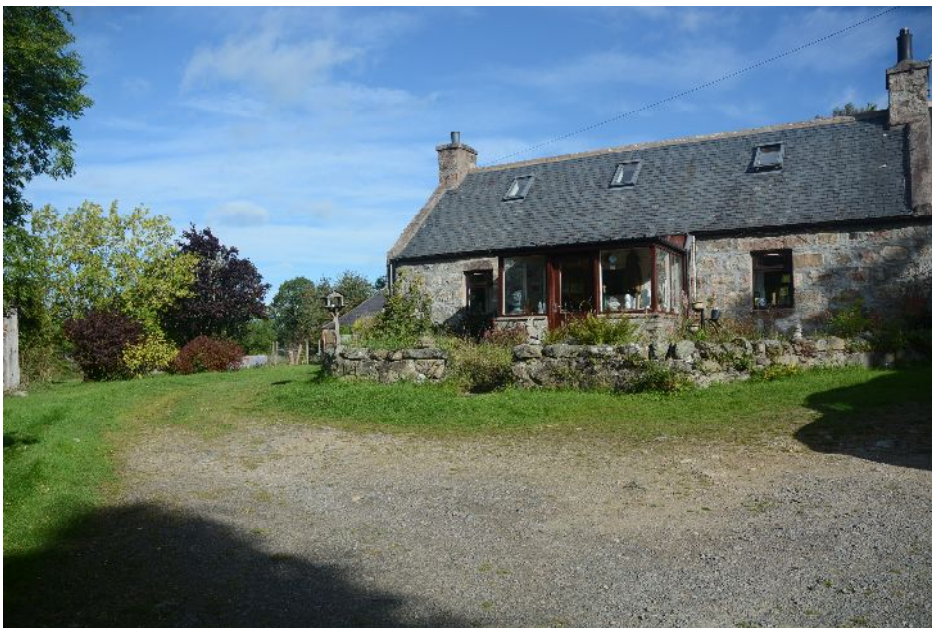
Illus 5 The croft house. The harled extension does not show in the photograph.
