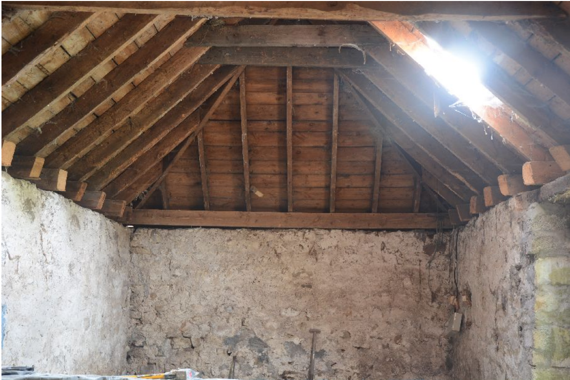
Illus 13 Interior of roof at E end showing sawn off cross braces
