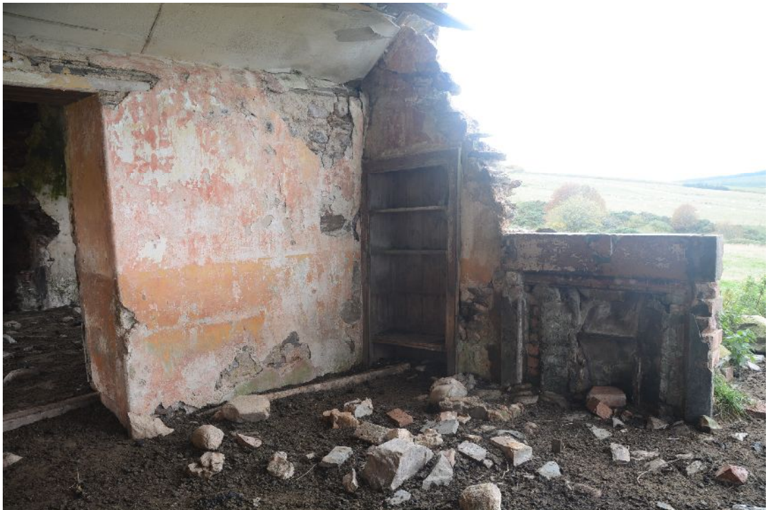
Illus 19 Room 2 looking W
