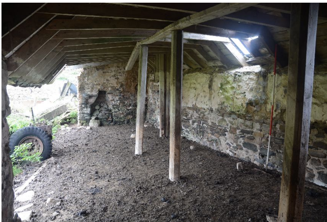
Illus 13 Building C looking S. Fireplace visible on back gable. Trevis hind posts along centre line in foreground
