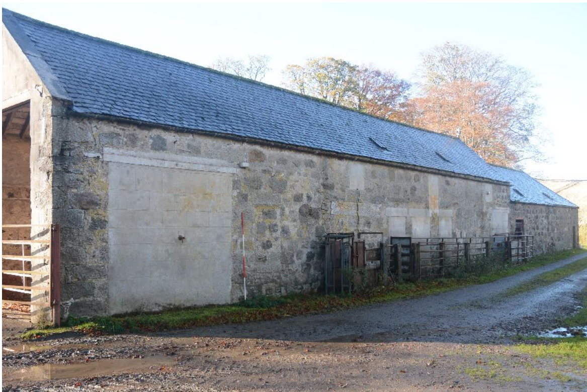
Illus 30 Building 1. NE elevation looking W
