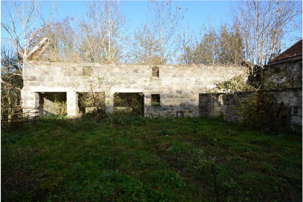
Illus 41 SW Elevation of mill seen from court
