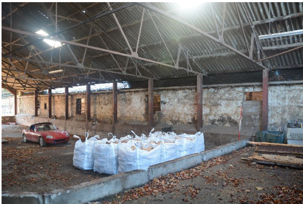
Illus 33 Looking S along NE wall of Area A, seen from central court
