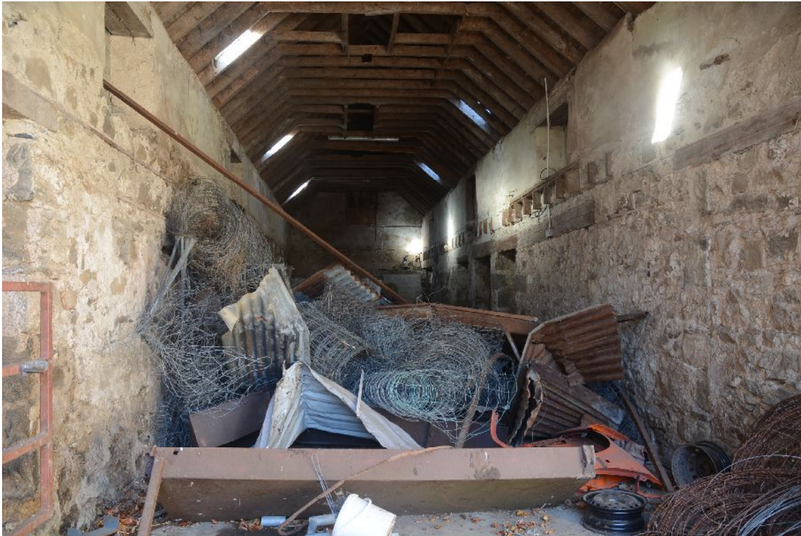
Illus 37 Interior of Area D looking NW. Note sawn off joists of loft floor
