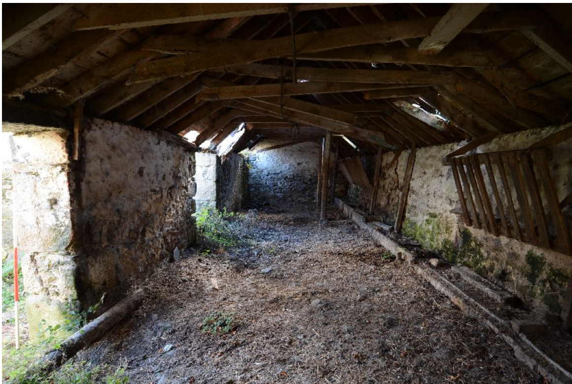
Illus 47 Interior of Building E looking SW
