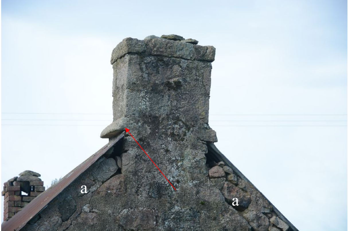
Illus 7 E Chimney with thatch protection (red arrow) and infill stonework (a)
