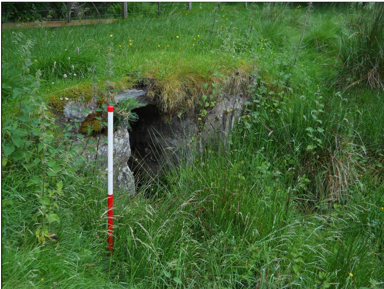
Plate 2 – Bridge Site 4 carrying access track Site 5
