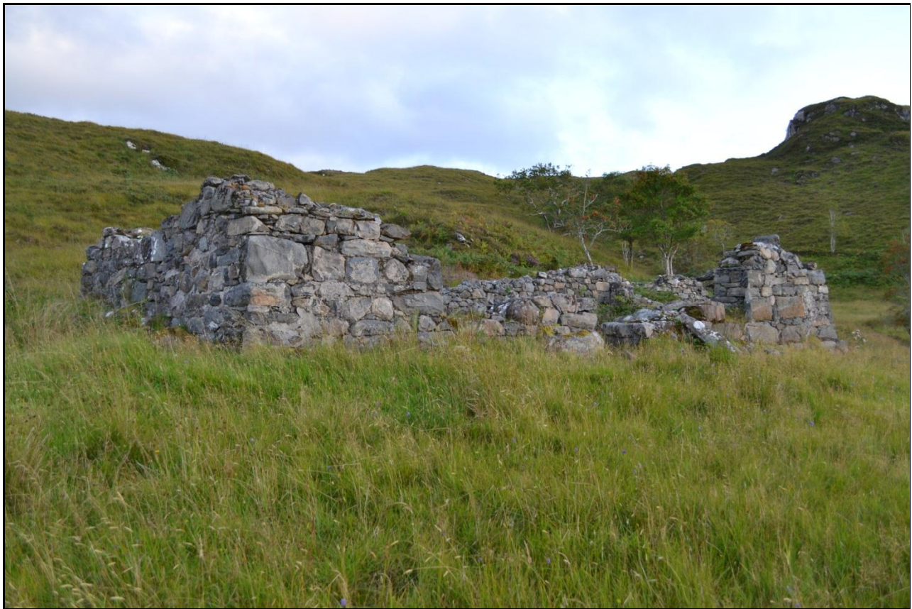
Plate 4 – Stone-built house with mortared wall joints Site 16, Airor Township
