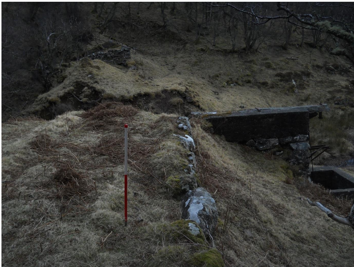
Plate 3 6 Top of the dam Site 16c and sluice housing Site 16b (to the right)
