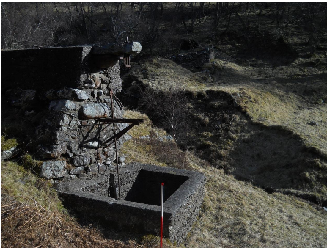
Plate 4 6 Sluice-gate housing Site 16b and the tiered back edge of the dam Site 16c
