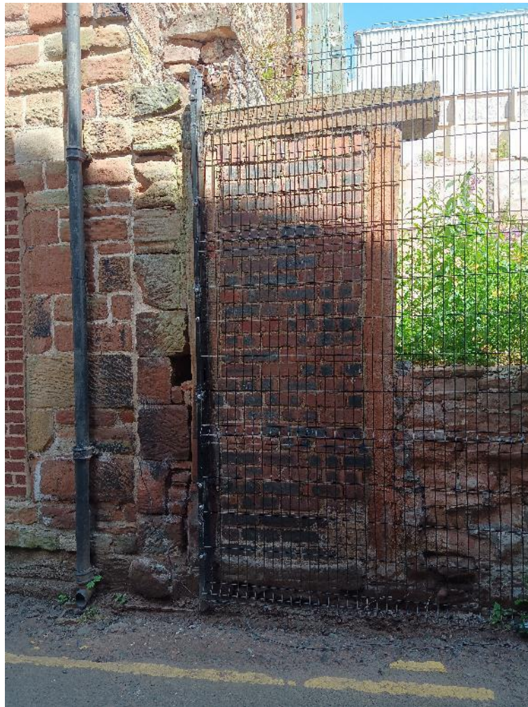
Plate 13: Blocked off doorway at west end of site
