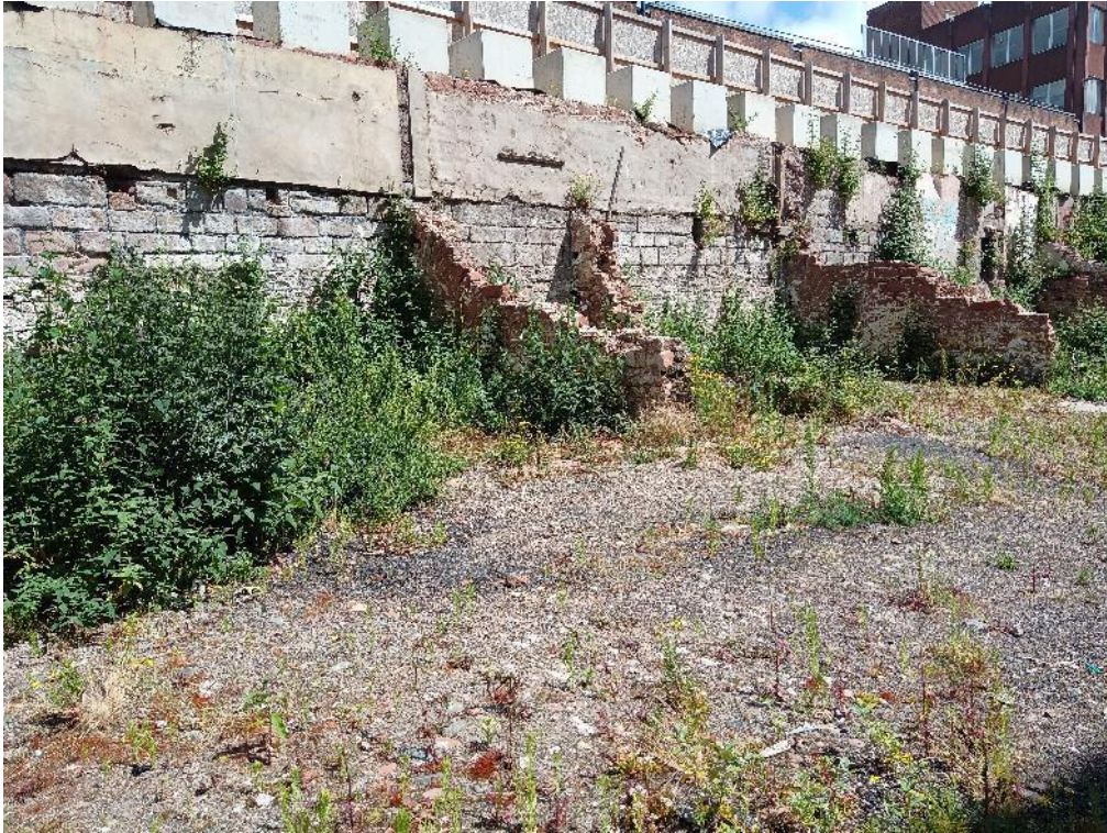
Plate 9: Remnants of stable partitions and west wall
