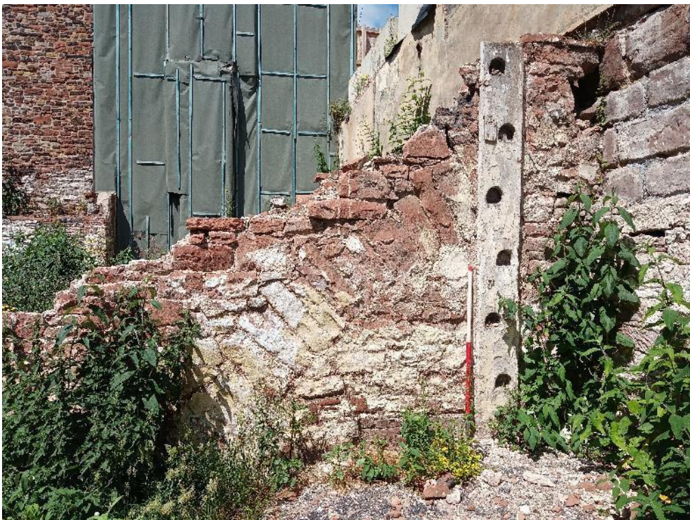
Plate 10: Ladder and arch support in former stable wall
