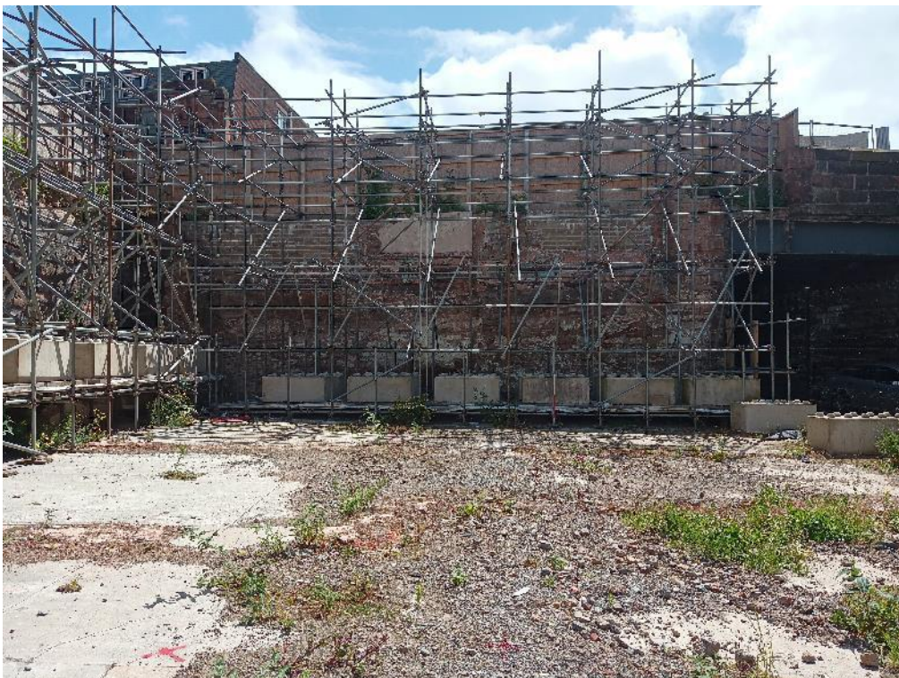
Plate 8: View of site towards Victoria Viaduct
