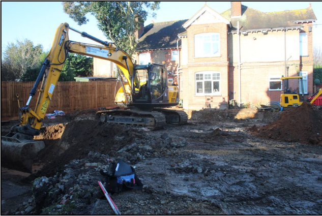
1 General site overview
