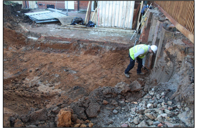
2 General site overview
