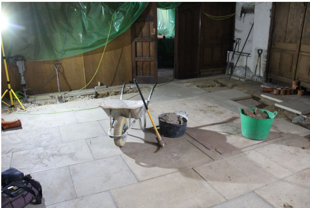
Plate 18: Working shot of the boxing pipework in the nave
