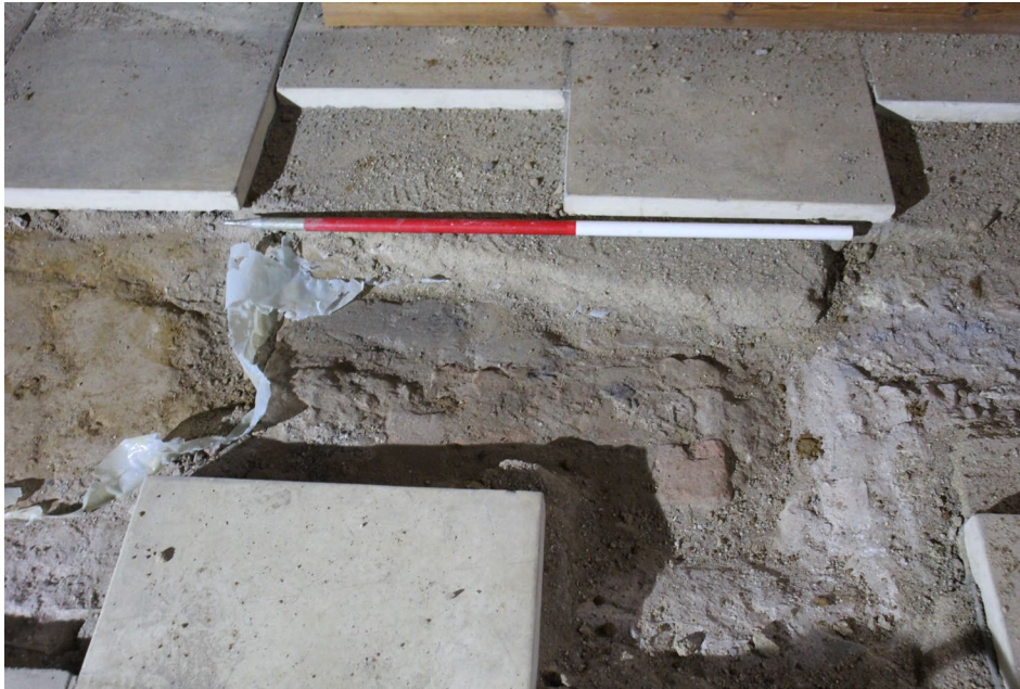
Plate 19: Monitoring of boxing pipework in nave
