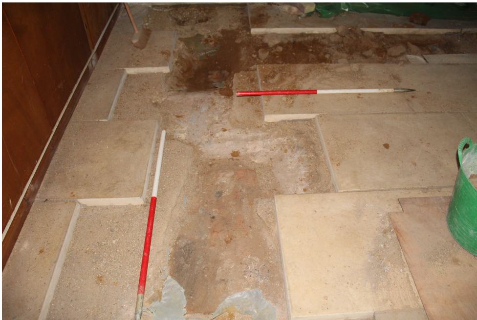
Plate 20: Monitoring of boxing pipework in nave
