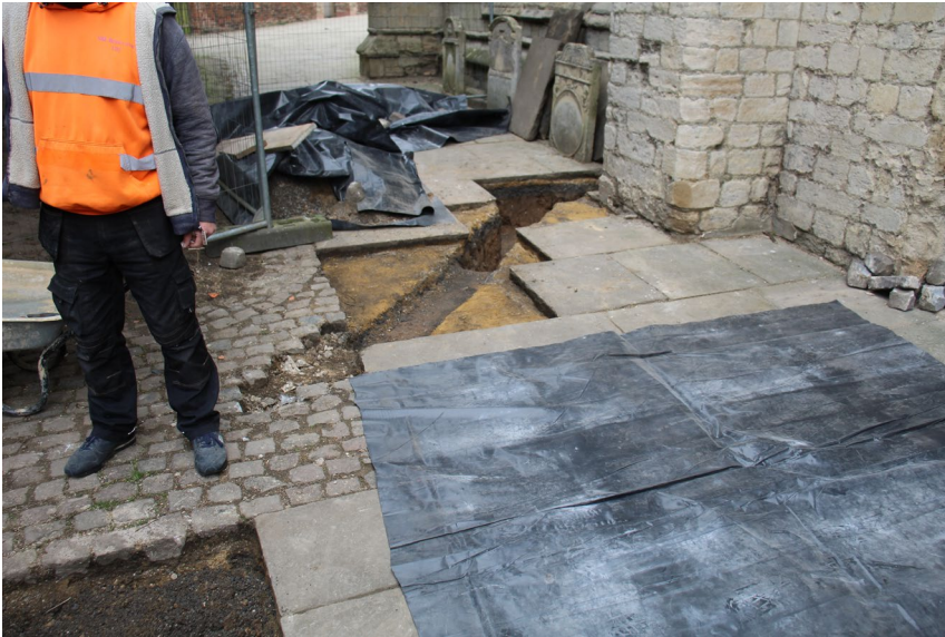
Plate 3: Northern trench with slabs removed north-east
