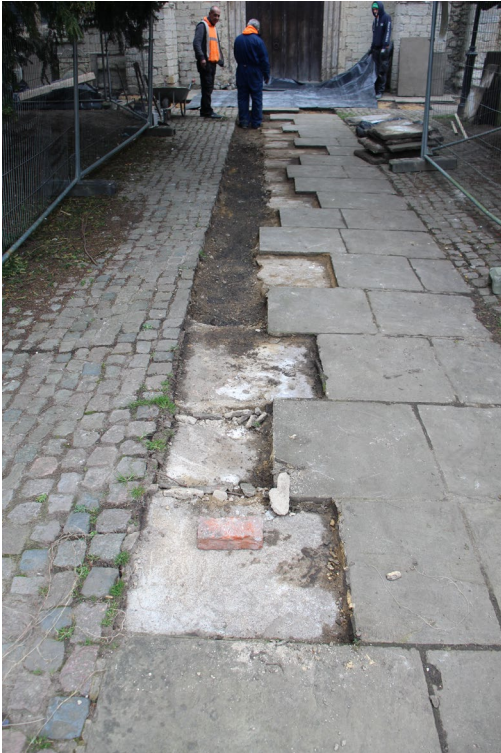
Plate 1: Western trench with slabs removed looking east
