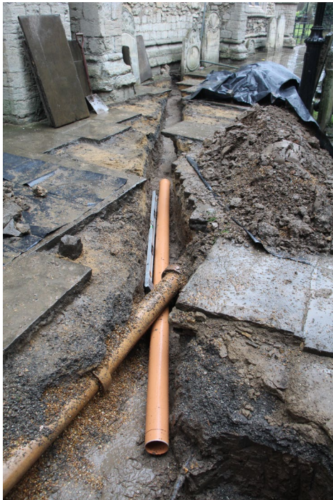
Plate 13: Southern trench post-excavation looking south-east
