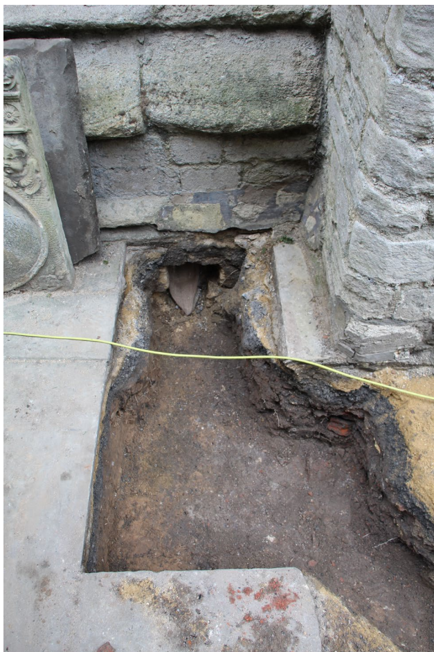
Plate 5: Northern trench post- excavation going under church
