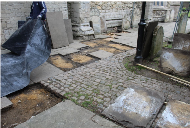
Plate 2: Southern trench with slabs removed looking south-east
