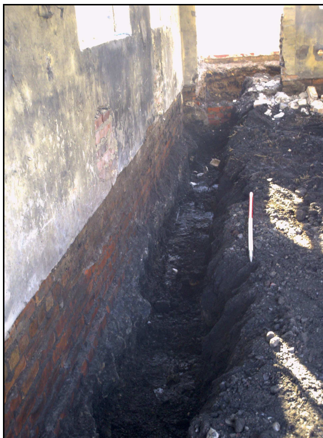
Plate 2: Trench Running NE-SW along interior foundation of SE wall
