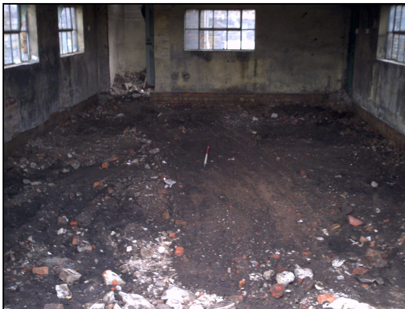
Plate 1: Interior of workshop after removal of concrete slab – SW Facing
