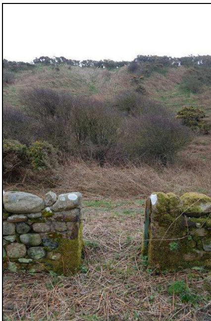
Plate 3: Example of one of the cottage gates, facing east
