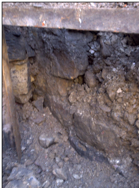
Plate 7: Shot of stone wall (013) in Area B beneath Lune Street from north west
