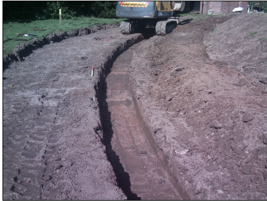
Plate 3: View northeast of trench within northern area of Area 2
