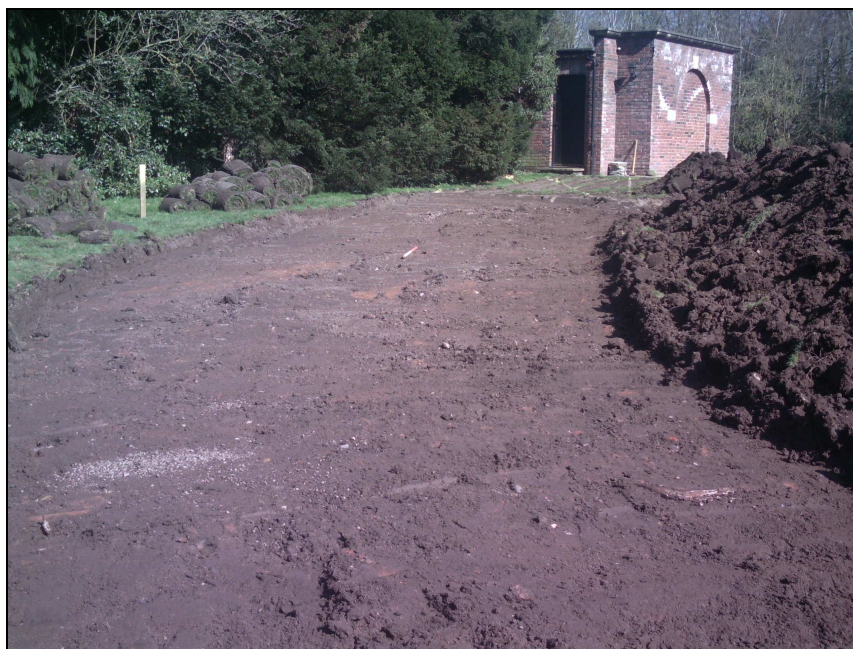
Plate 1: View northeast of northern end of Area 2
