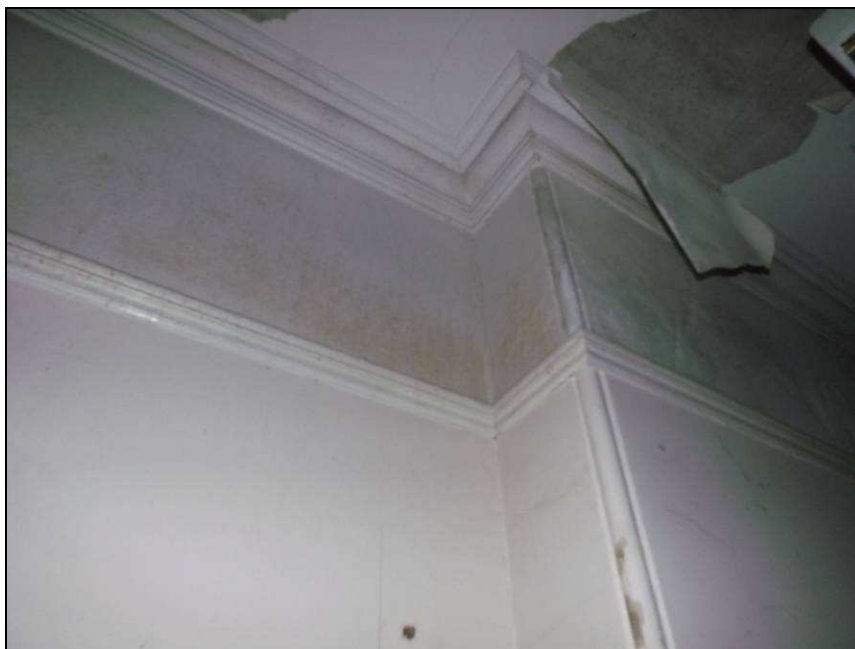
Plate 42: Detail of surviving coving and picture rail, first floor
