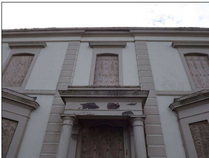
Plate 22: Detail of entablature of the portico and first floor windows
