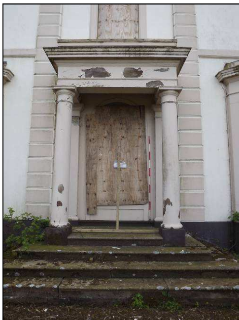
Plate 21: Detail of original main entrance set within a portico, north elevation
