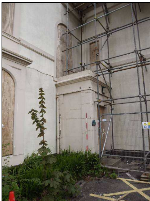
Plate 27: Detail of possible inserted porch, south elevation (Scale = 2m)
