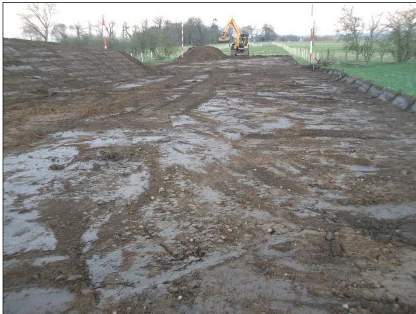
Plate 7: Area 10, topsoil stripping within the pipeline easement (facing east)
