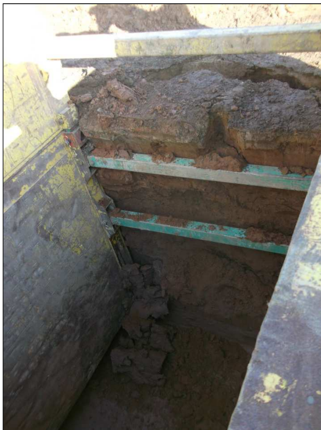
Plate 11: Area 3, horizontal bore shaft through natural substrate (101) on the eastern side of the Brunstock Beck (facing east)
