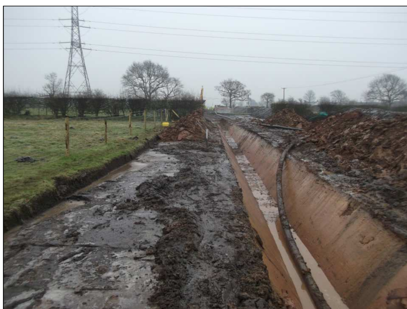
Plate 15: Area 7, Pipeline Trench Crossing Area 7 into Area 8 (facing east)
