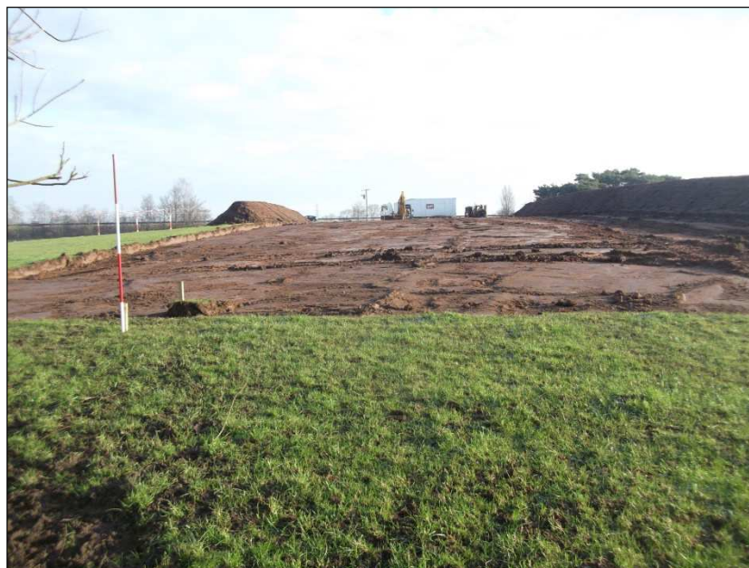
Plate 3: Area 3 topsoil stripped easement (facing east towards M6 Motorway)
