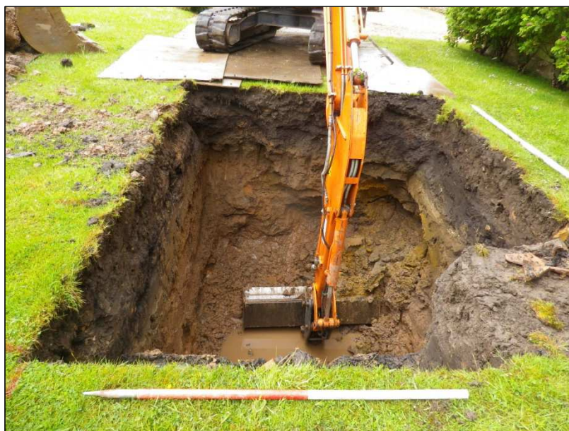
Plate 1: excavation of new septic tank pit (facing west)
