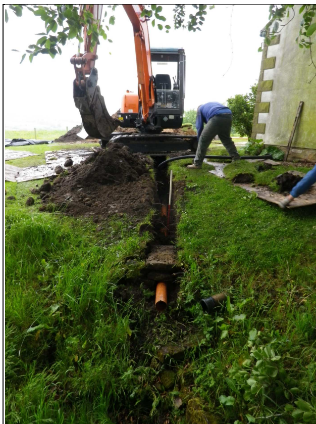
Plate 2: excavation of outflow trench (facing south-west)
