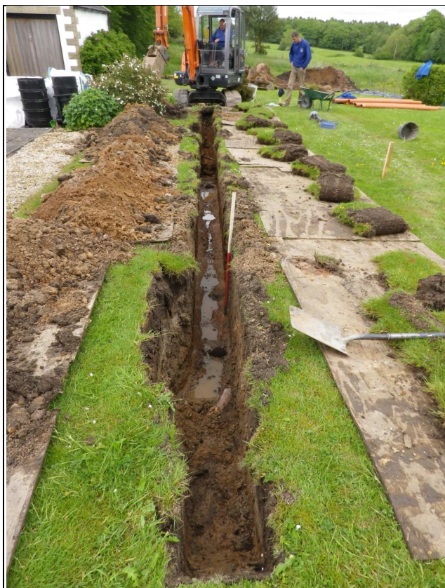
Plate 3: excavation of foul pipe connection trench (facing east)
