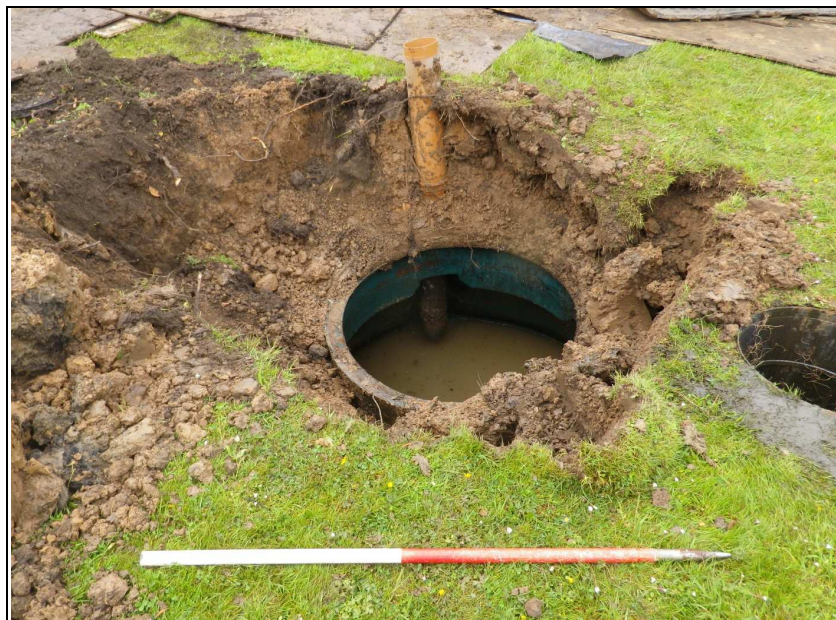
Plate 4: Excavation for removal of redundant septic tank (facing north)
