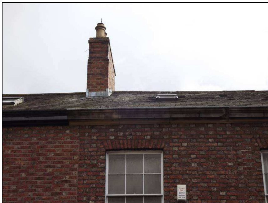
Plate 6: Detail of decorative stone cornice, west elevation
