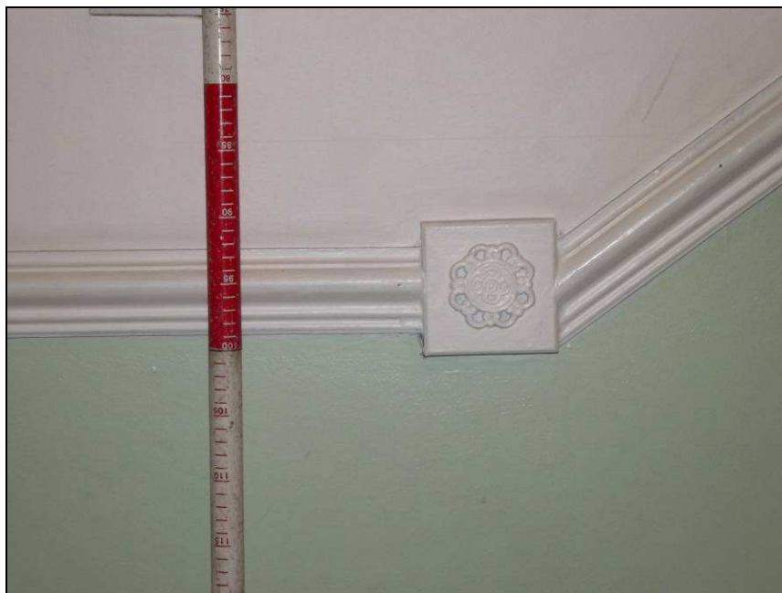
Plate 25: Detail of detailing on dado rail, ground floor hallway
