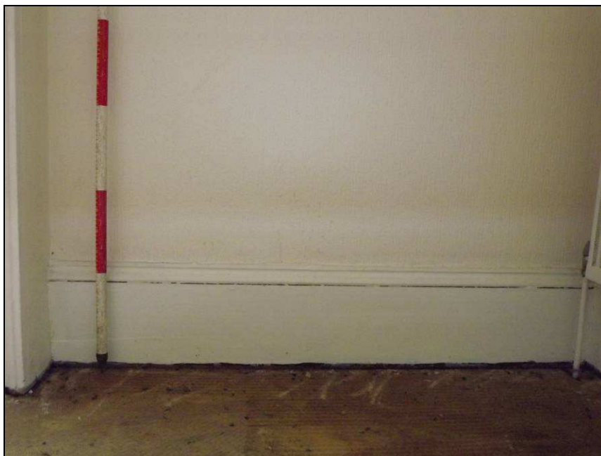
Plate 31: Detail of skirting board, Room G1, ground floor
