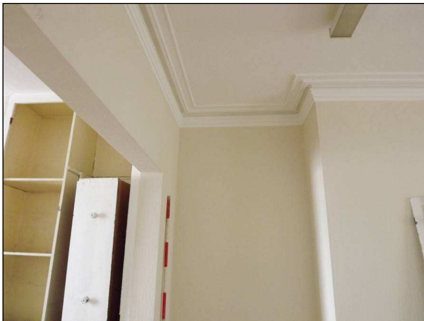
Plate 50: Detail of coving, Room F2 on first floor
