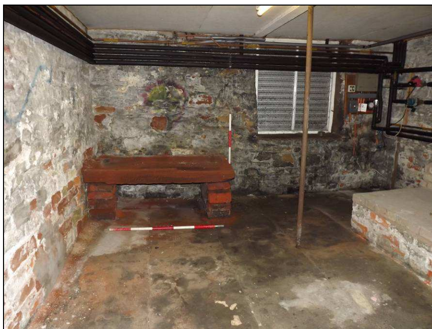
Plate 67: View looking east showing the sandstone 'trough' in Room B2 (Scales = 1m each)
