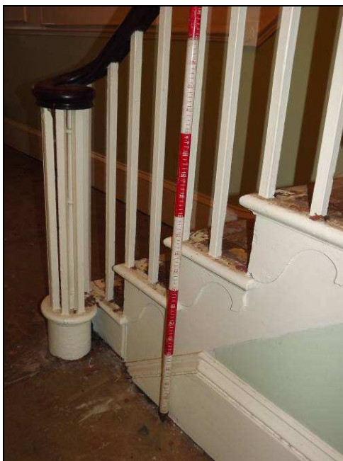
Plate 23: Detail of staircase balusters and open string detailing
