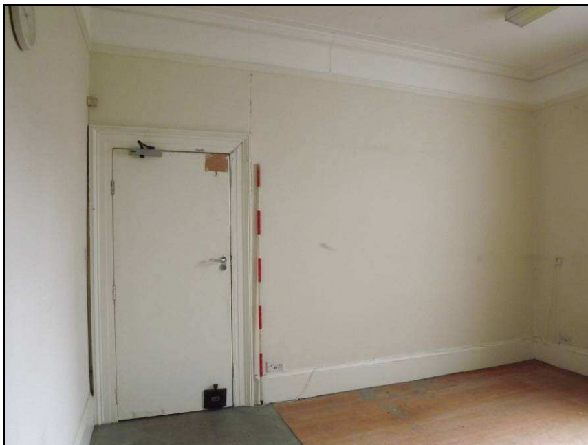
Plate 32: North wall of Room G2 (Scale = 2m)
