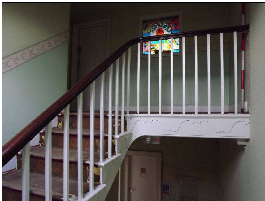
Plate 53: Detail of staircase and landing at second floor level
