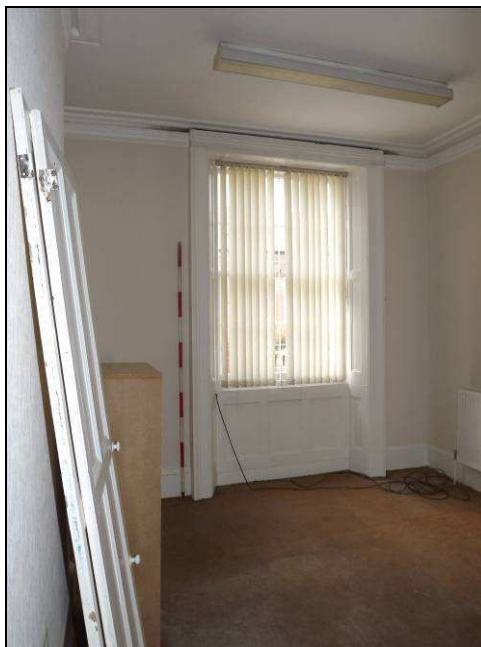
Plate 48: Detail of window, west wall of Room F2, first floor
