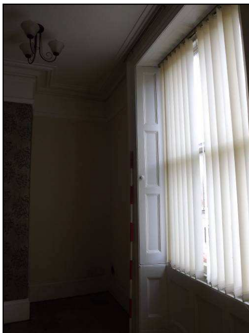
Plate 27: Detail of one of the shutters, window in Room G1
