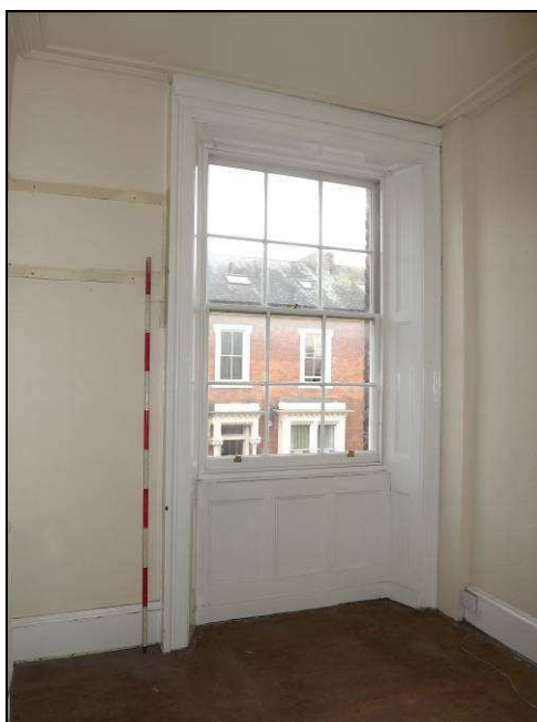
Plate 51: Window in the west wall of Room F3 (Scale = 2m)
