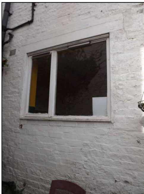
Plate 17: Detail of inserted kitchen window, south elevation
