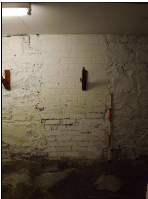
Plate 62: Detail of blocked doorway in north wall of basement (Scale = 1m)
