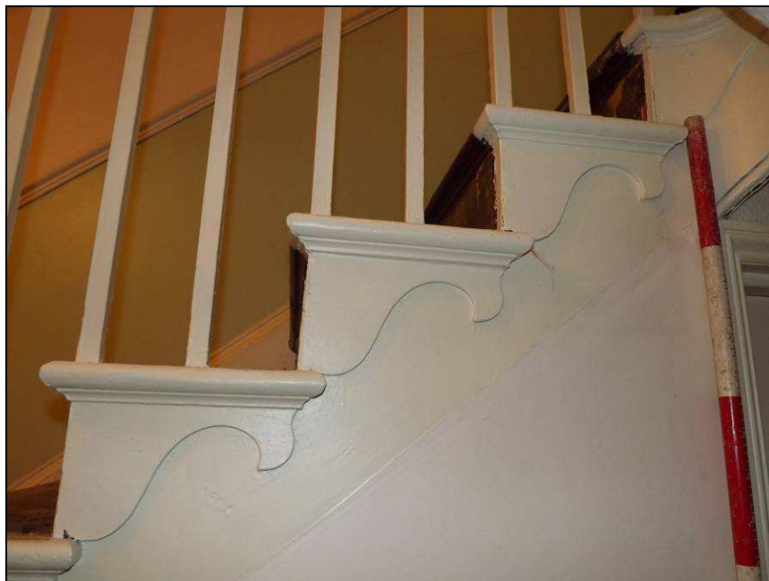
Plate 22: Detail of the side (open string) of the staircase
