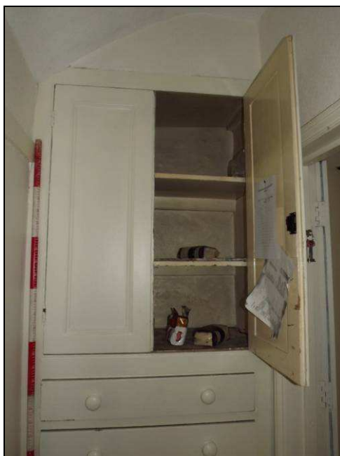
Plate 36: Detail of cupboard and shelving, ground floor
