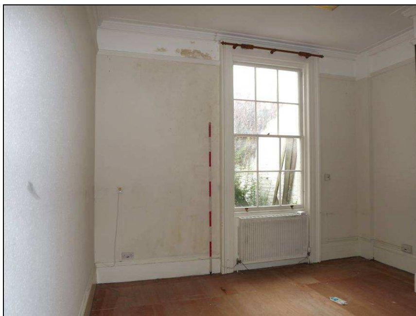
Plate 33: Window in east wall of Room G2, ground floor
