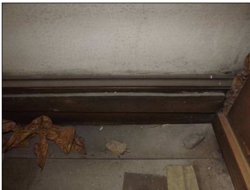
Plate 47: Detail of skirting, behind cupboard and drawers in Room F1
