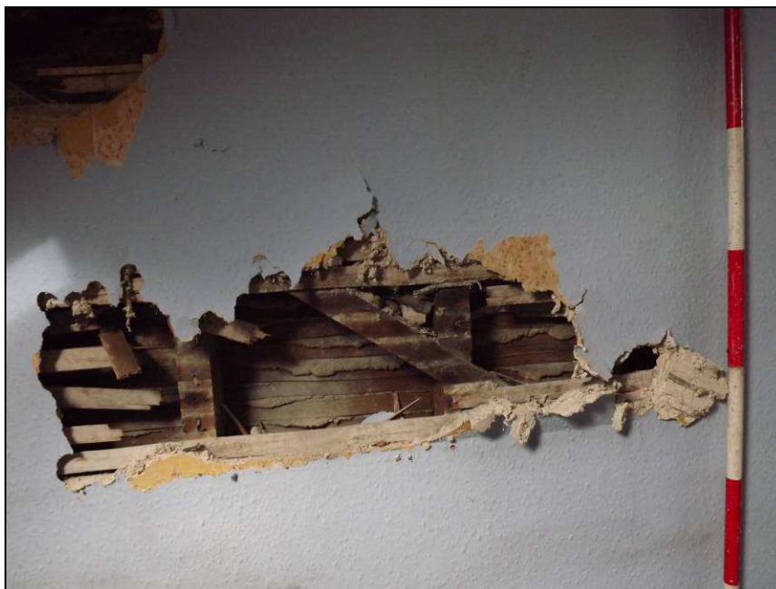
Plate 55: Detail of lathe and plaster wall, Room S1 in attic
