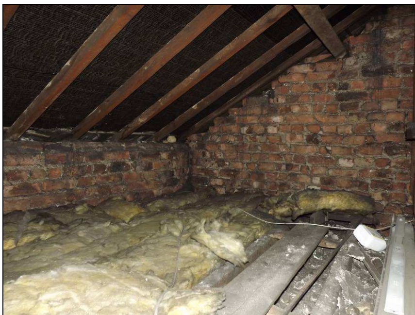
Plate 60: View looking north showing the party wall between No. 7 and No. 5
