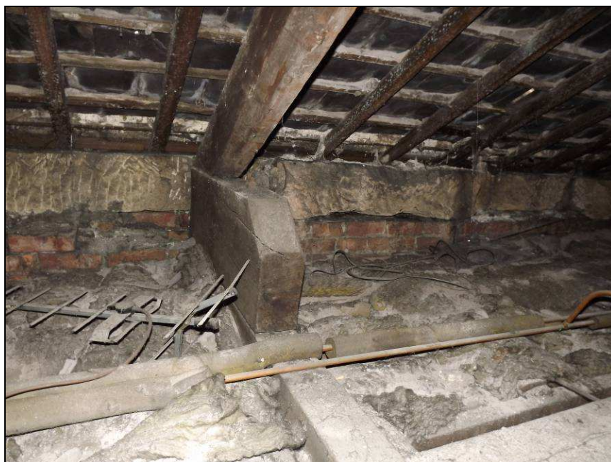
Plate 58: Detail of roof structure, west wall of building
