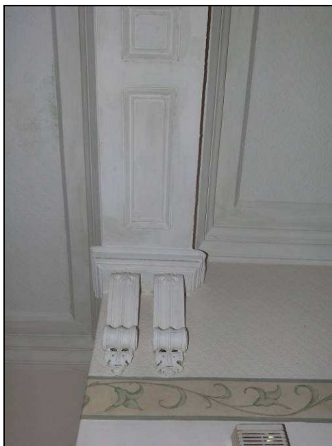
Plate 21: Detail of one of the console brackets and panelling, hallway
