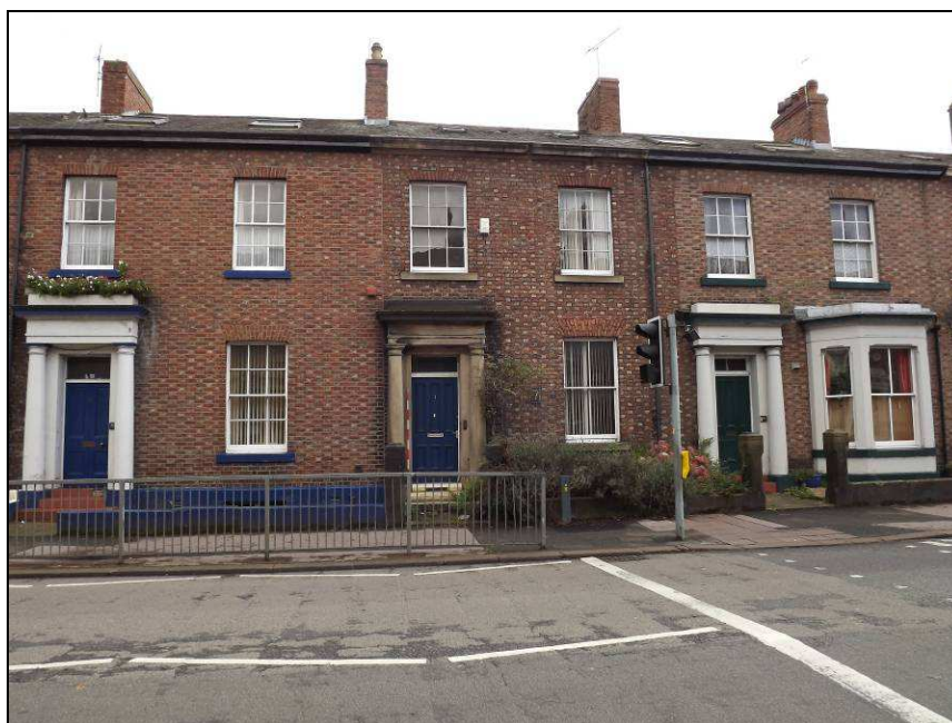
Plate 4: No. 7 Spencer Street, west elevation
