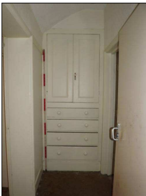
Plate 35: Detail of wooden cupboard and drawers, set between the staircase and Room G3 on the ground floor (Scale = 2m)
