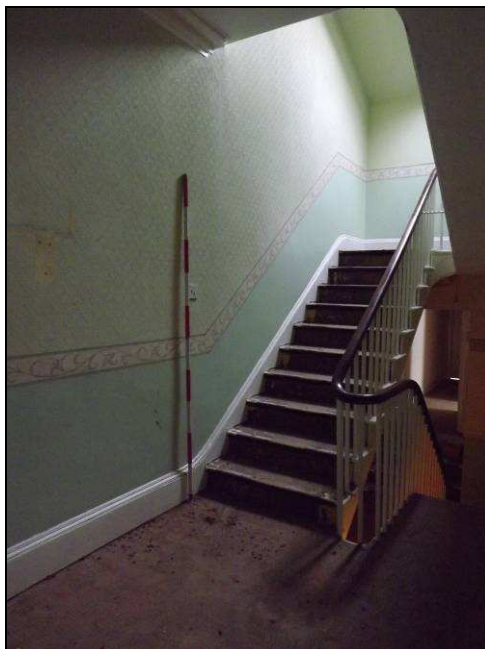
Plate 52: Staircase to second floor (attic) (Scale = 2m)
