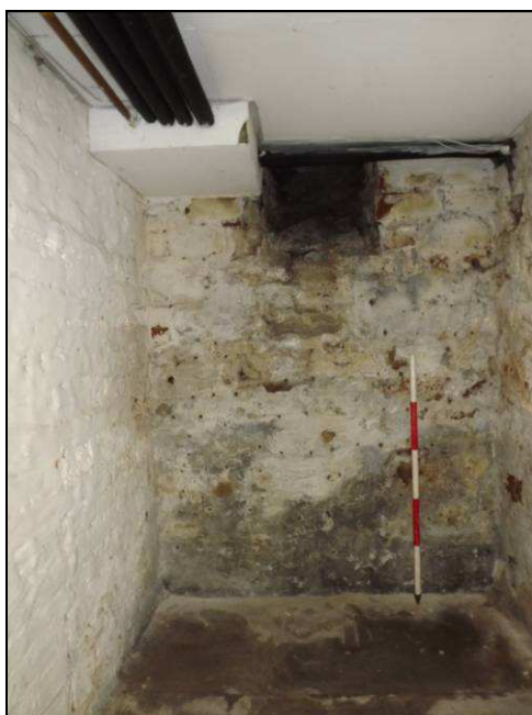
Plate 63: View looking west showing ventilation hole for basement (Scale = 1m)
