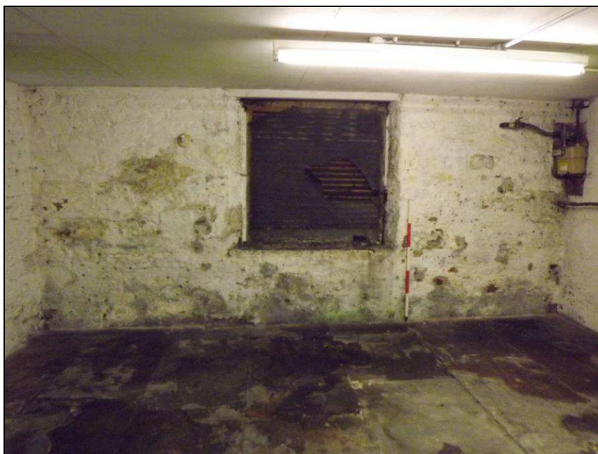
Plate 66: Detail of window in west wall of Room B1 (Scale = 1m)
