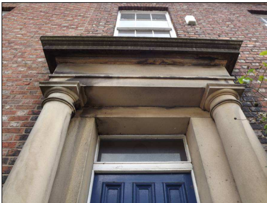
Plate 9: Detail of door surround, main elevation of 7 Spencer Street
