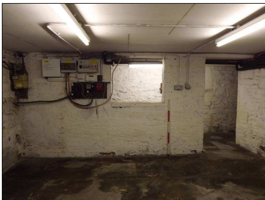
Plate 64: View looking north showing the north wall of Room B1 with square opening (Scale = 1m)
