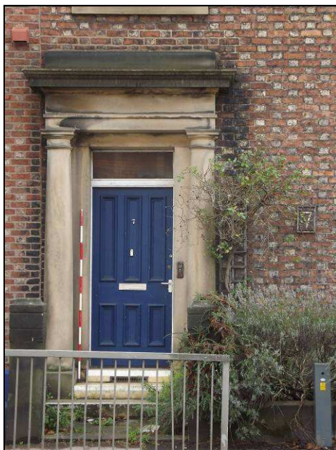
Plate 7: Detail of main entrance into 7 Spencer Street (Scale = 2m)
