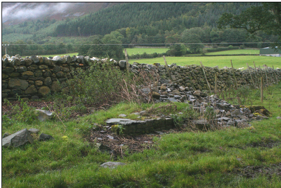
Plate 4: The ruins of a small building at the northern end of Field 3, facing northeast; the remains of the foundation can be seen, as well as the remains of a stone flagged roof
