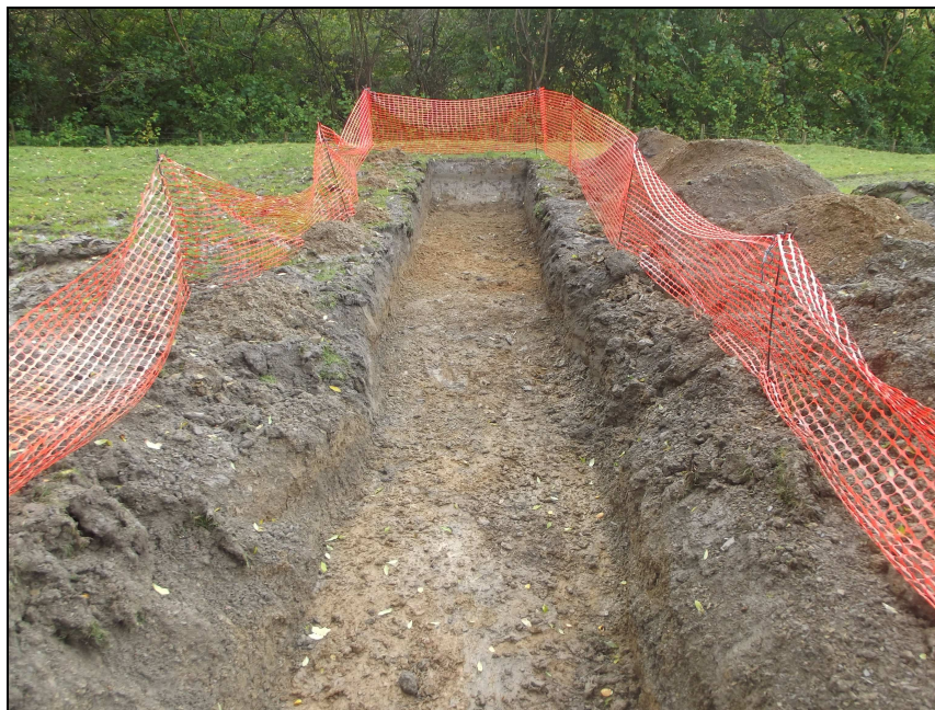
Plate 16: Trench 4, looking south west
