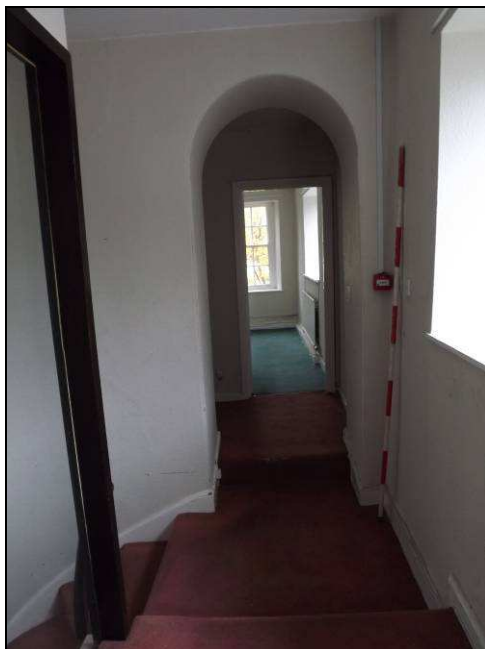
Plate 55: East end of first floor showing change in floor level for inserted staircase (Scale = 2m)
