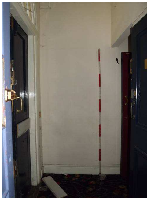
Plate 25: Possible blocked doorway, to west side of main entrance from Ladies' Walk
