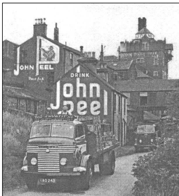
Plate 2: View looking west showing some of the brewery buildings in the 1950s. The gable end of the survey building is shown left of photograph with the John Peel, Pale Ale' paintwork
