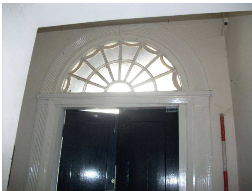
Plate 24: Detail of fanlight as seen from the interior, south elevation
