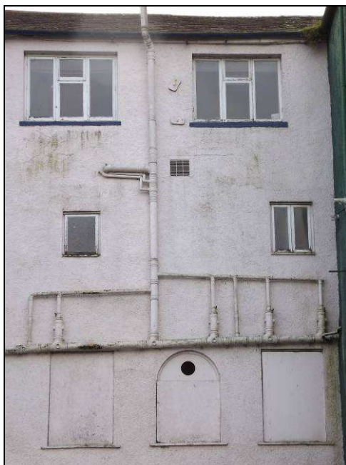
Plate 20: Detail of boarded windows and pipework for toilets above, north elevation
