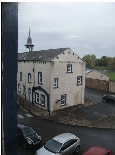
Plate 62: Former wine and spirit warehouse as seen from Ladies' Walk Level of the survey building (Room 4)
