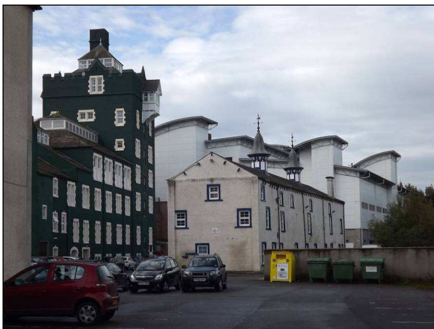
Plate 61: View looking west showing the stand alone remains of the wine and spirit warehouse with the green brewery buildings to left of photograph
