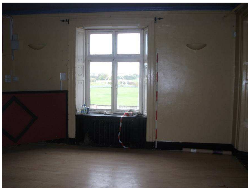
Plate 36: Window in north wall of Room 2
