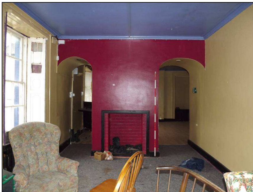
Plate 42: East wall of Room 3 showing inserted doorways and mock fireplace (Scale = 2m)
