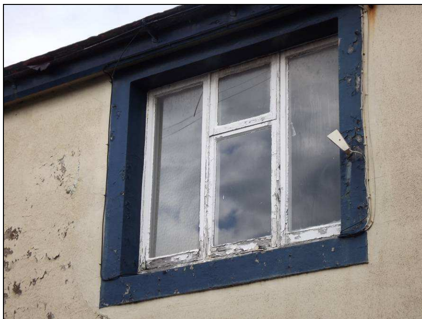
Plate 15: Detail of one of the inserted first floor windows, south elevation
