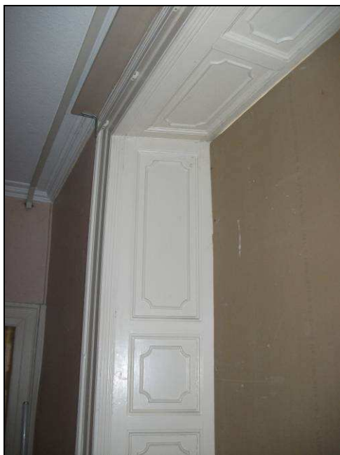
Plate 31: Detail of panelling of window surround, south elevation, Room 1
