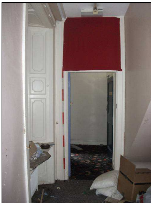
Plate 30: View looking west showing the panelling of the window in Room 1, with the inserted staircase to right of photograph
