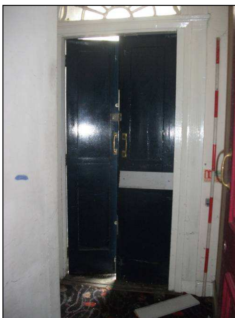
Plate 23: Detail of internal side of main entrance door in south elevation
