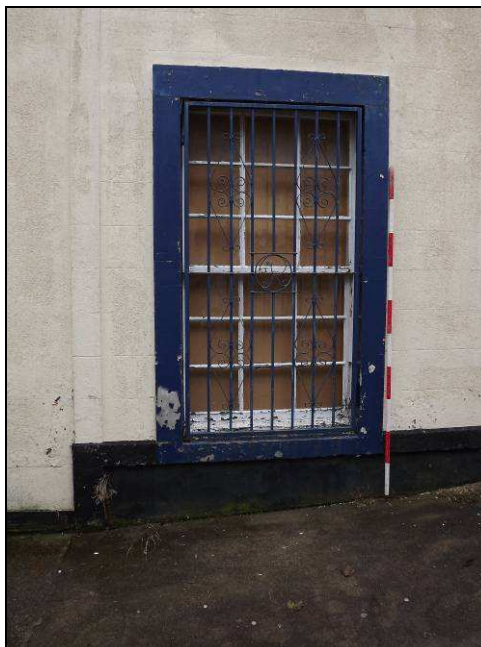
Plate 13: Western original ground floor windows, south elevation
