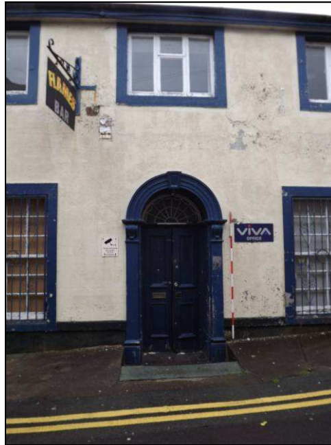
Plate 8: Original doorway in south elevation on Ladies' Walk (Scale = 2m)
