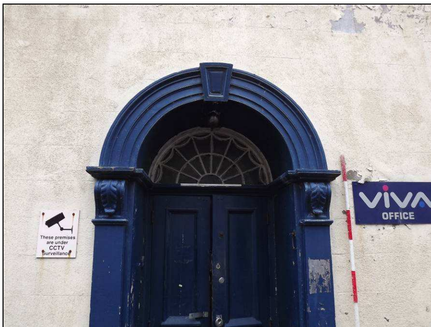
Plate 10: Detail of arched head of doorway in south elevation
