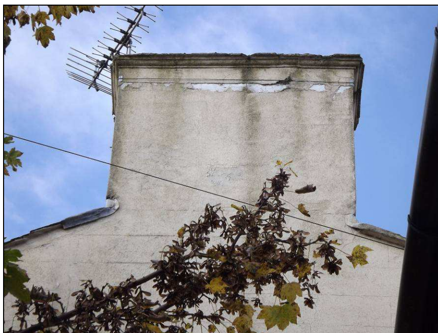
Plate 6: Detail of chimney stack at east end of building
