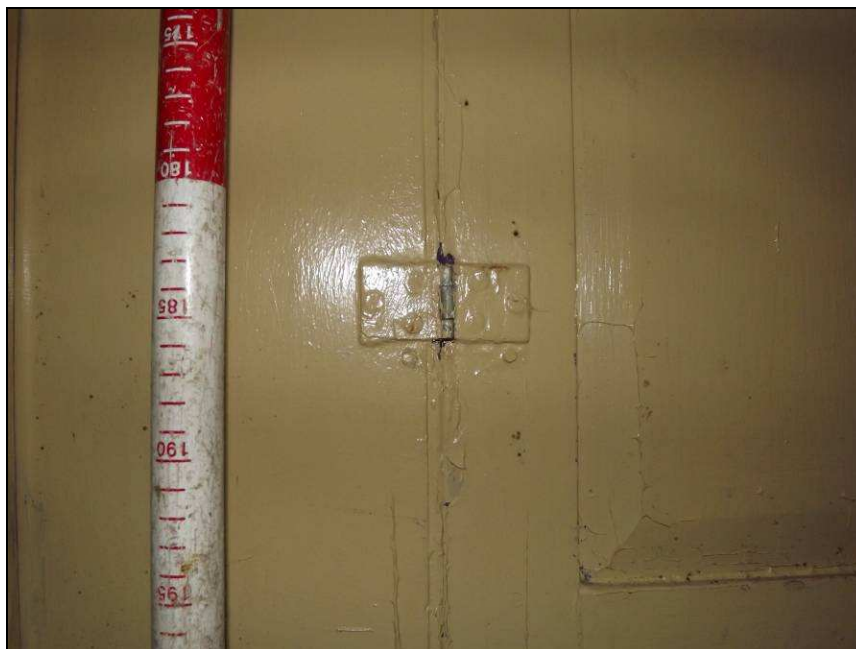
Plate 40: Detail of shutter hinge, window in north wall of Room 3
