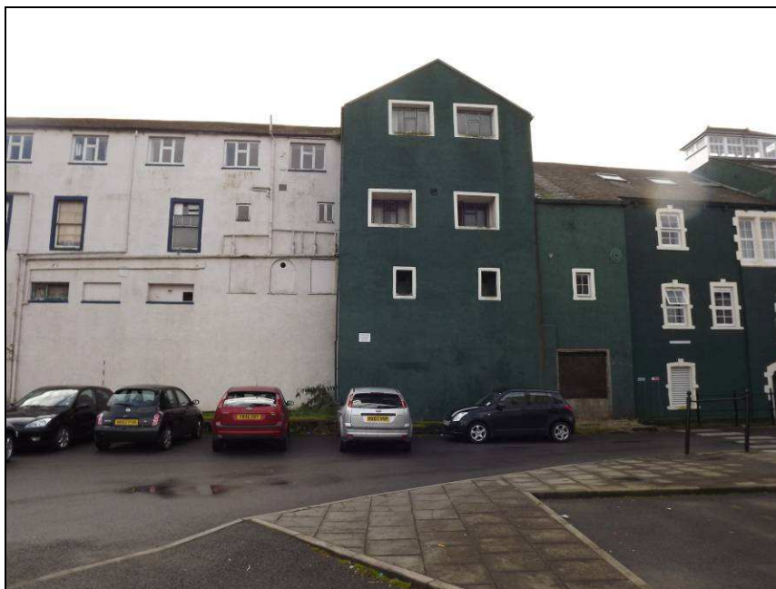
Plate 18: West end of survey building showing a projecting gabled section
