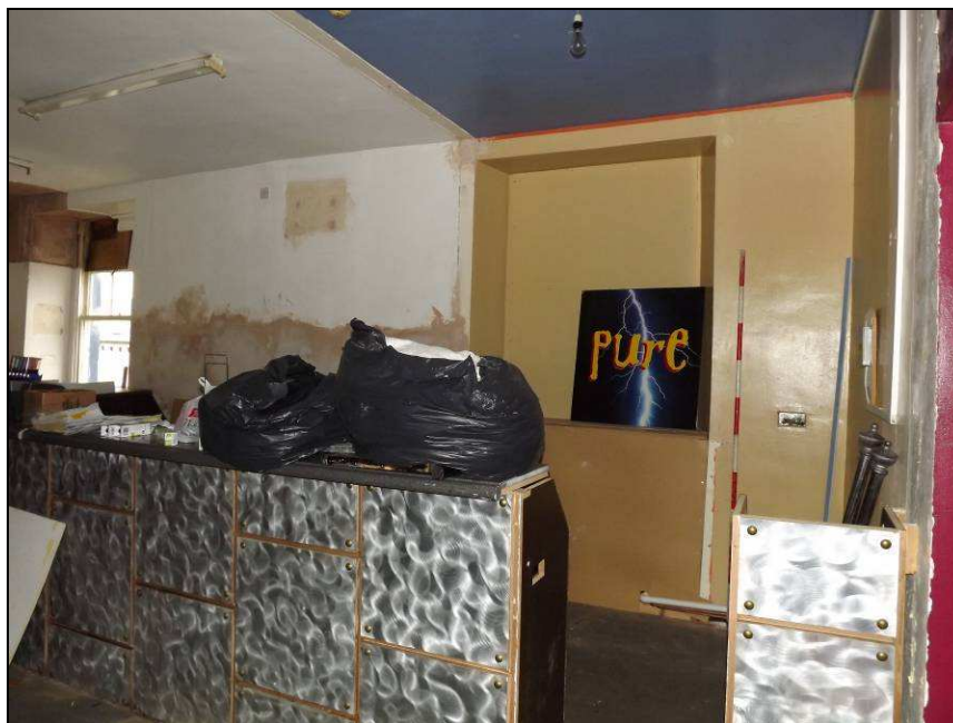
Plate 45: North wall of Room 4 showing location of boarded window
