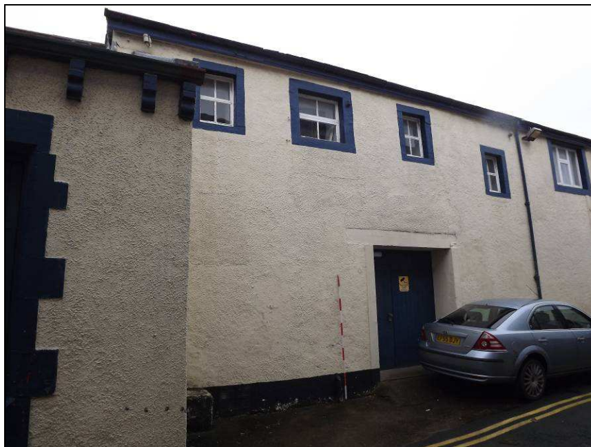
Plate 9: Possible inserted doorway, west end of south elevation (Scale = 2m)
