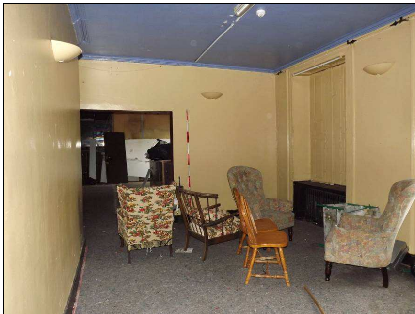
Plate 41: West wall of Room 3 showing large opening, the wall to the left is a later stud partition (Scale = 2m)
