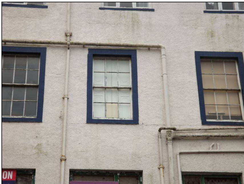
Plate 19: Detail of 'first floor' windows as seen in the north elevation
