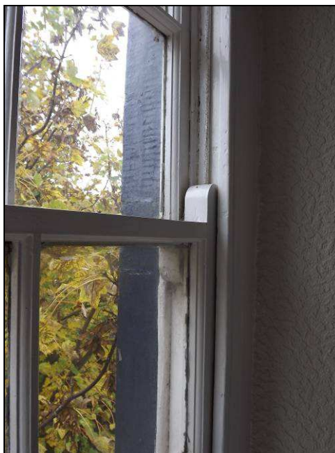
Plate 57: Detail of window horns, east gable, first floor level
