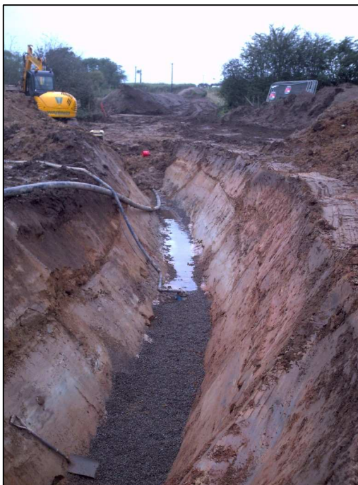
Plate 2: Wastewater pipe trench in Field 3 looking east
