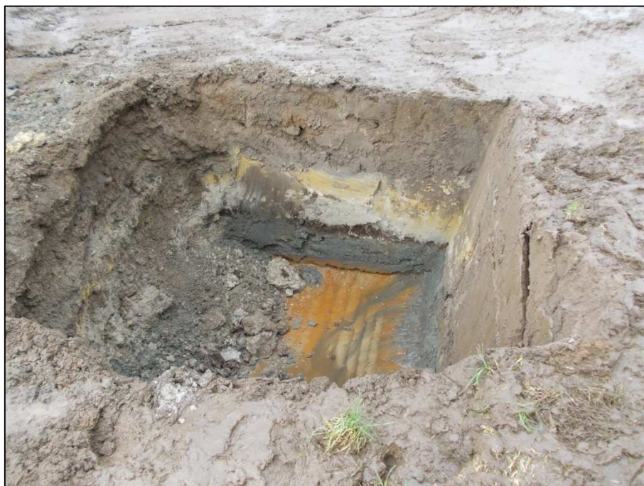
Plate 3: Pit for manhole at eastern extent of pipeline facing east
