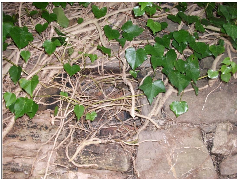
Plate 19: Close-up of blocked up window from riverbank in {506}
