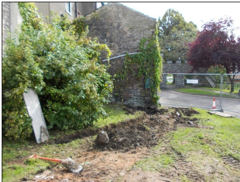
Plate 1: Location of Trench 1 looking south
