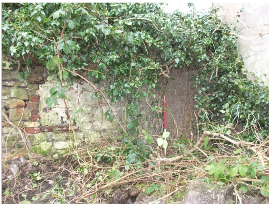
Plate 21: View from site of structure {506} with blocked door and window visible
