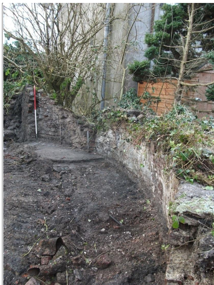
Plate 12: View looking southwest of extent of surviving windmill structure {501}
