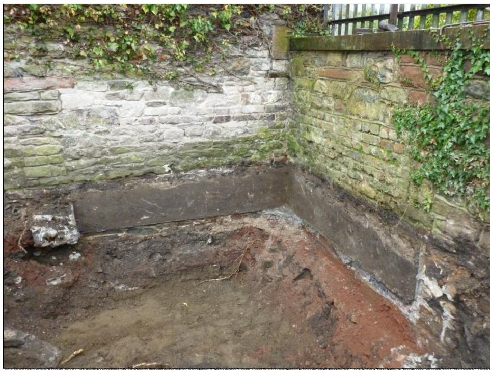
Plate 6: The Police Stable building showing the projection of walls {319} and {320} with concrete raft {321}
